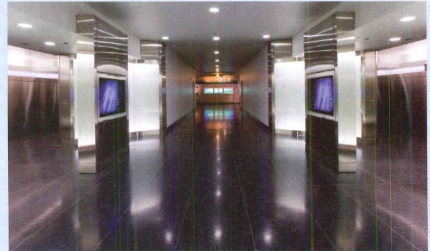
The Chicago Museum of Science and Industry used high-efficiency plumbing products and monitoring systems to realize significant water savings.
