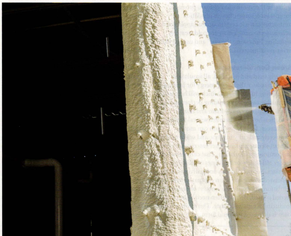
Spray foam insulation has been successfully installed to contribute to fire safety and to green building considerations.
