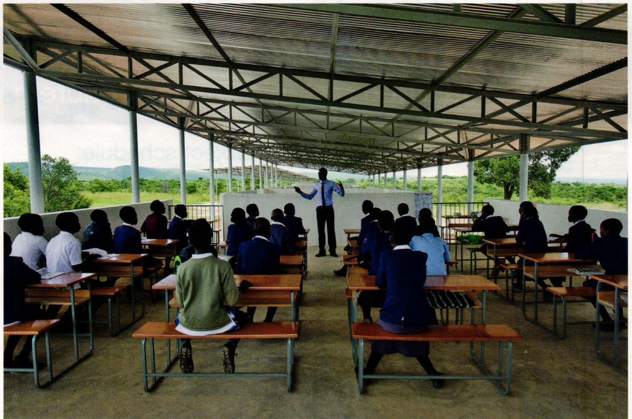
CLASS ACT Steel columns and trusses, along with the metal doors and windows, were purchased in the capital city of Lusaka and transported to the site over new roads built by the 14+ Foundation. The concrete (opposite) was mixed on-site using local labor. The arts-based curriculum is taught in daylight classrooms on two floors: at ground level (above) and an upper one (right) with a roof for shade and no walls.
