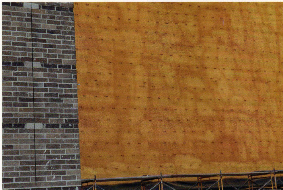
As a continuous air and water-resistive barrier, spray foam insulation seals completely around attachments such as these brick ties.
