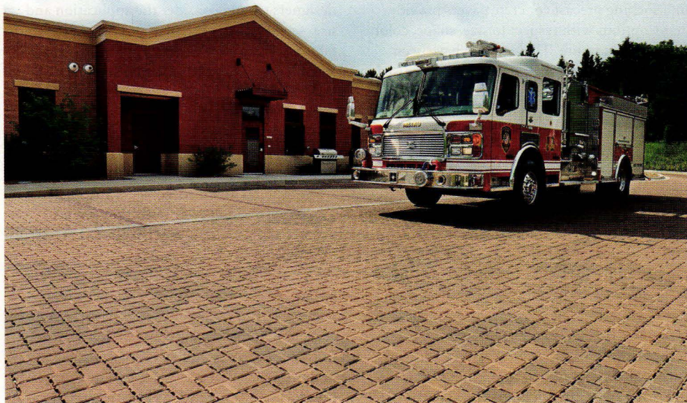
The Grand Traverse Fire Station, Grand Traverse, Michigan, designed by Gourdie-Fraser, Inc., shows color options for permeable interlocking concrete pavers.
