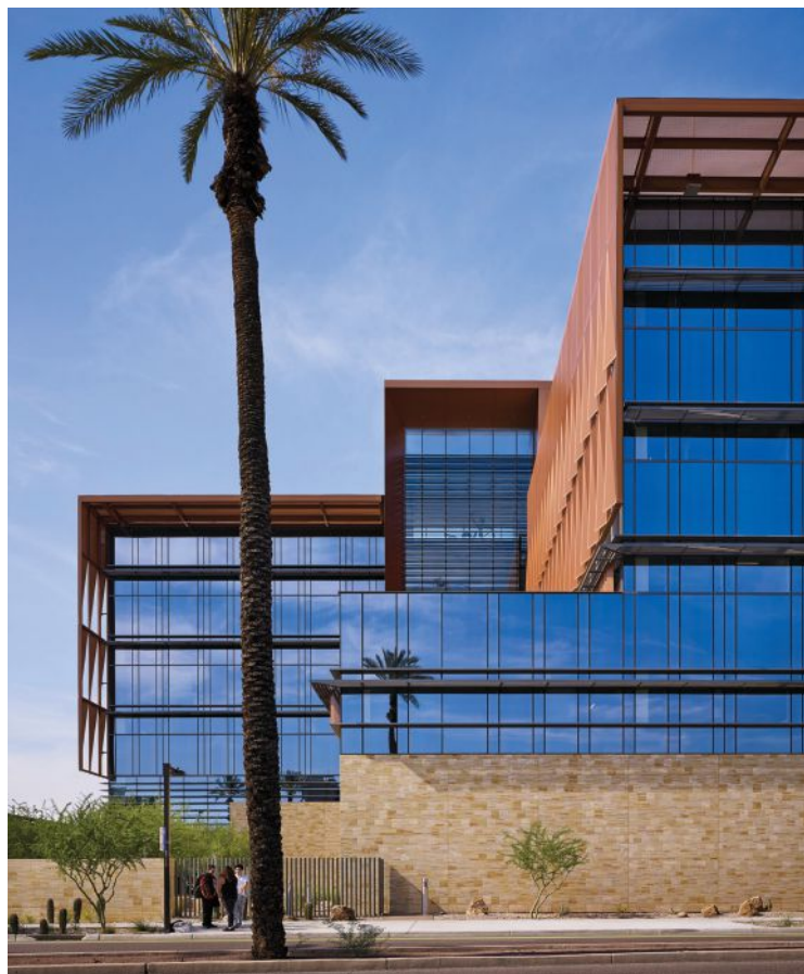
DESERT FLOWER The rhythmic placement of folded copper-colored screens on the east and west facades not only serves as a shading device but also creates a unique identity for the new building, which features large expanses of stone and glass as well.
