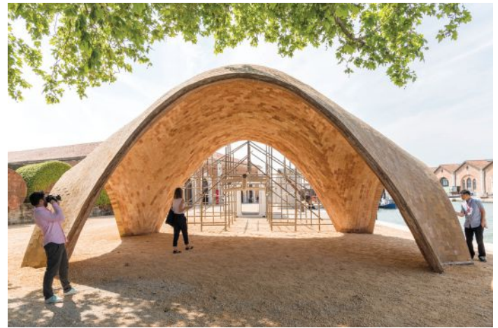
AT THE VENICE BIENNALE, THE NORMAN FOSTER FOUNDATION UNVEILED A PROTOTYPE OF A DRONEPORT, WHICH WOULD SUPPORT A NETWORK OF DRONE ROUTES FOR DELIVERING SUPPLIES IN DEVELOPING NATIONS.
