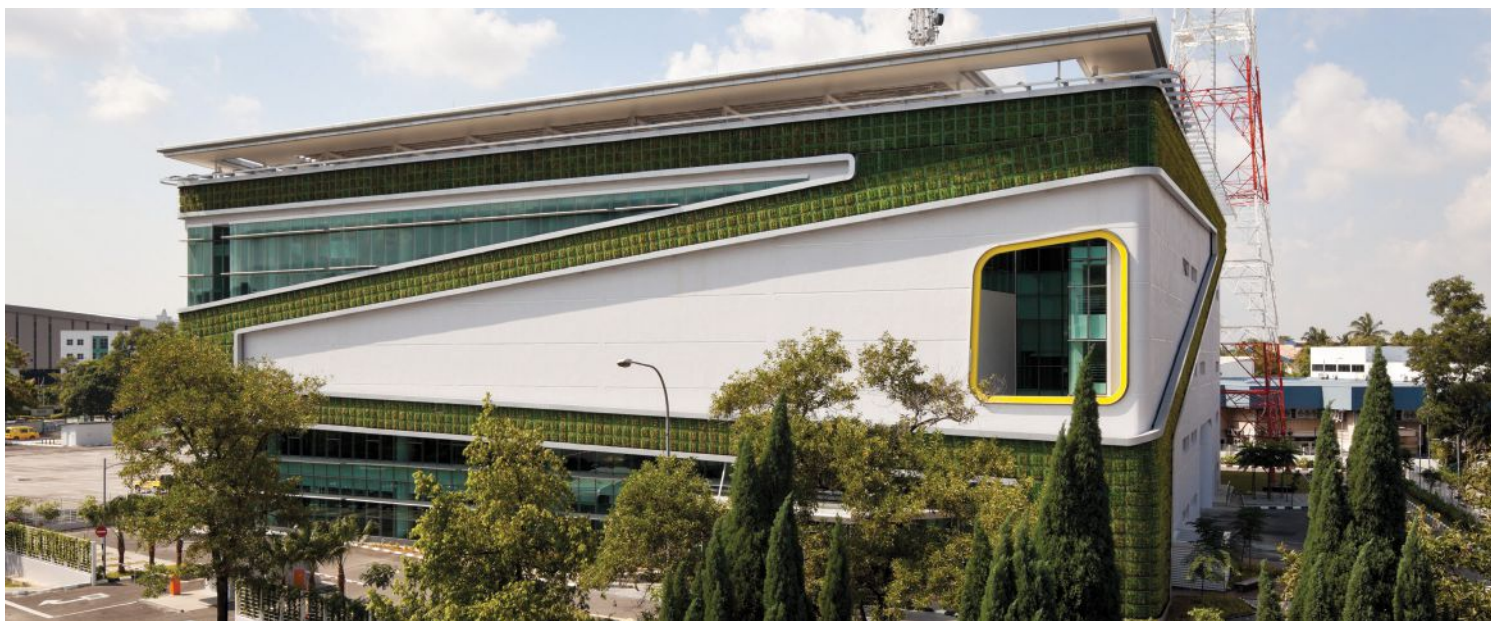
ENGINEERED ECOSYSTEM Plant selections and continuity of vegetation from the ground up maximize the diversity of birds, butterflies, and other fauna finding refuge and foraging at the DiGi data center in Malaysia.
