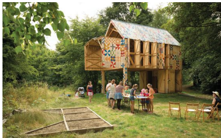
Je Ahn (left, top) and the team at Studio Weave recently completed Midden Studio, a zinc-clad artist's getaway in Scotland on the footings of a structure that once housed animal manure (top, right). In Kent, they built a zany outdoor classroom (above). RIBA South East named it Building of the Year in 2013. A pavilion for Clerkenwell Design week makes ingenious use of fiber-cement (bottom).
