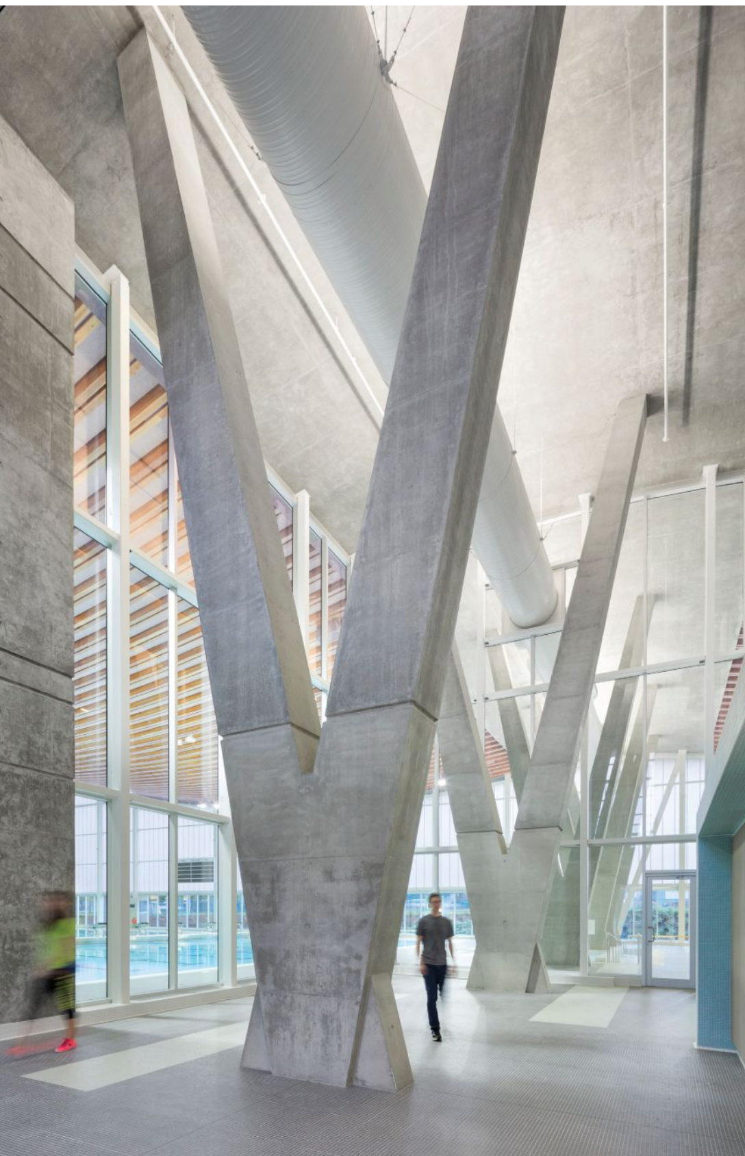
GRANDVIEW HEIGHTS The ceiling's roller-coaster-like contours are made up of pairs of exceedingly slender curved glue laminated beams (opposite). They are supported at each end of the building by concrete buttresses and at midspan by V-shaped concrete columns that help articulate the entrance area (above).
