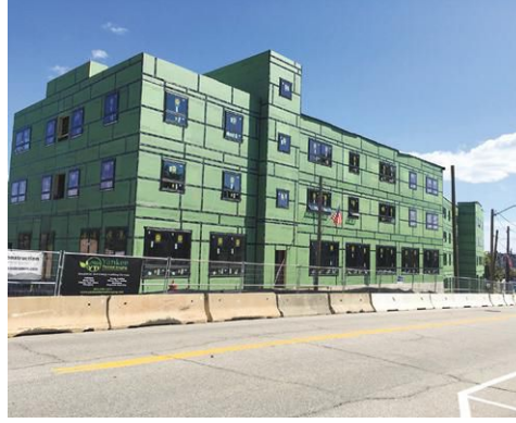
Integrated sheathing and tape systems are popular in multifamily construction because of their high performance and jobsite labor savings.
