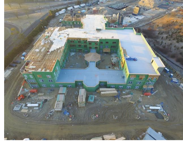
Integrated sheathing and tape systems are popular in multifamily construction because of their high performance and jobsite labor savings.
