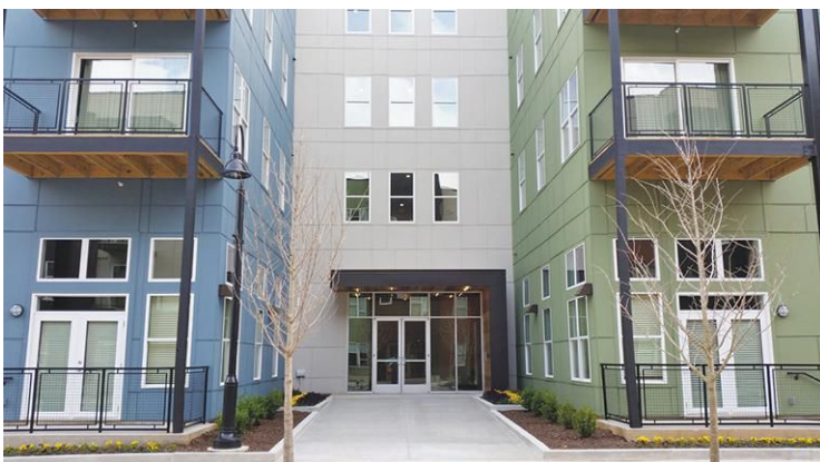
Exterior cladding panels can be held in place along their edges using extruded aluminum trim that also contributes directly to a more contemporary and market appealing facade design, such as at the Artisan in Huntsville, Alabama, shown here.
