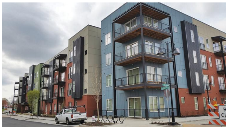
Exterior cladding panels can be held in place along their edges using extruded aluminum trim that also contributes directly to a more contemporary and market appealing facade design, such as at the Artisan in Huntsville, Alabama, shown here.
