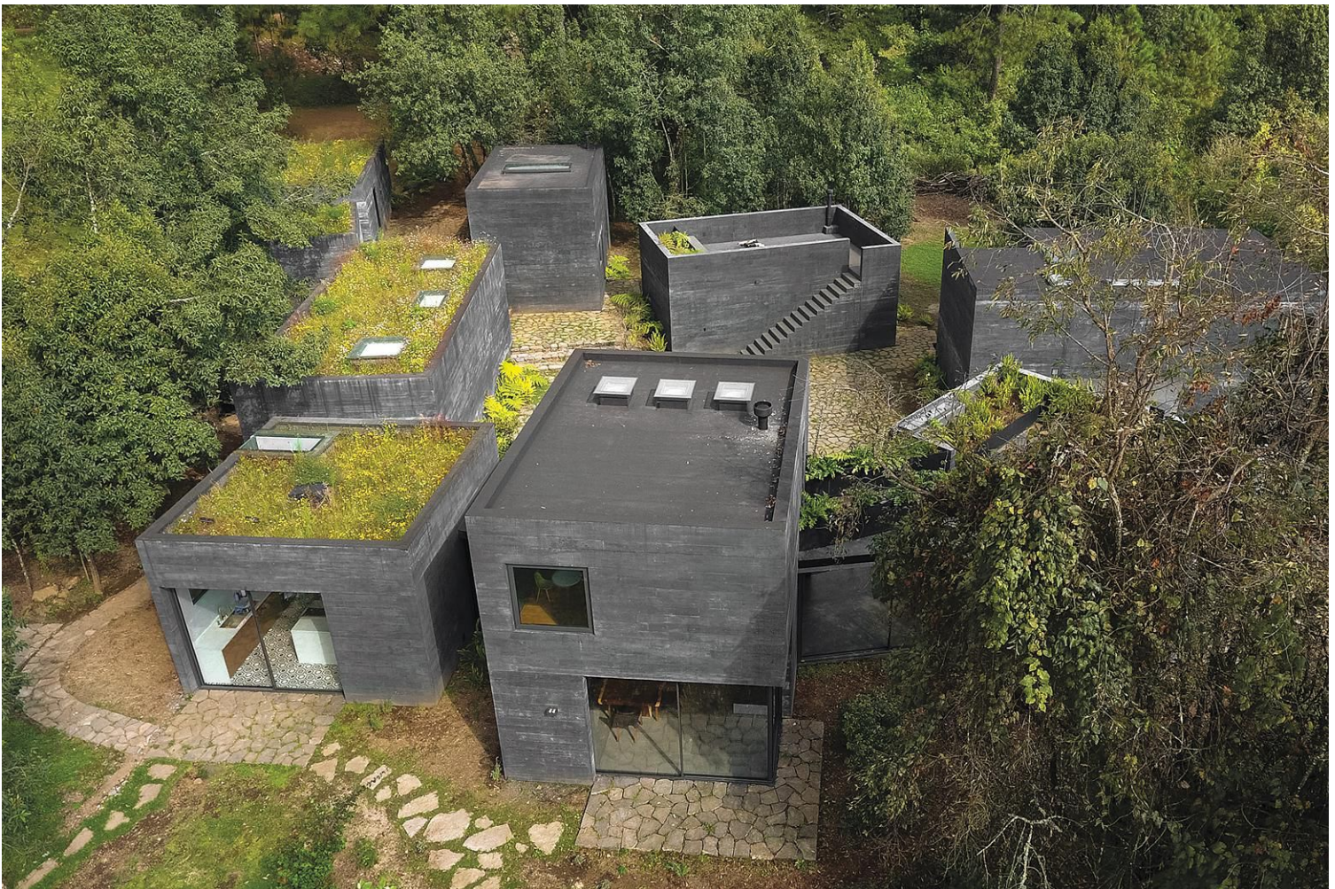
BOXED SET Casa Bruma comprises nine volumes (above) of poured-in-place concrete, set at angles in its partially wooded site to create an irregularly shaped courtyard (opposite). The pavers here conceal a below-grade cistern for collecting and storing rainwater, the house's only water source.
