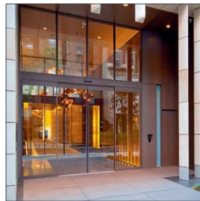
Automatic Sliding Doors
