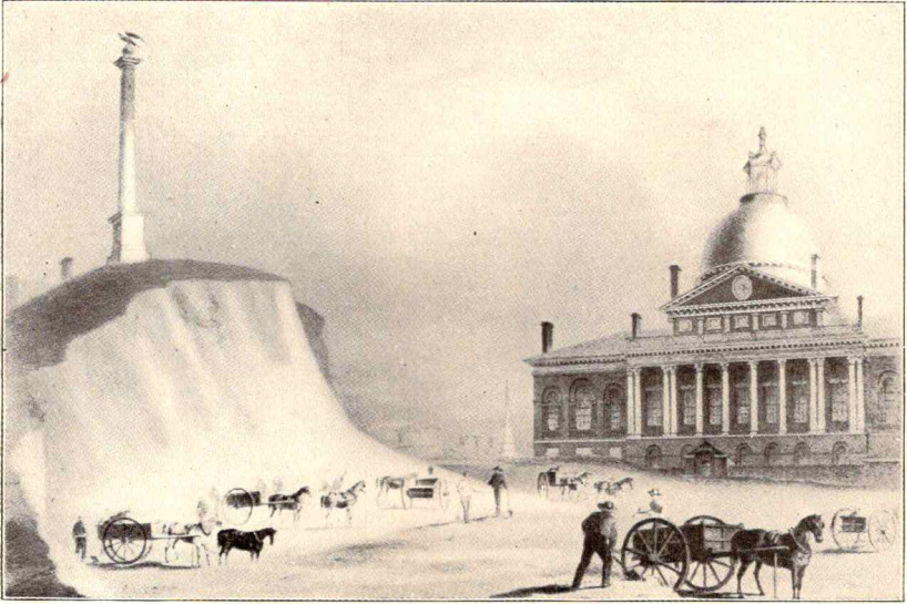
BEACON HILL DURING EXCAVATION
