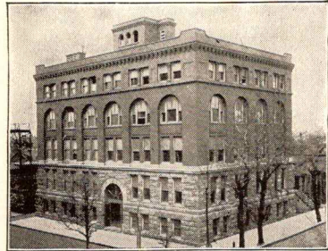
MACHINERY HALL, ARMOUR INSTITUTE OF TECHNOLOGY.
