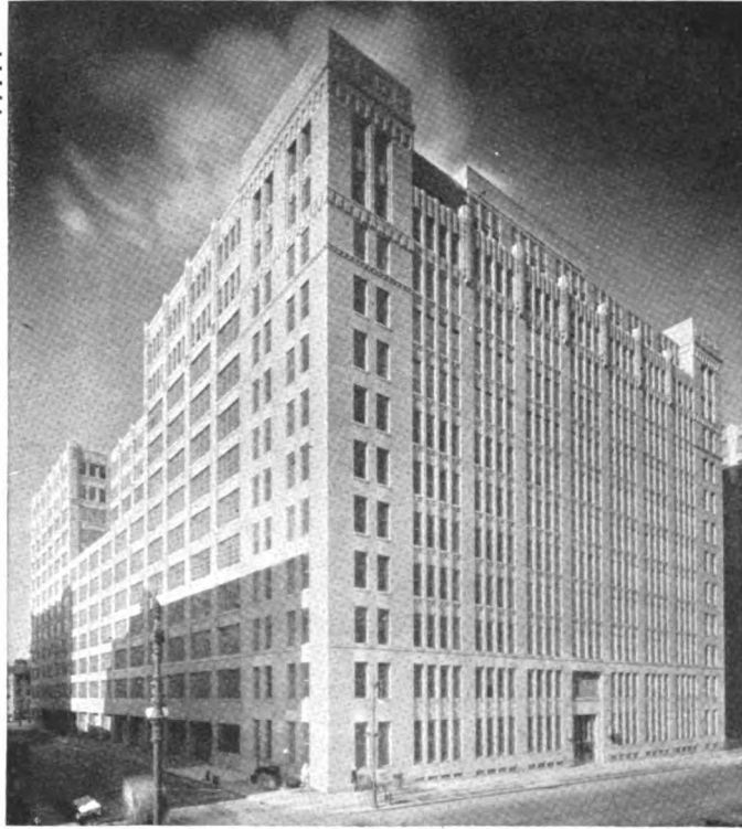
U. S. Appraisers Stores and Customs Court Building, New York City. Buchman and Kahn, Architects; Alex. D. Crosett, Engineer; Shroder and Koppel, General Contractors; Turner Construction, sub-contractors for concrete and masonry. Twelve stories and basement, area 200 by 400 feet. Structural concrete frame; steel column cores; flat slab and beam-and-girder floors.
