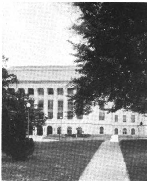
View of the Agricultural Build- ing from the Mall
