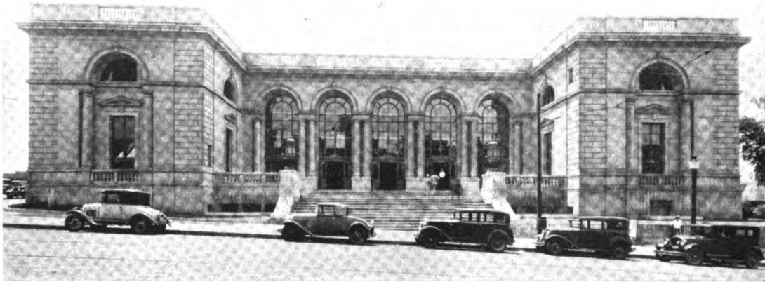
U. S. Post Office, Akron, Ohio Exterior of Limestone furnished by Bloomington Limestone Company
