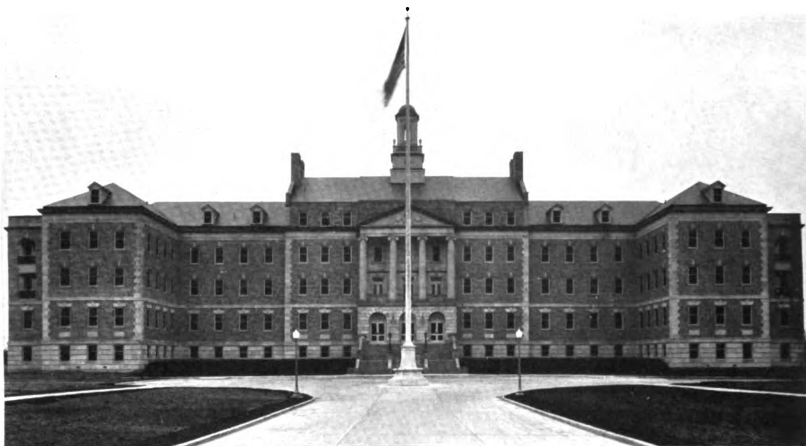
FACADE OF MAIN BUILDING UNITED STATES VETERANS' HOSPITAL, INDIANAPOLIS, INDIANA Construction Div., Veterans' Administration, Architects Ralph Sollitt & Son, Contractor
