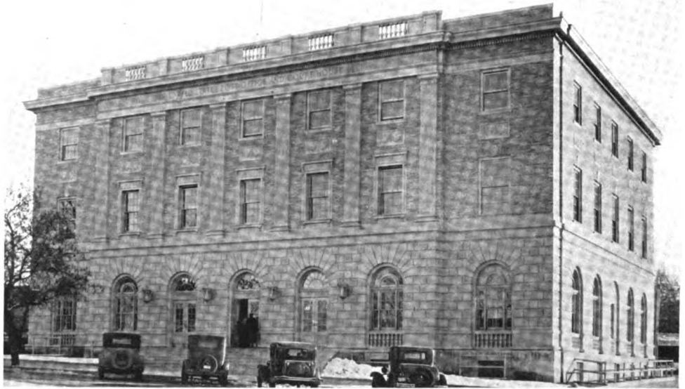
The new United States Post Of- fice at Prescott, Arizona. Office of the Supervising Architect, Architects, Robert E. McKee, Builder.
