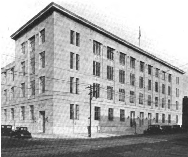
U. S. Post Office, Camden, N. J. Office of Supervising Architect, Architects Agostini Bros., Builders
