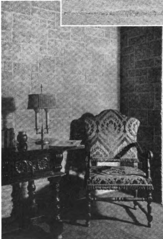
An office interior of concrete masonry, the surface decorated with a base coat of reddish brown and a top coat of light buff portland cement paint.
