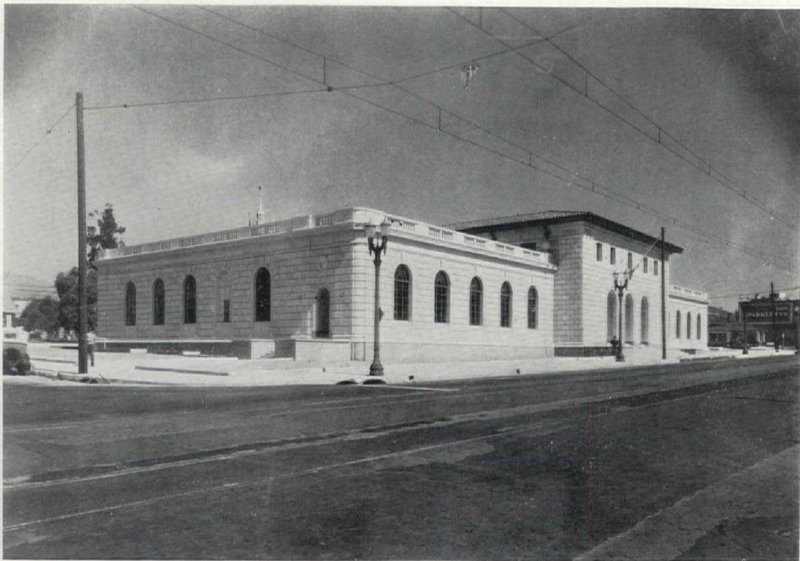
POST OFFICE, GLENDALE, CALIFORNIA
