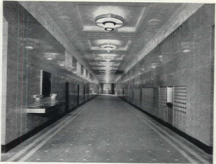
Virginia Black Serpentine base and door trim, U. S. Post Office & Court House, Hartford, Conn., Malmfeldt, Adams & Prentice, Architects.
