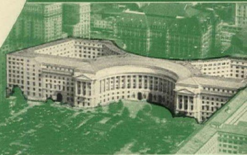
3. POST OFFICE DEPARTMENT BUILDING
