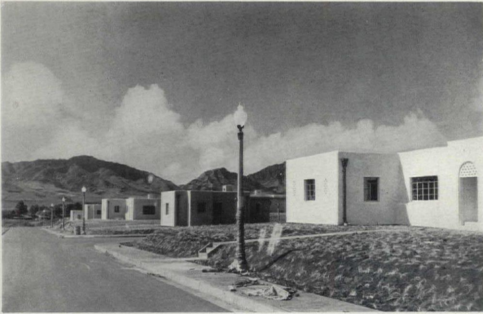
Flat roofs and stuccoed walls in Hawaii. A group of houses for Non-commissioned Officers at Wheeler Field.
