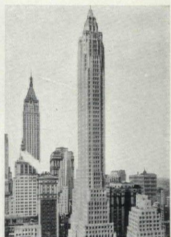
Cities Service Building, New York
