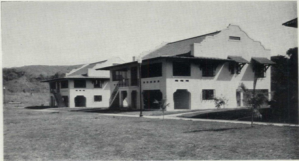
(Below) Field Officers' Quarters at Fort Clayton, Canal Zone. One-story buildings of typical "Zone" construction. The first floors are raised quite high above the ground as a protection against insects. The windows are protected by overhangs against rain, the windows being open at all times.
