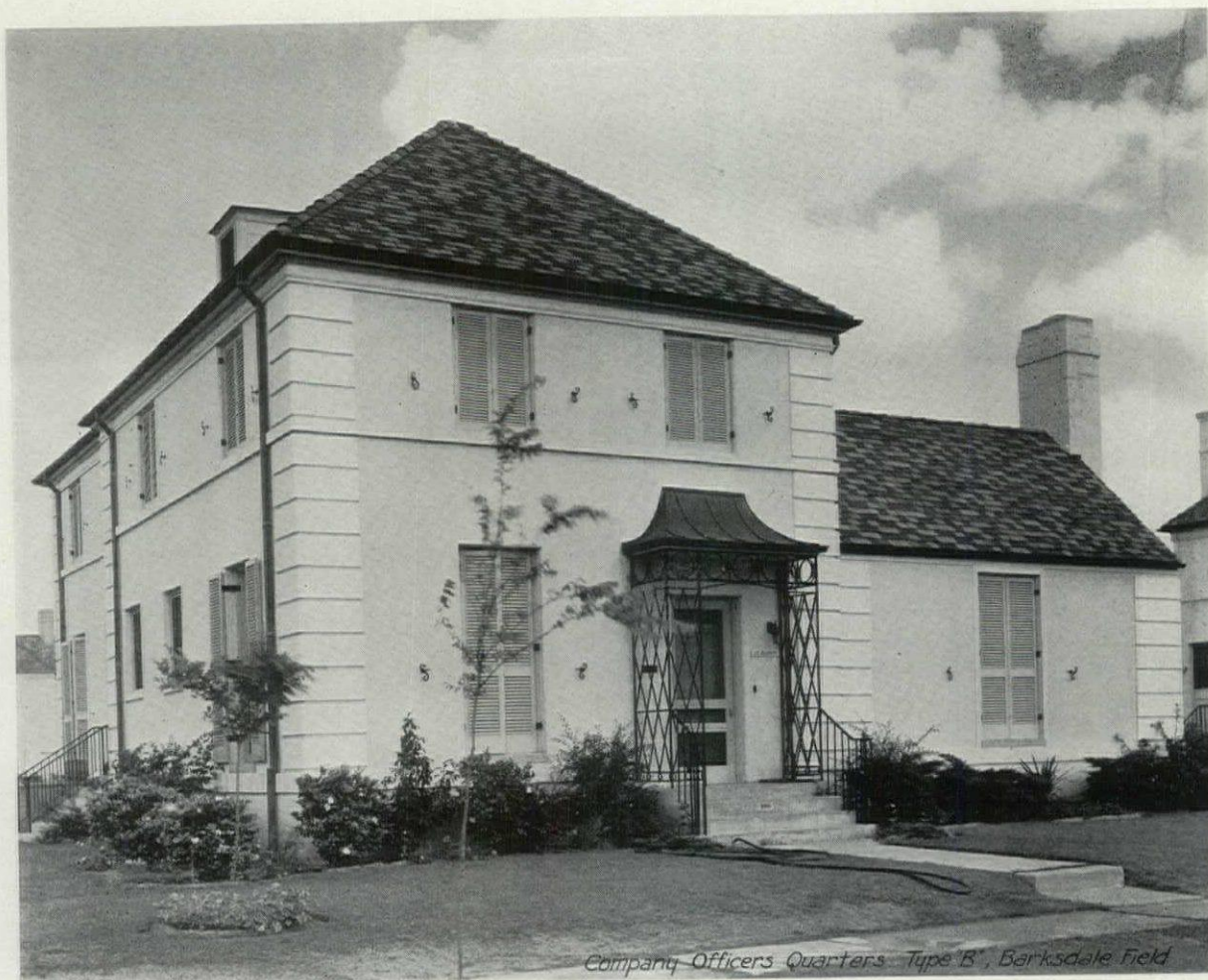
A type of house for a Company Officer at Berksdale Field, Louisiana, with the living room in one wing. Outside blinds are useful in this part of the country.
