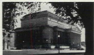
Archives Building (below)—G. A. Fuller Co., Contractor; Clyde R. Place, Consulting Engineer. "Freon" air conditioning equipment by York Ice Machinery Corporation.
