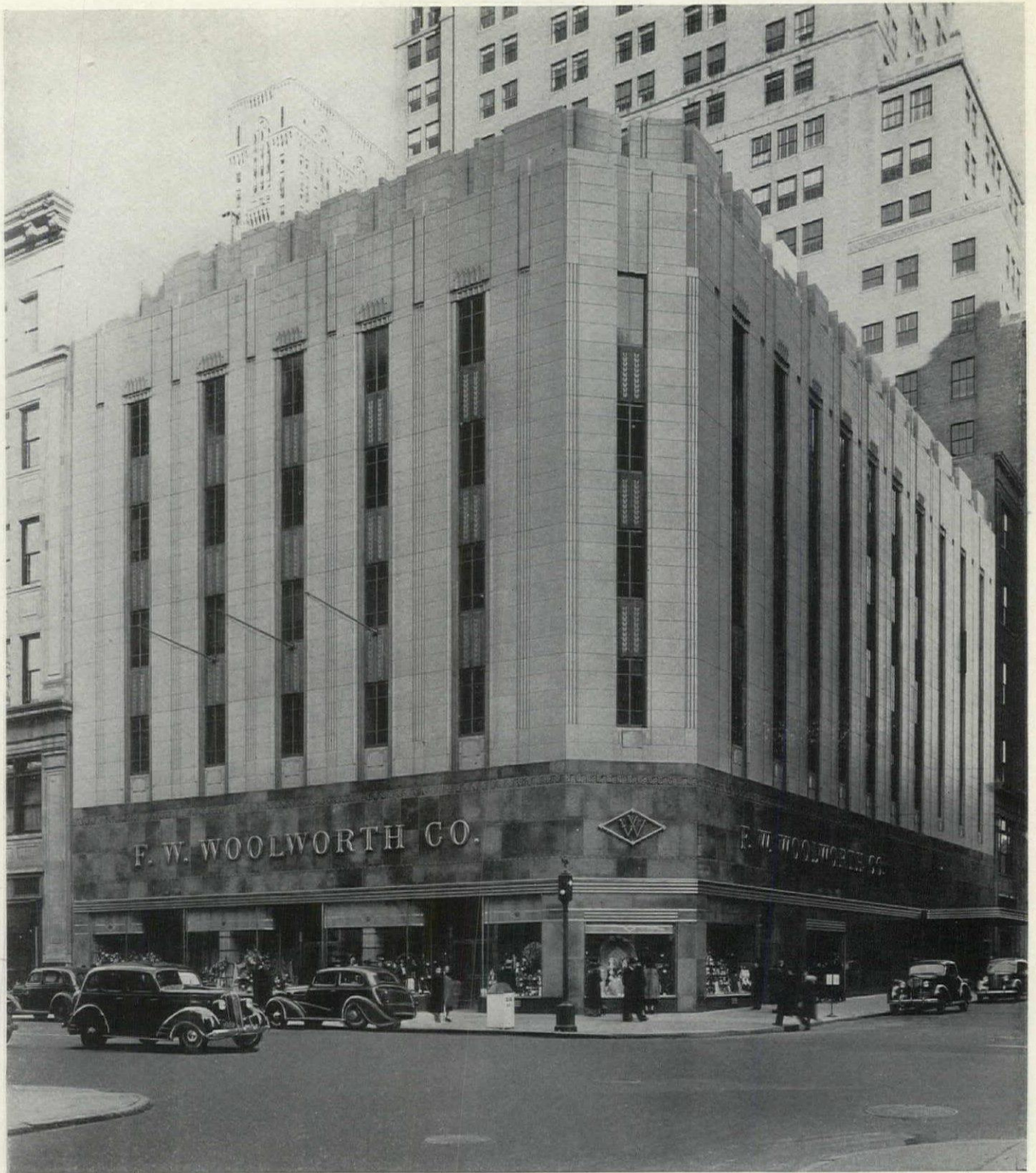
Building for F. W. Woolworth Co., N. E. Cor. 5th Ave. & 39th St., New York.
