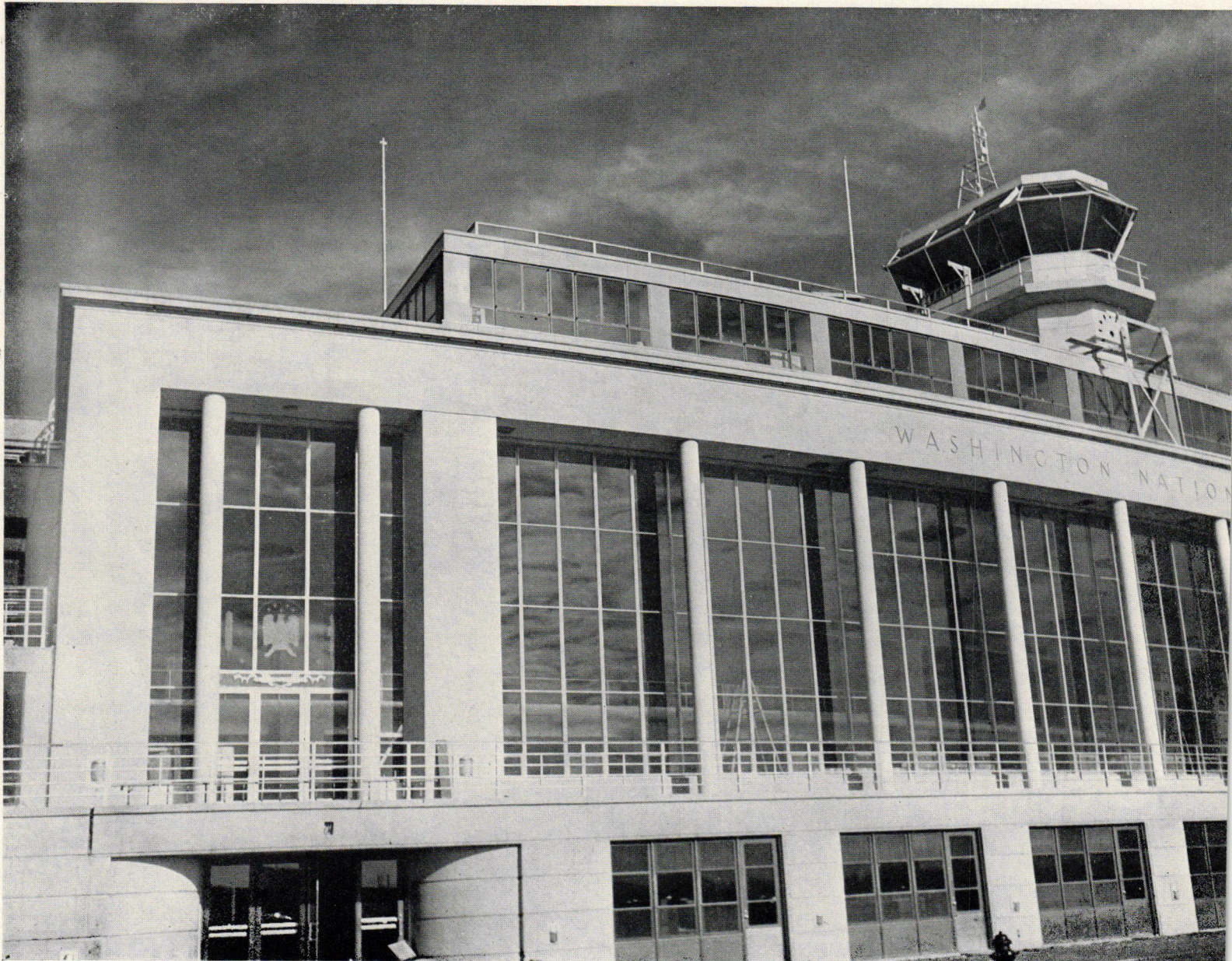
CLOSE-UP OF TERMINAL BUILDING From landing field, showing control tower.
