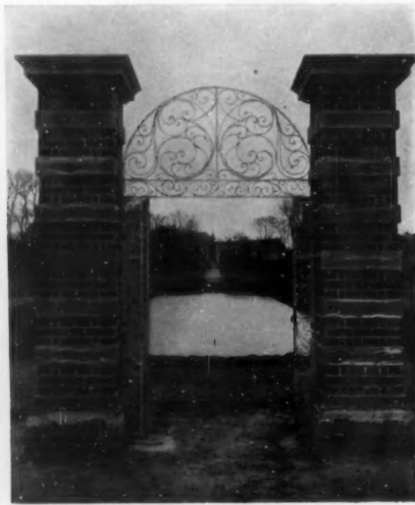
AN OLD SPANISH GATE AND GRILLE
