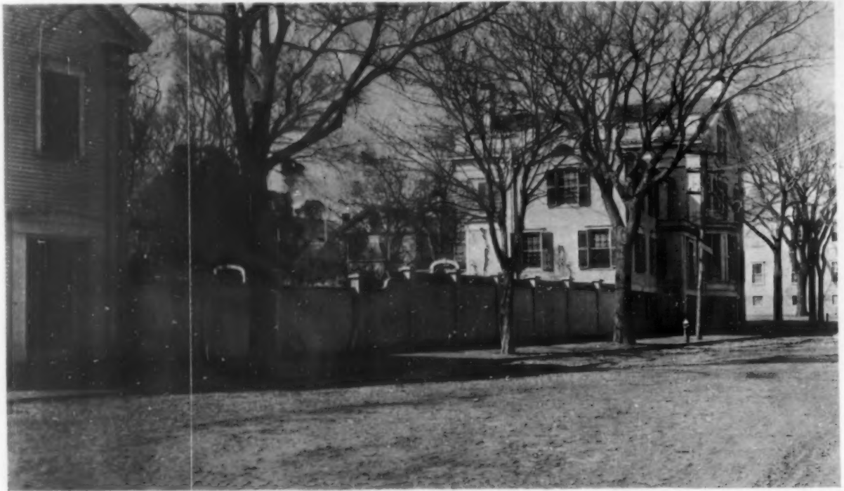
THE SANFORD PLACE FROM THE STREET
