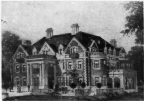
RESIDENCE OF A. R. PEACOCK, PITTSBURG ALDEN & HARLOW, ARCHITECTS
