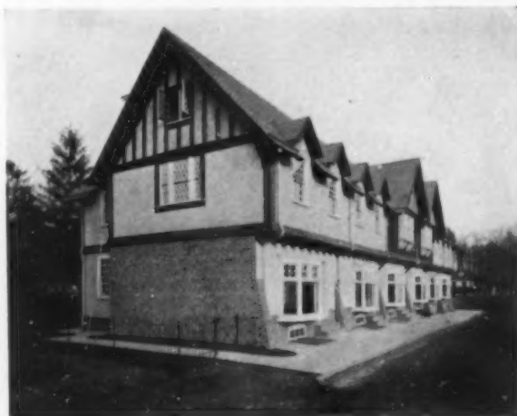
THE NORTH END OF THE ROW
