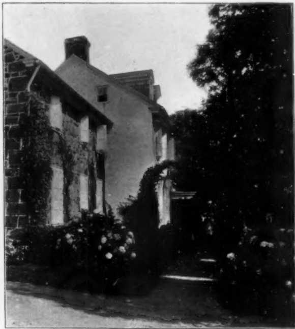
THE ENTRANCE TO THE TERRACE
