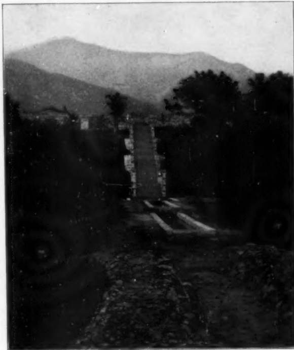
WORK NOW BUILT AT "EL FUREIDIS"
