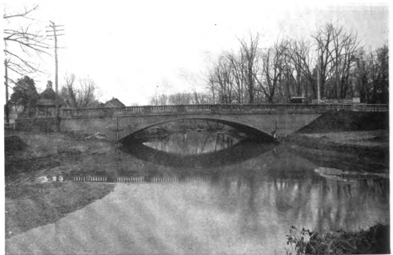
CONCRETE BRIDGE OVER POQUESSING CREEK, PHILADELPHIA. THIS BRIDGE HAS A SPAN 71 FEET WIDE, WITH A RISE OF 9½ FEET Cement Age
