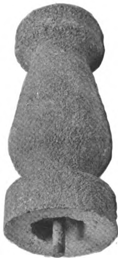
CONCRETE BALUSTER IN A PHILADELPHIA BRIDGE, SHOWING ROUGHENED SURFACE, SOMEWHAT LIKE PEBBLE DASHING
