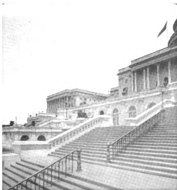
A NEARER VIEW OF THE WESTERN STEPS
