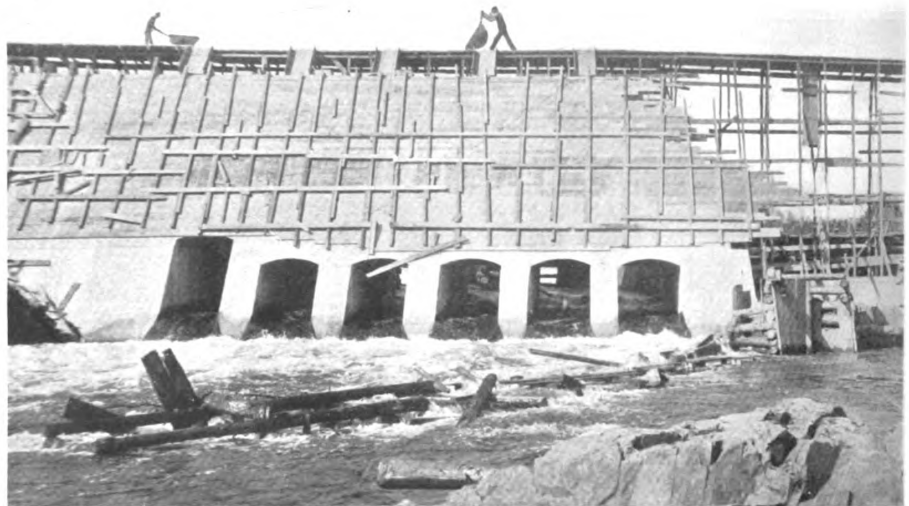
CONCRETE DAM AT SPRAGUE'S FALLS, ME.
