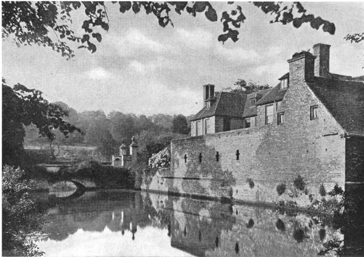
GROOMBRIDGE PLACE, KENT. THE WEST BRIDGE
