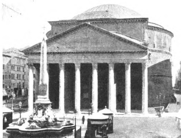
THE PANTHEON, ROME. BUILT A. D. 120. WALLS OF CONCRETE, FACED WITH BRICK
