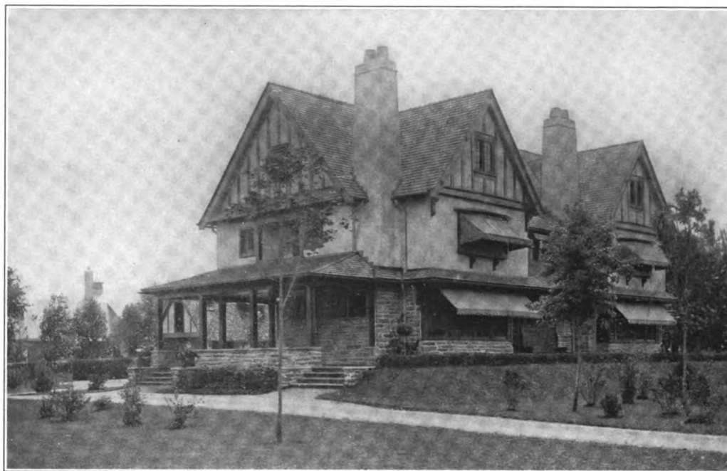
THE HOUSE FROM THE GARDEN TERRACE
