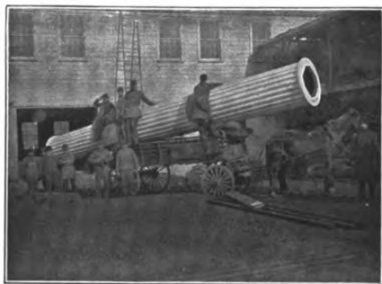
THE LARGEST "LOCK JOINT" COLUMN EVER BUILT 40 1/2 inches in diameter, 33 ft. 10 inches long. One of four furnished by us for the Portico of the Allenhurst Club, Allenhurst, N. J.
