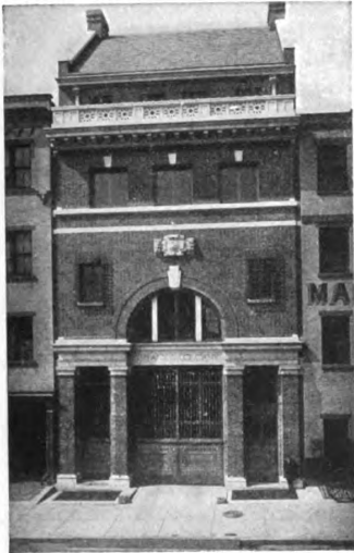
Tiffany Garage, 140 E. 41st St., New York McKim, Mead & White, Architects
