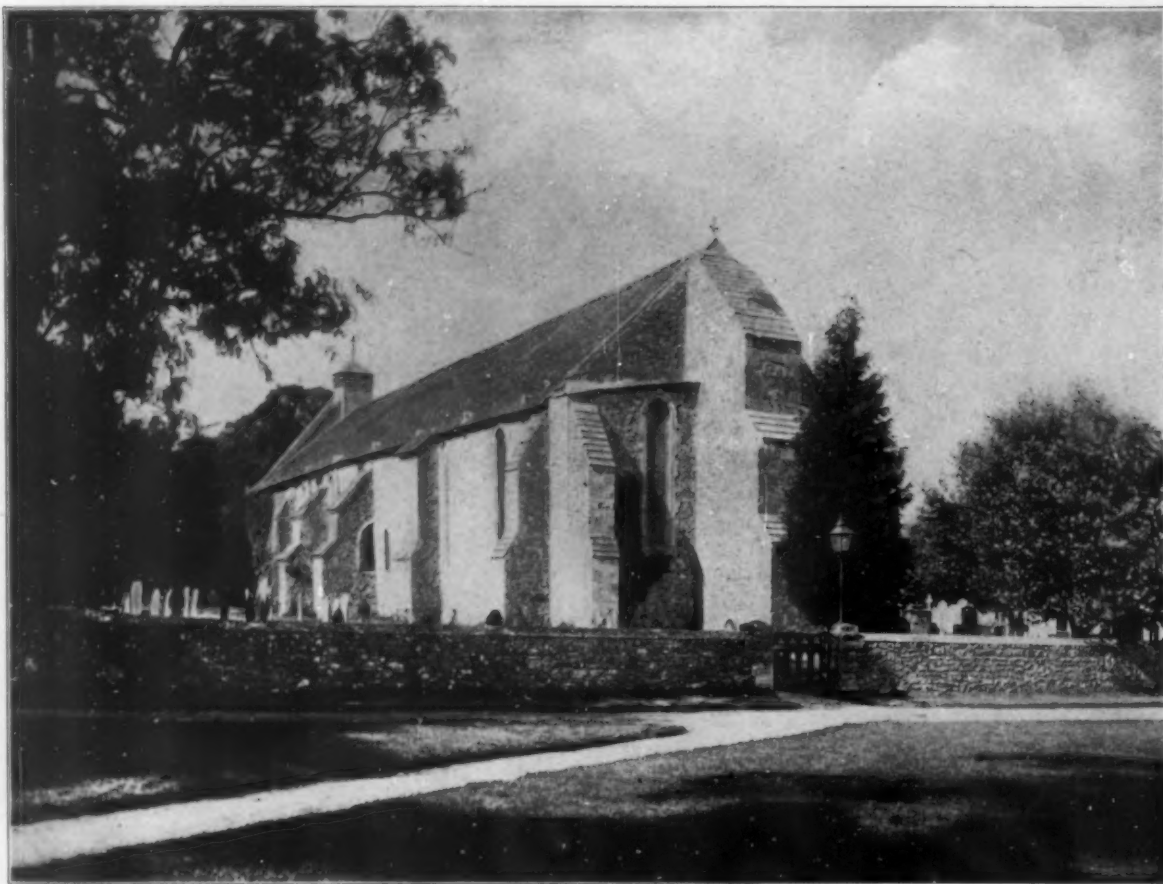
BEAULIEU PARISH CHURCH, FORMERLY THE REFECTORY
