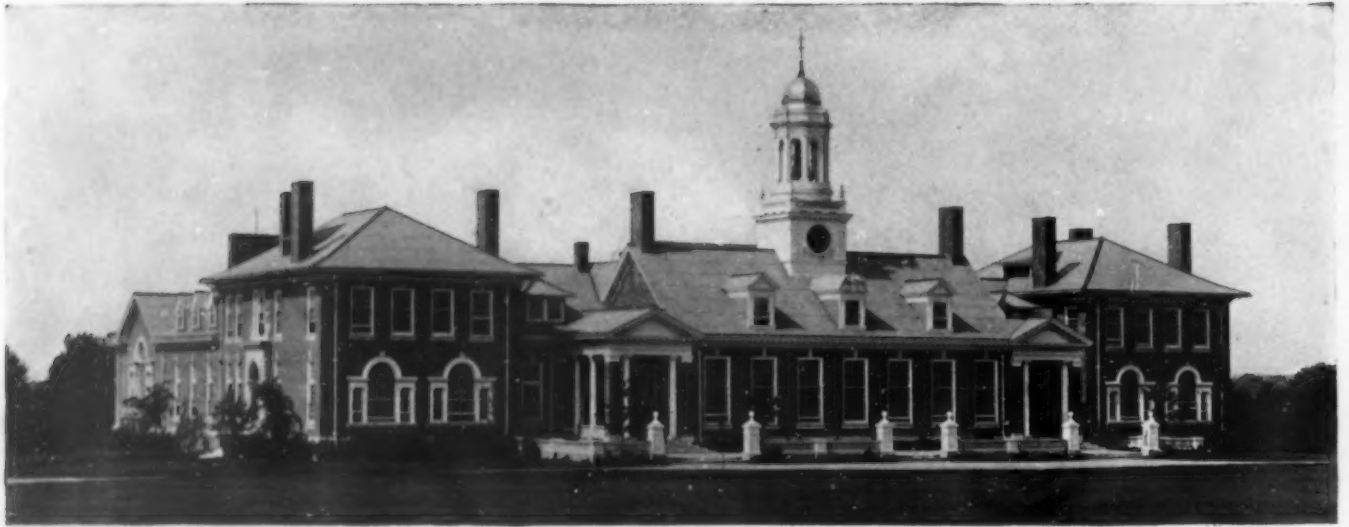
NEW BUILDING—GROTON SCHOOL
