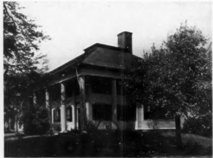
THE SANFORD RESIDENCE, BUILT IN 1832
