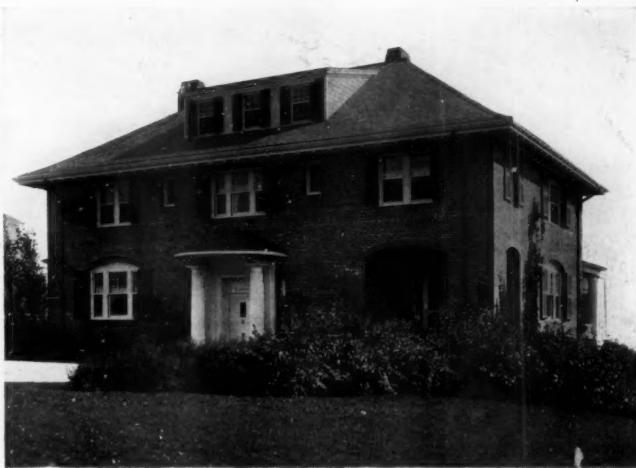
THE HOUSE ENTRANCE SHOWING THE QUAIN T ROUNDED HOOD
