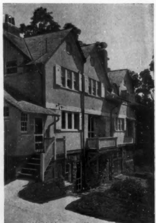
A light and accessible basement is entirely above ground at the rear. The central balcony opens from the dining-room
