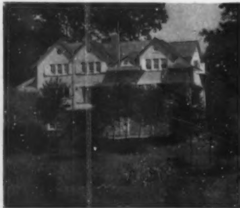
A warm gray stucco is used for the walls, with natural shingles and white wood-work, excepting a dull blue belt-course
