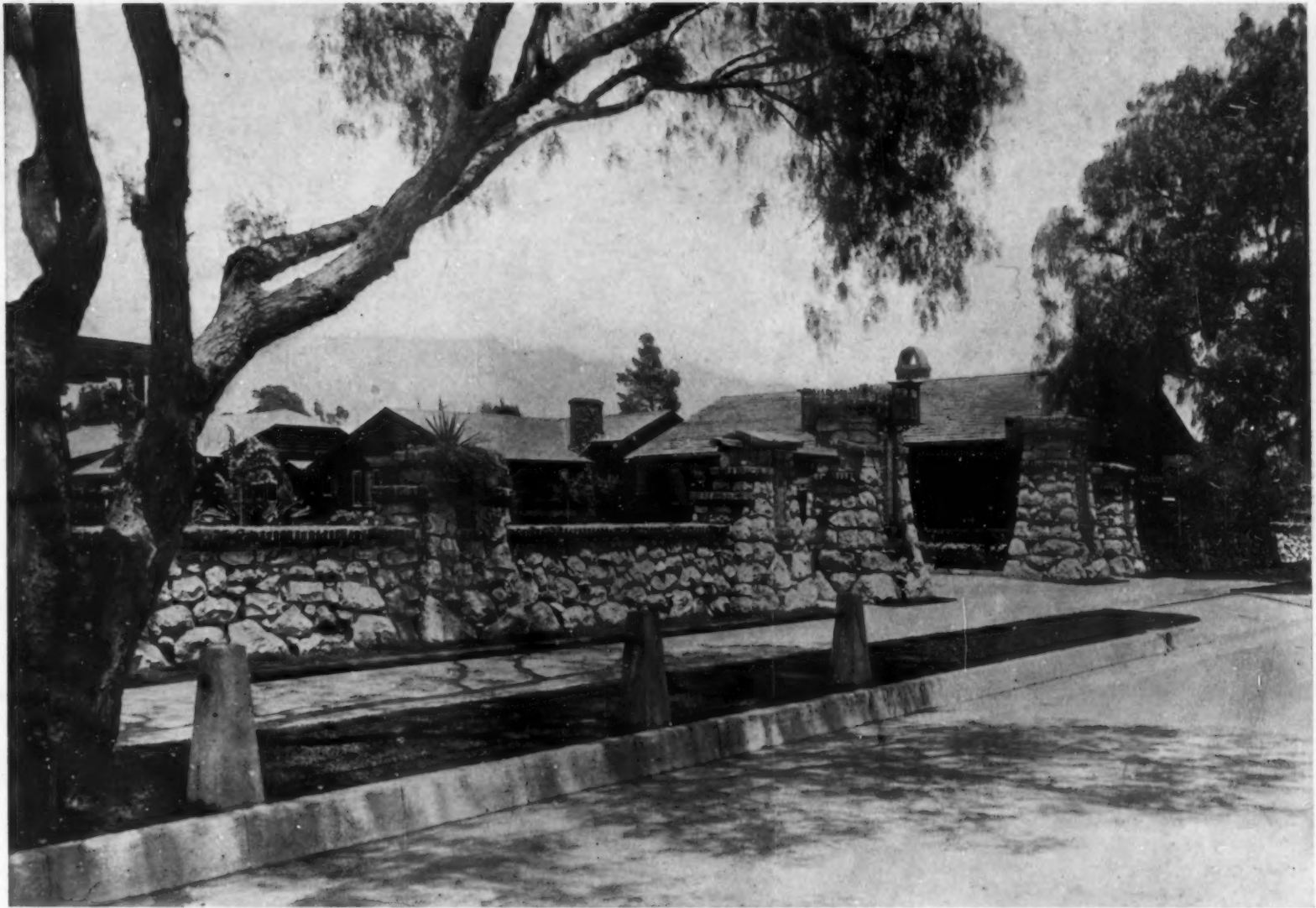
A wall, four feet high, of arroyo stones capped with clinker brick, broken by plant-bearing posts and central entrance gateway, bounds the western boundary line of the property
