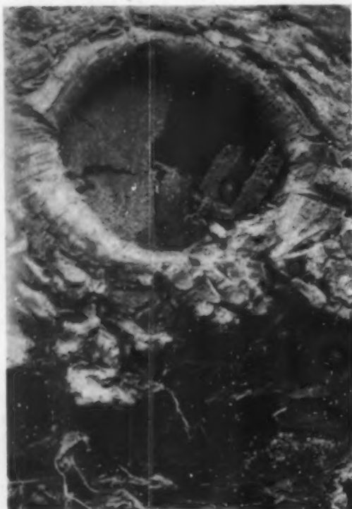
A wound, now become dangerous, that could easily have been cured at once by a dressing of coal tar; the latter is better than paint for the purpose
