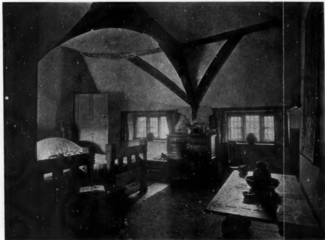
In the main bedroom, situated over the dining-room in the 14th century wing, the old framing of the roof timbers has been carefully preserved
