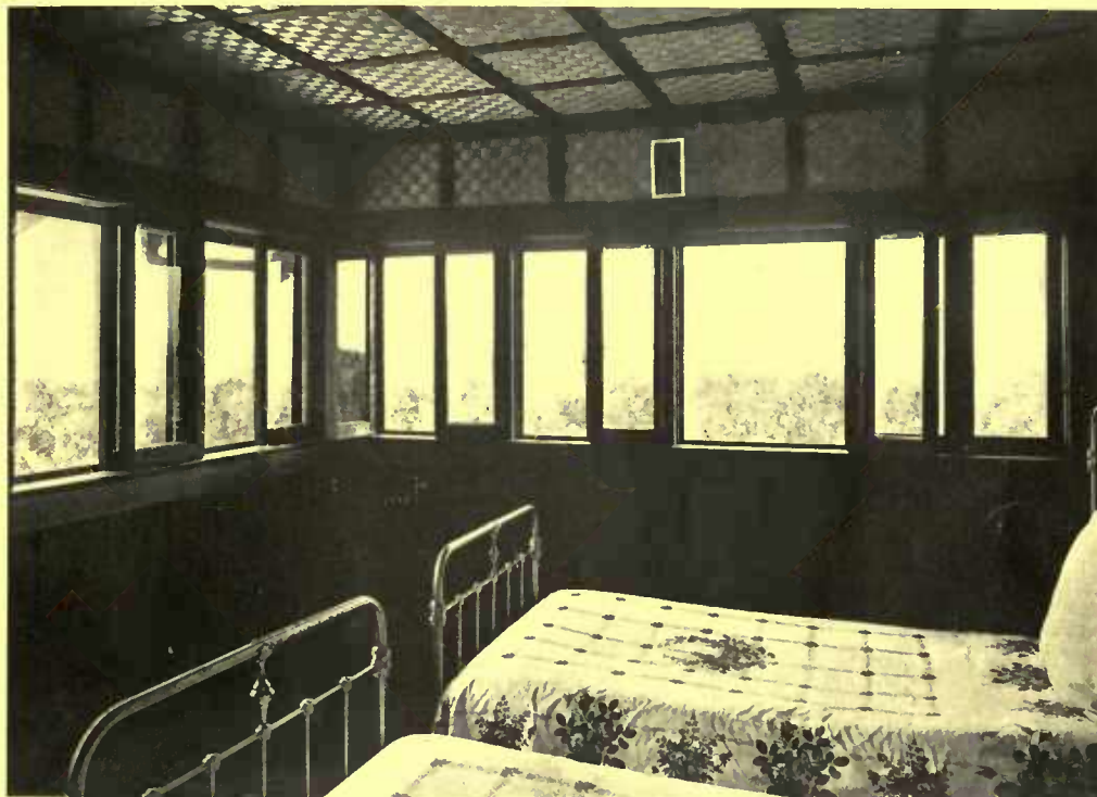
There is an air of fitness in the furnishing of this sleeping porch. The ceiling and frieze are covered with woven basketing held on by battens
