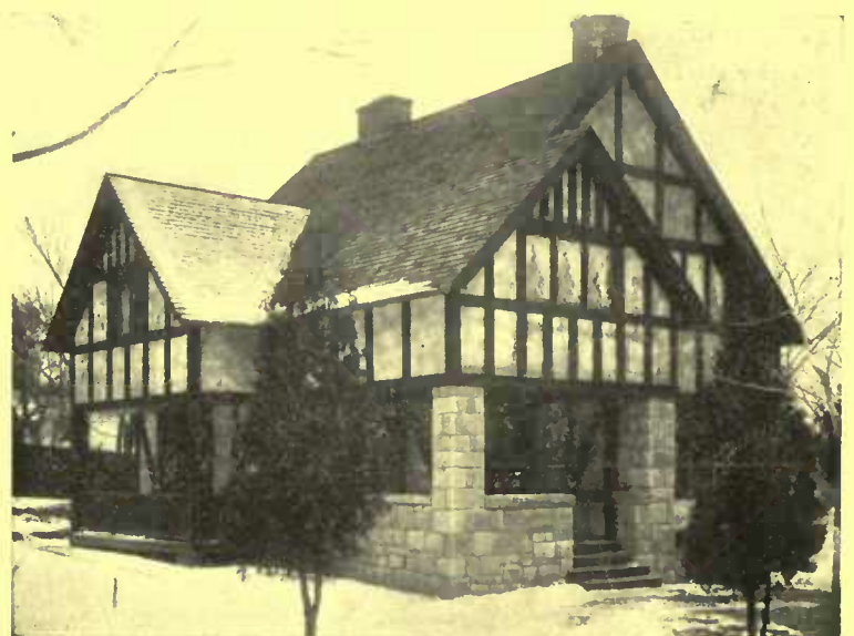
Half-timbering increases the cost of stucco on lath 5c a square foot. The stone foundation here is very expensive because of the carefully trimmed stone, and at the same time is less attractive
