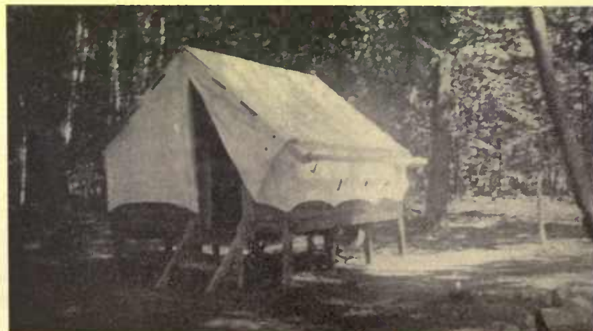
An ordinary canvas tent was stretched over the framework shown above and a raised floor constructed. In this the entire summer was comfortably spent
