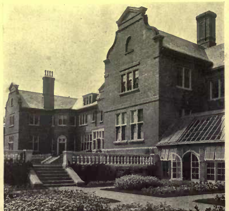
The effectiveness of terraces as evidenced in houses of the English Tudor type is shown in the Rice house at Ipswich, Mass. W. G. Rantoul, architect
