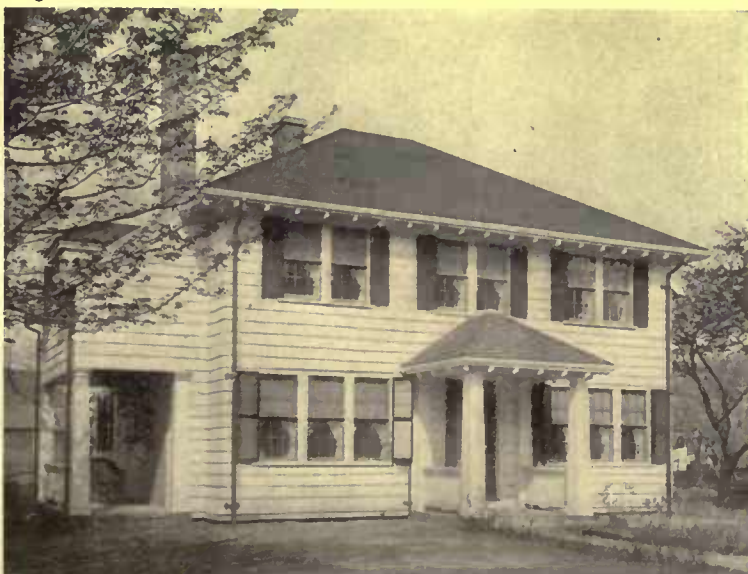
A painted clapboard house costs about 30c per square foot of surface. On side walls painted boards are more enduring than stone or shingles
