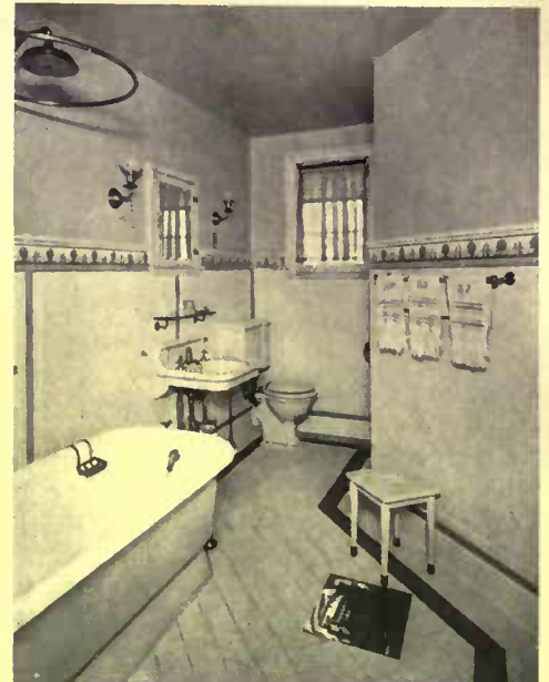
A tiled bathroom which gets decorative effect from laying tiles in herring-bone pattern
