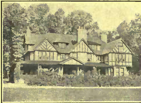
RESIDENCE AT ARDMORE, PA. Architects, Basley & Truscott, Philadelphia
