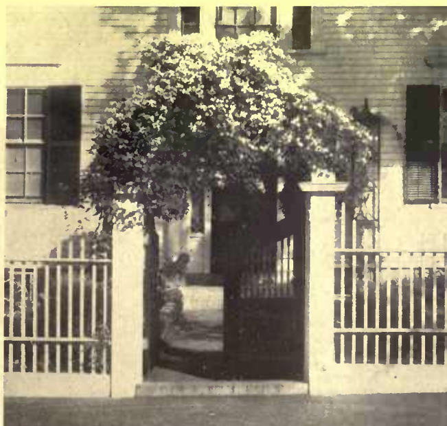
The entrance gateway swings a double gate with slender baluster grille
