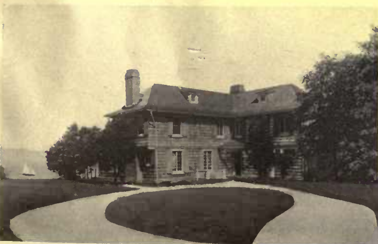
Shingles as a wall treatment are not so commonly used as formerly, but a successful treatment is shown in this house at Shoreham, L. I.
