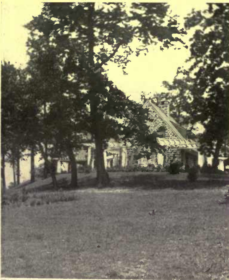
The gray stone house is set upon a woodland knoll and from the incurved front has an extended view
