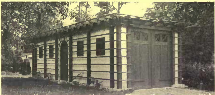
The garage is lattice covered and has an attractiveness often absent in buildings of this type
