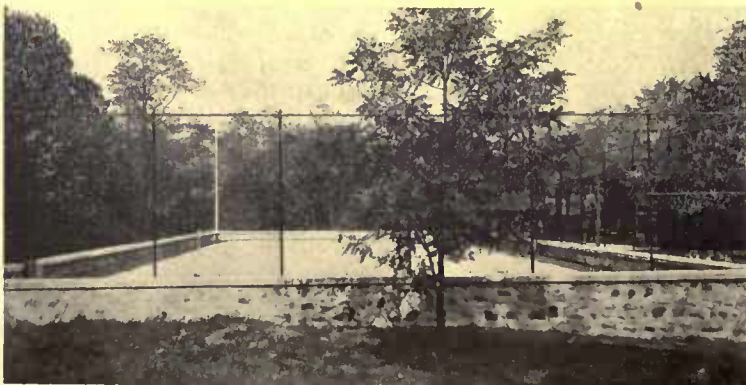
Sometimes a tennis court must have an outside foundation and must be built inside of stone retaining walls. It is durable but quite expensive
