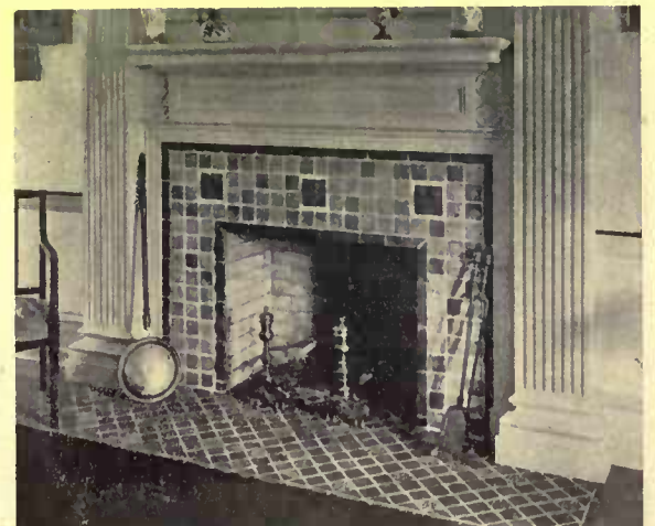
Where the appearance of hand work is desired the tiles are of varying sizes and each of different hue from its neighbor
