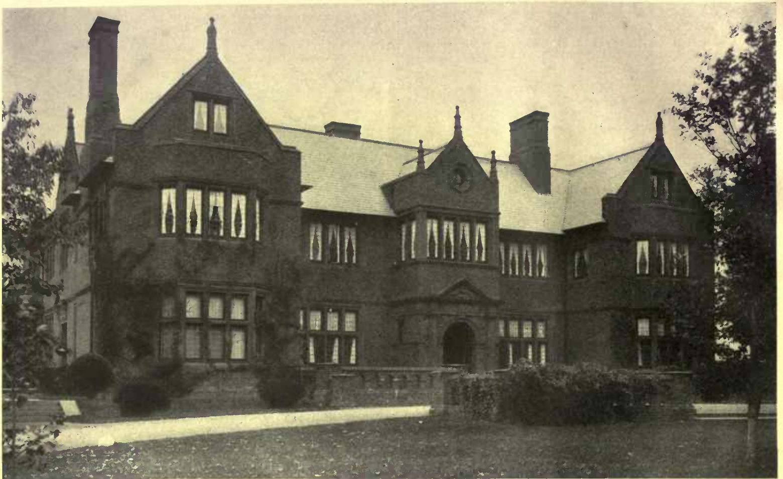
The house of J. S. Morgan, Esq., Pametos; Messrs. Cope & Stewardson, architects. In England the house builder's first consideration is to place the house so that the public, the master's and the servant departments will occupy the most logical positions in relation to the setting. This main entrance segregates the public part of the house entirely from the more private part, seen on page 18, top of page
