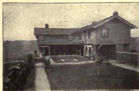
Stained with Cabot's Shingle Stains. Myron Hunt and Elmer Grey, Architects, Los Angeles, Cal.
