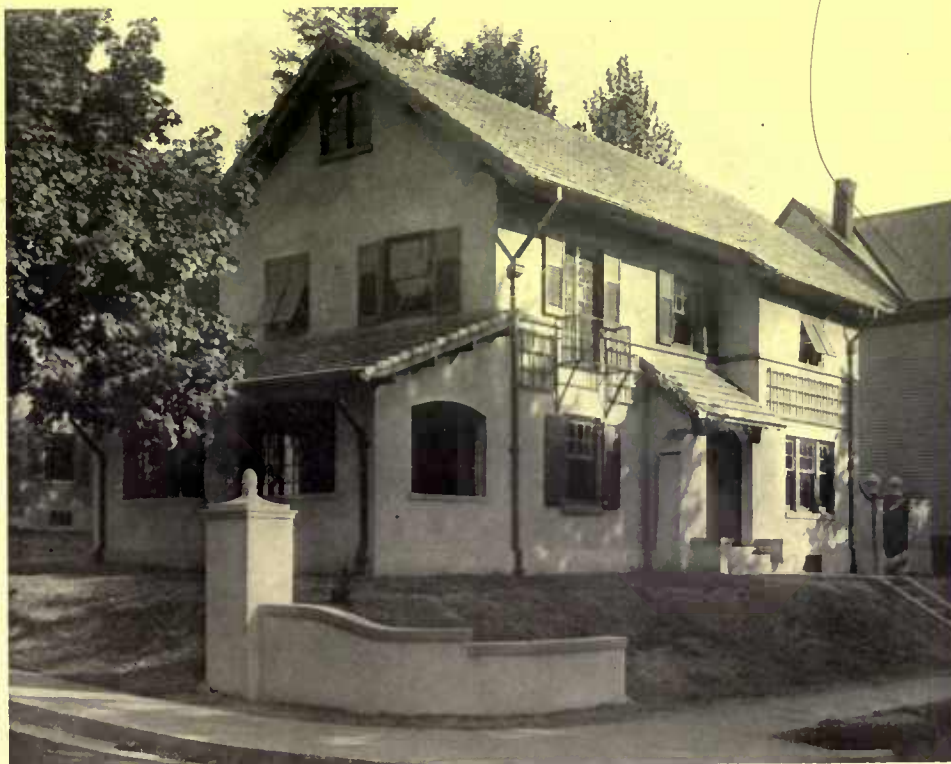
Where a site is comparatively level the leaders are run into tiles carrying the water into barrels of loose stones some distance away from the house underground
