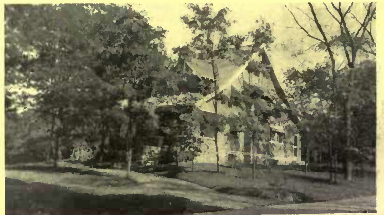
An interesting house for a timbered location is that of C. R. Tyng, Brantwood, Short Hills, N. J. James L. Burley, architect
