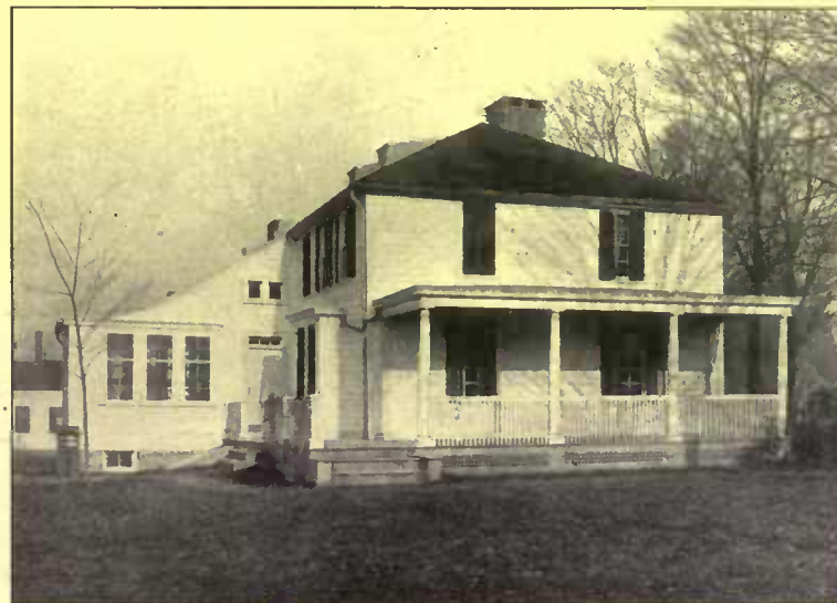
The porch end shows the square bay and the roof shape of the open air room ell
