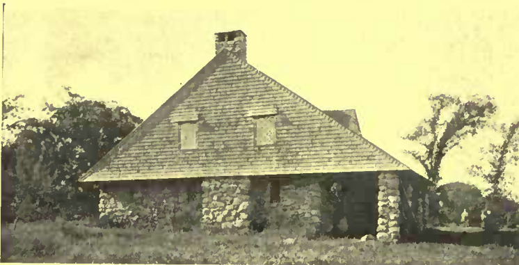
The upper part of this house projects on the farmhouse lines and forms a natural porch. This is a type planned for coolness
