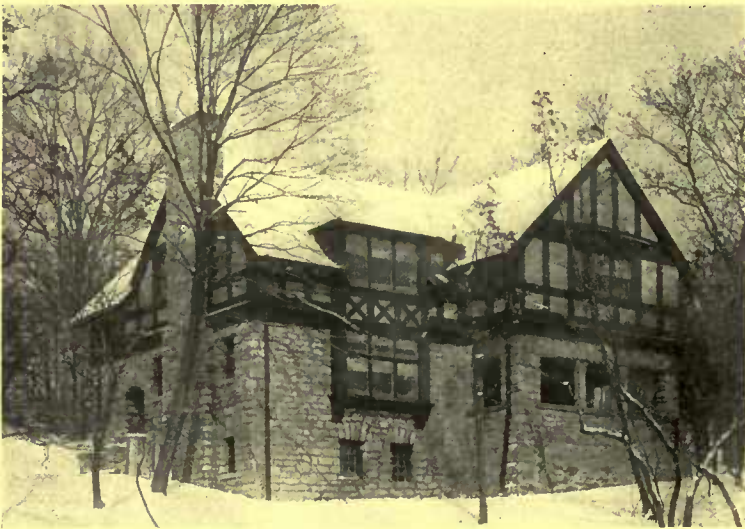
A half-timbered house of good style at Felston, Riverdale-on-Hudson, N. Y., that shows a happy combination of field-stone and timber work
