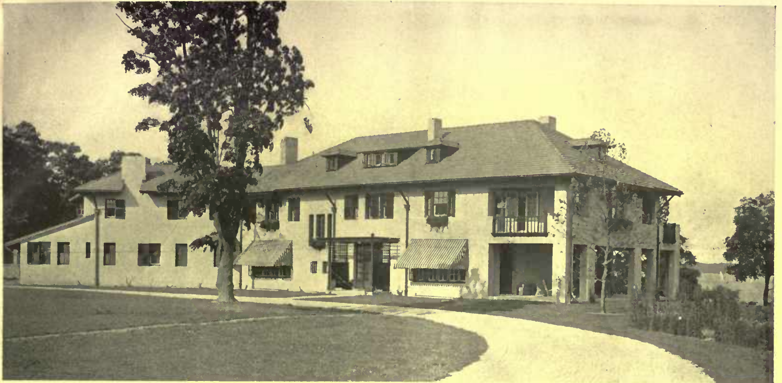
The Rush residence at Oyster Bay is an exceedingly fine example of a house well planned for its location. The long roof line takes off the apparent height, and the porch arrangement makes cool the rooms on the first floor. Clinton MacKenzie, architect
