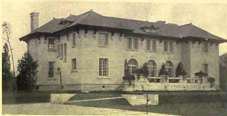
A modification of the mission type that preserves some of the distinctive features, yet is a suitable style for Northern localities
