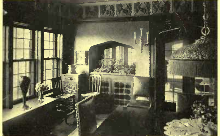
Here the walls have the suggestion of massiveness, so rough plaster is used, which permits a relief frieze in colors, but of the same material
