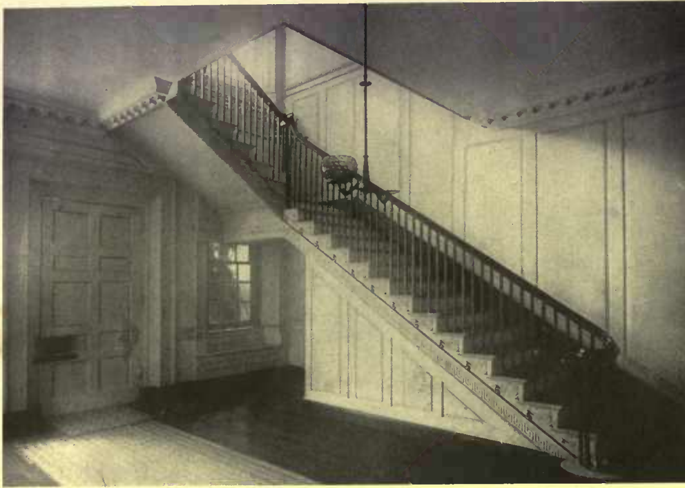
An old Colonial home where the panels themselves are extremely wide. We cannot secure such widths in boards to-day
