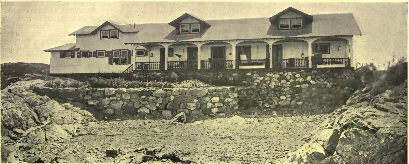
The problem of a porch is a different one with the seaside cottage. This is almost like the deck of a ship, and takes every advantage of the ocean breeze and permits a long promenade in unfavorable weather
