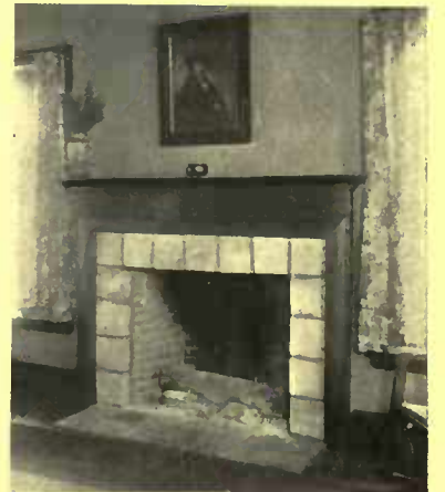
The mantel in the living-room is of waxed red gum with irregular tiles
