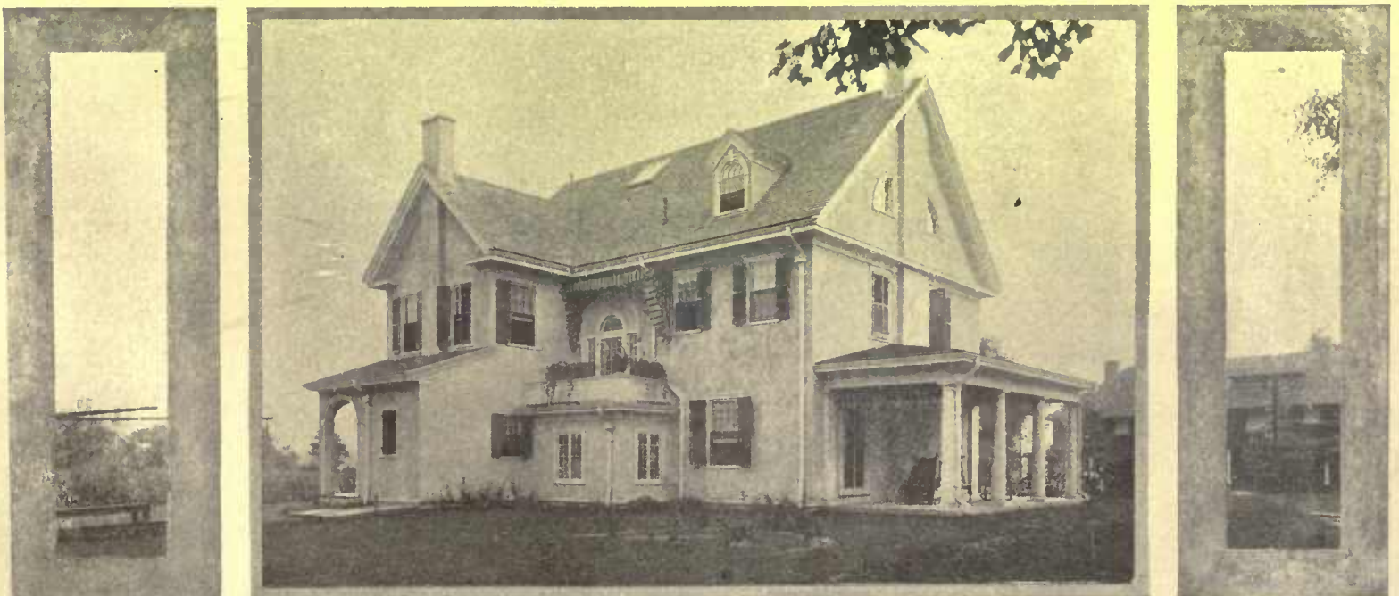
A small balcony much in demand when outdoor seclusion is required is built over the roof of the den. The decorative window contains a door opening out from the stair landing
