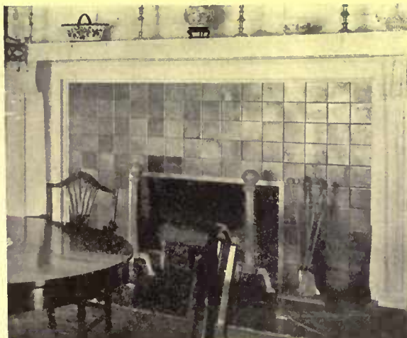
Where the tiles are uniform in size an interesting decorative feature is obtained through the use of various shades of the same color
