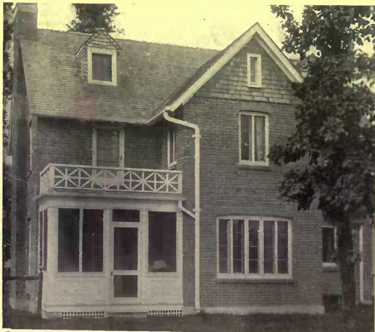
One point of note is the good finish of the rear elevation, which is of equal dignity with the front
