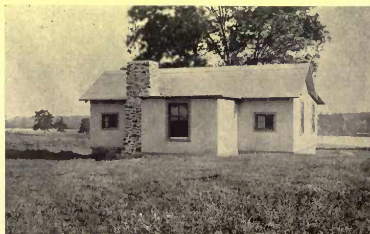
A rear view of the bungalow shows the huge chimney built of stones from the nearby river
