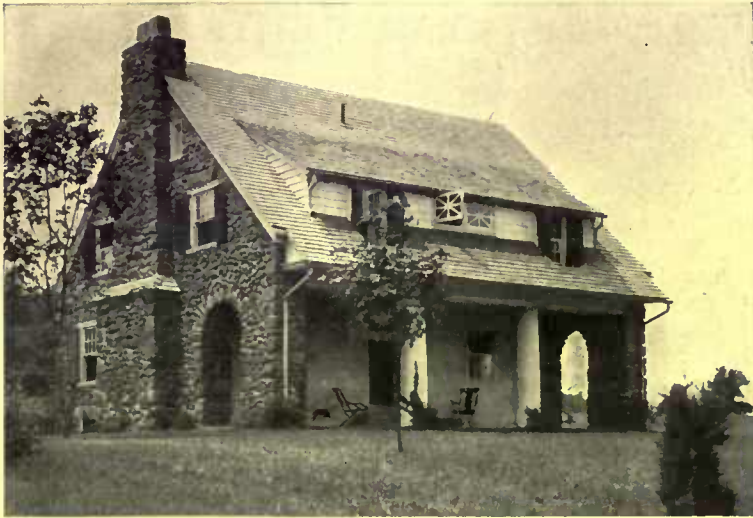
Where stone is used, a wall of cobbles is the most economical. Here only the end walls are stone; the rest, covered by the projecting roof, is of stucco over a frame wall. Charles Barton Keen, architect
