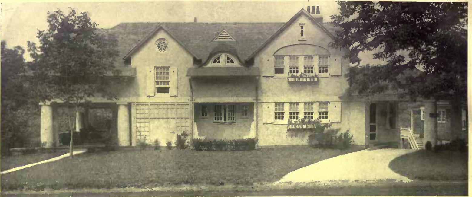
The home of Dr. R. R. Ryan, at Scarsdale, N. Y., is a pleasing American type of the plaster house that had its origin in England and has been developed by such architects as Parker & Unwin. The use of solid shutters beside small paned windows is particularly effective here
