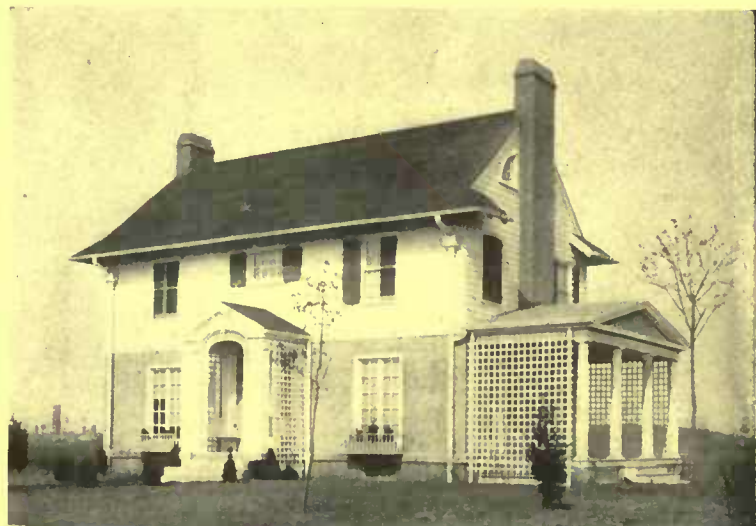
An interesting effect is obtained in this simple house on the Garden City Estates by uniting stucco and concrete in the wall treatment
