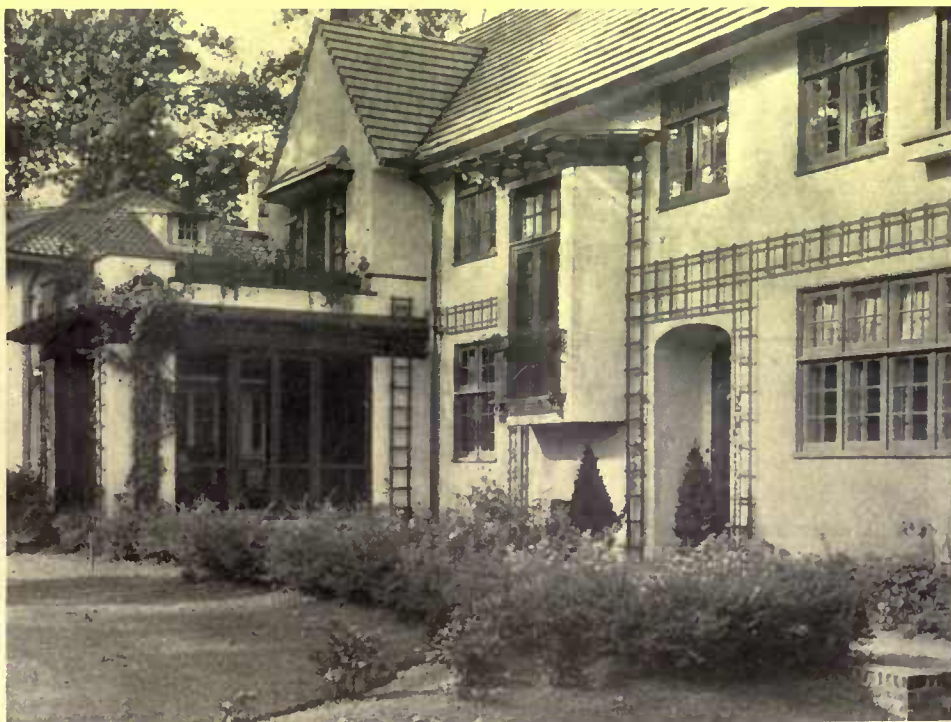
All impression of bareness is relieved by the use of a simple lattice running over the larger blank spaces of the walls
