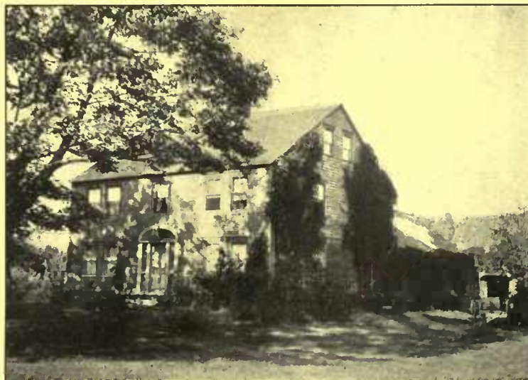
Such a building as this has possibilities for making a livable and attractive home
