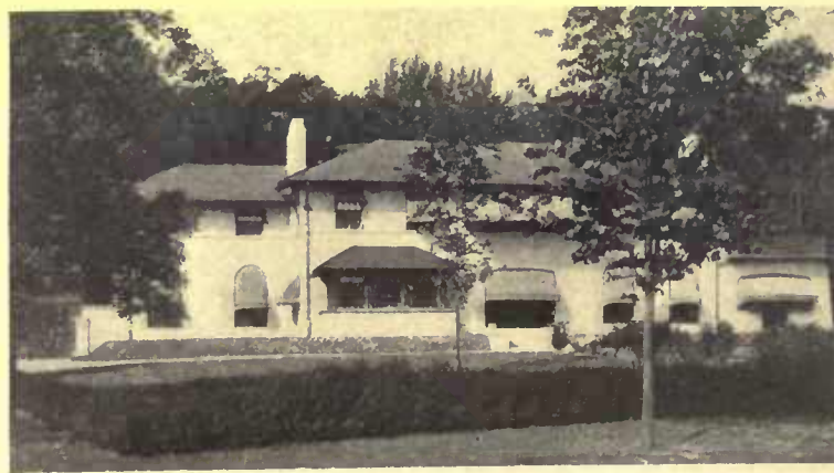
Mr. Jewett's house at Englewood is a noteworthy example of simplicity in the wall treatment of plaster houses
