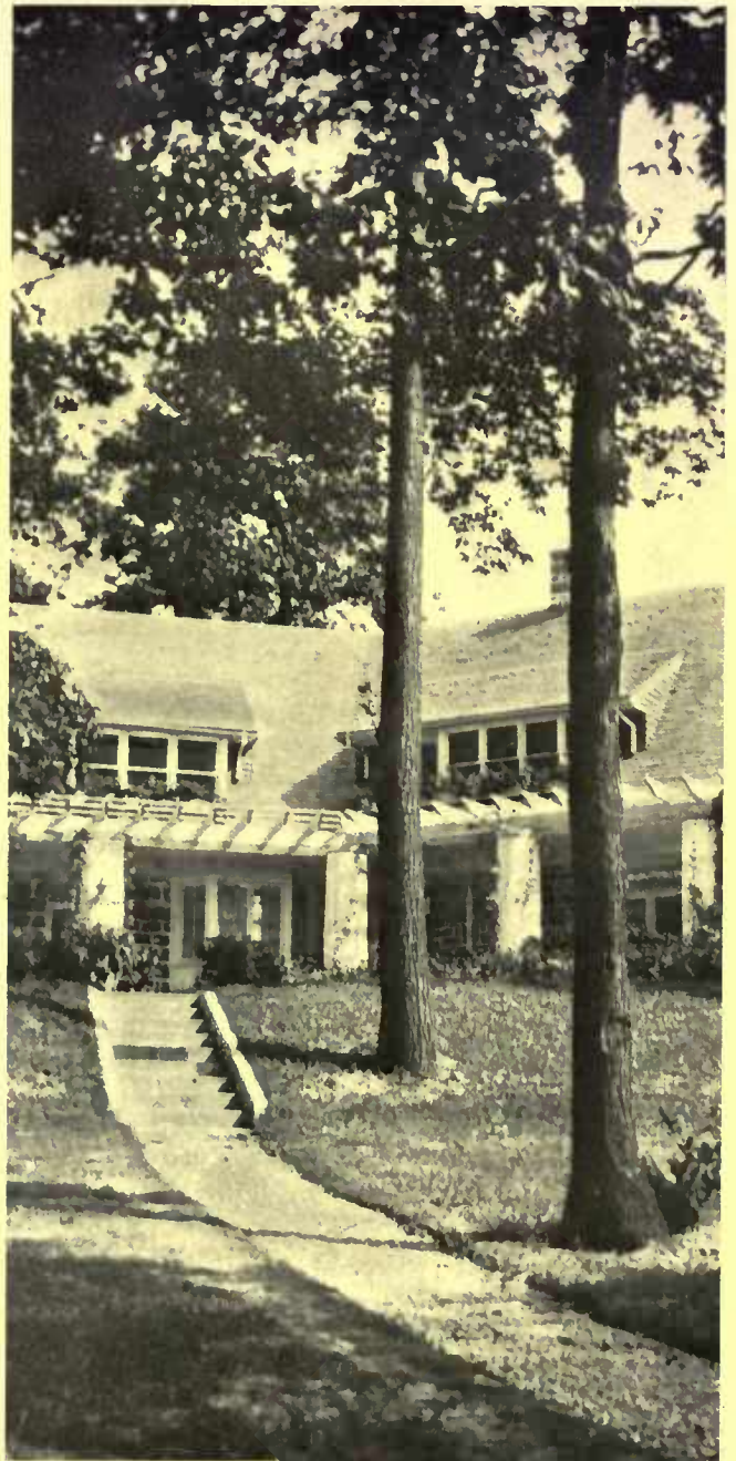
The pergola about the house is a unique feature, but calculated to give just the right amounts of shade and sunlight
