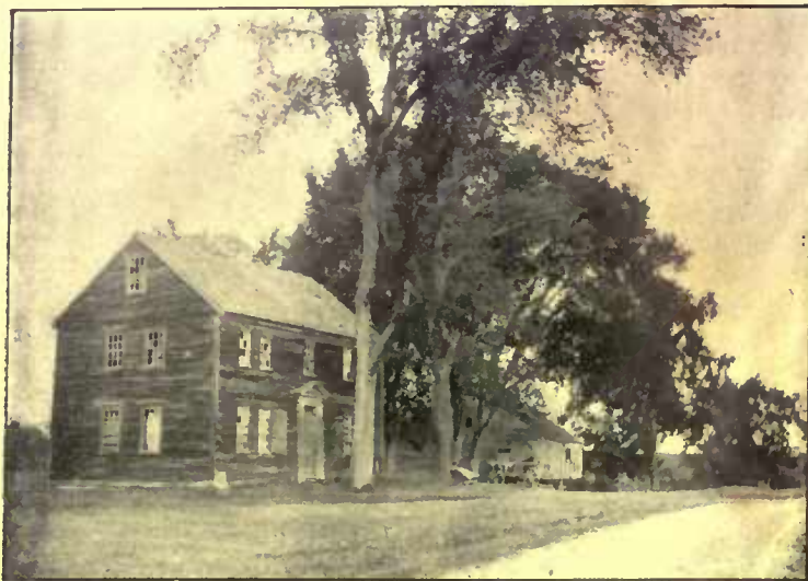
A Southern Maine house which is worth the time of examination for remodeling
