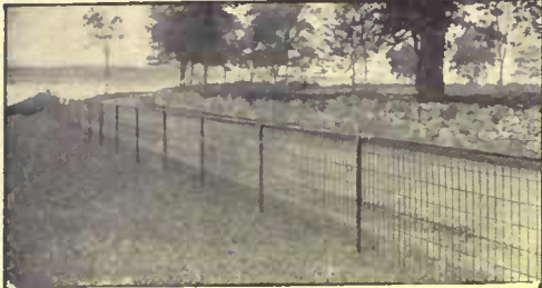
Woven wire fence at Saugatuck, Conn., erected on Anchor Posts.
