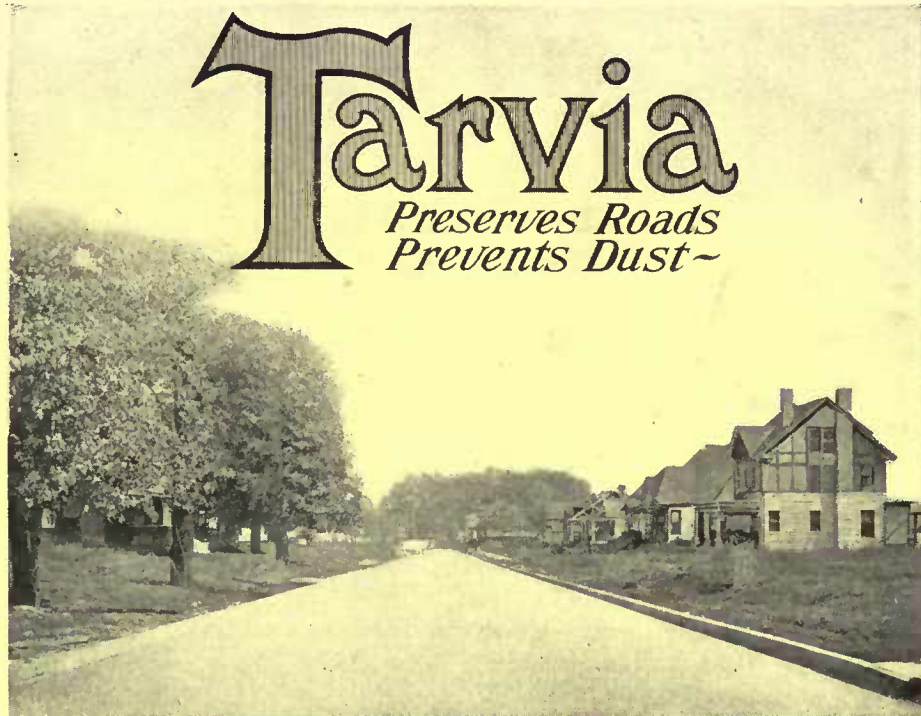
Cowden Avenue, Memphis, Tenn. Constructed with Tarvia X.
