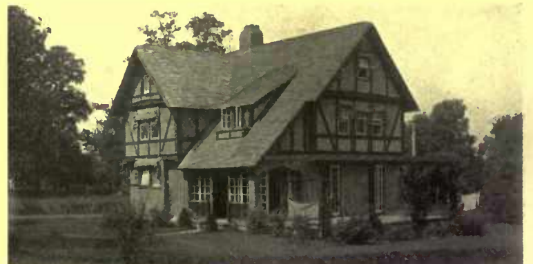
Shingle thatch is often used successfully, as in the house of George C. Holten at Great Neck Villa. E. W. Hazzard, architect
