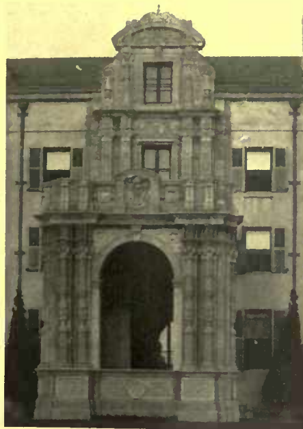
A Spanish doorway on a house at Rye; Cram, Goodhue & Ferguson, architects
