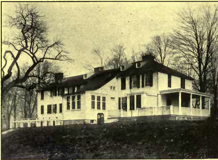
The rear is the river elevation and from this open air room the outlook is of the very best
