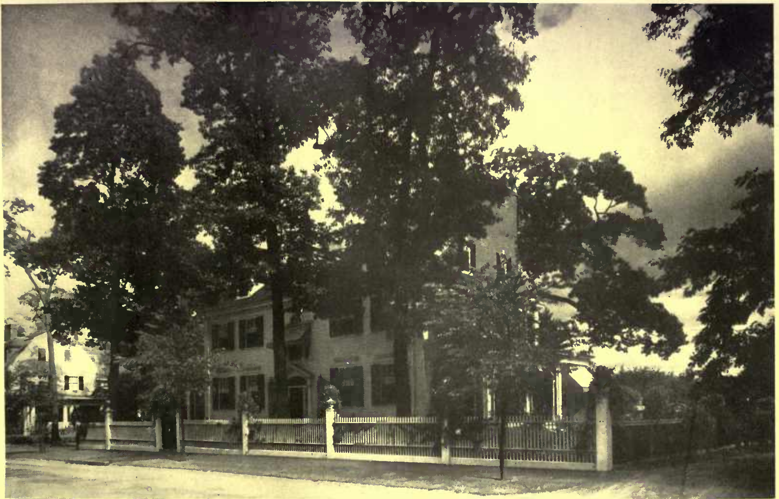
The home of B. F. Pitman, Longwood, Mass.—Kilam & Hopkins, architects. The straight lines of the fence are broken by the vine-covered posts and gateway; the white wall is shaded by three great trees
