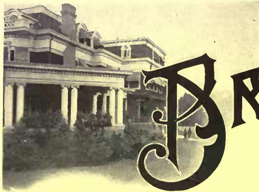
Residence of Mr. T. A. Sperry, Cranford, N. J. Equipped with Brunswick Refrigerating Plant.
