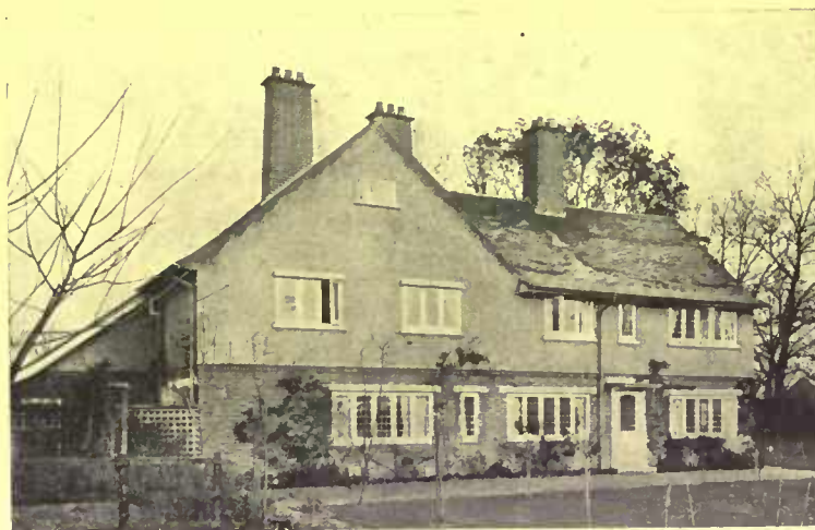
A very good combination is made of brick wall below and stucco over brick above. The cost per square foot averages 66c
