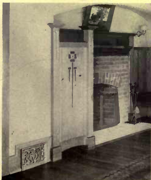
Wall registers are made in an infinite variety of patterns and can be had to coincide with the decorative scheme
