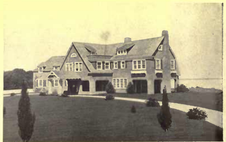
Plaster seems to be the most successful material for the exposed position on salt water. The residence of William T. Ashley, Shoreham
