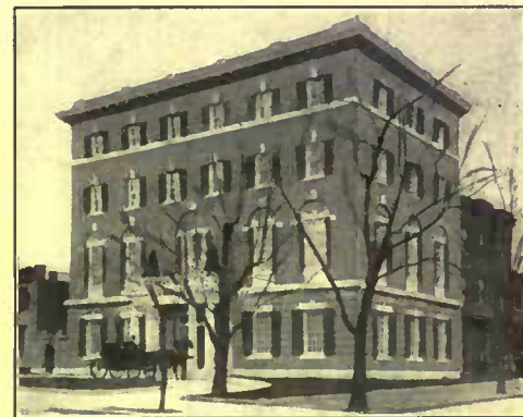
Kelsey Heated Residence, Washington, D. C. Mr. J. H. De Sibour, Washington, Architect
