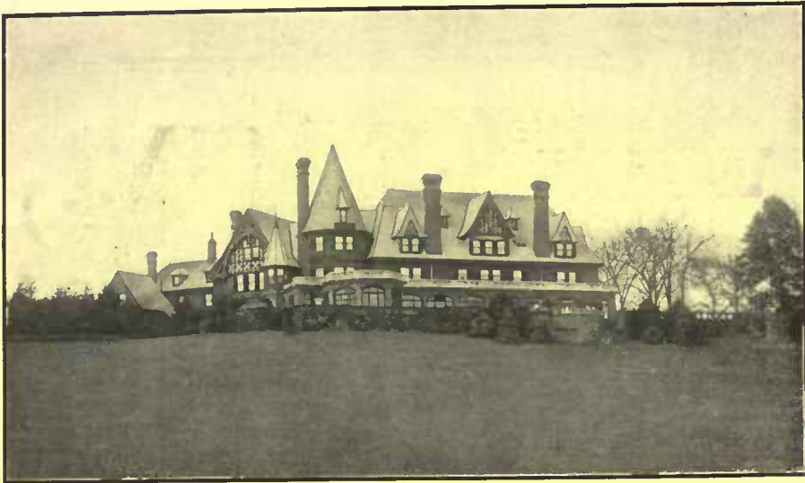
Asbestos "Century" Shingle Roof—Quintard Estate, Portchester, New York
