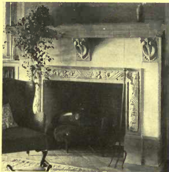
Tiles often are used for this entire fireplace and mantel. Here they have all the beauty of bas-relief carving
