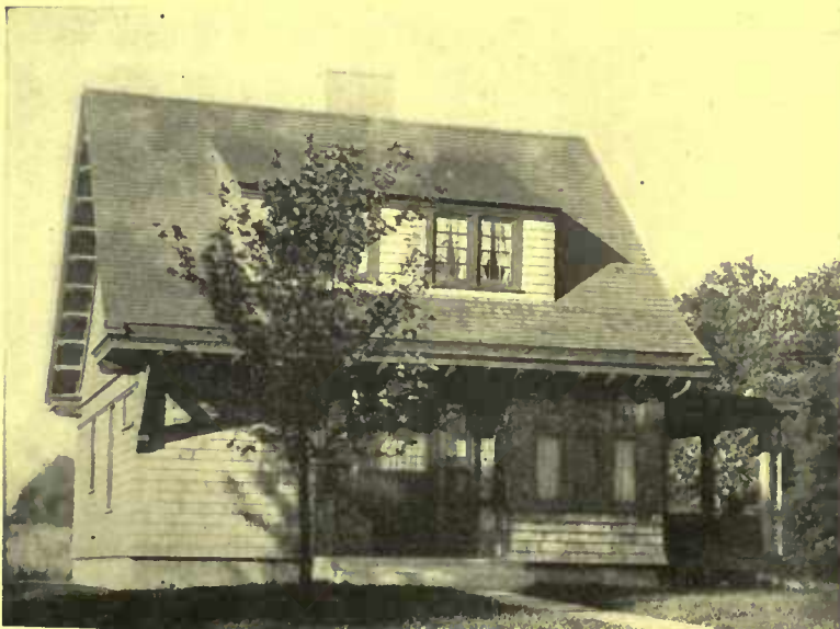
Shingles over a frame wall are the least expensive material to be used. This little house is especially economical because of its shape—a square house can be built for less than one with wings or ells
