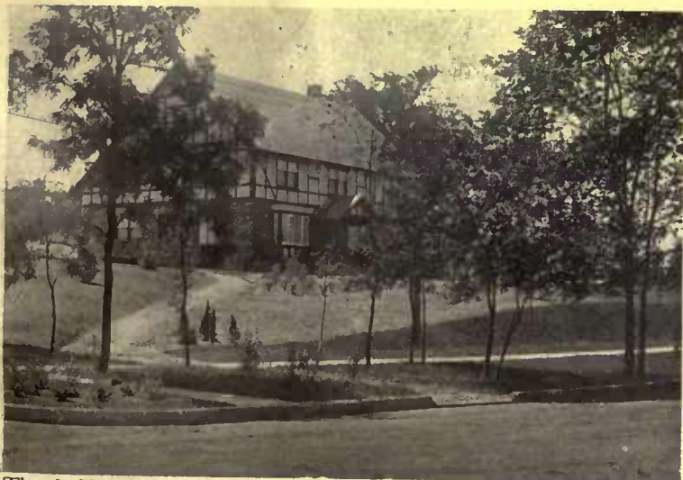
That half-timber work may well be combined with a local stone foundation is shown here in the home of Mr. A. C. Ayer at Scarsdale
