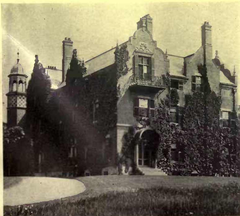
When Mr. Cabot built his house in Brookline it was to fit the site of a house destroyed by fire. He chose the freedom of English lines to do this satisfactorily
