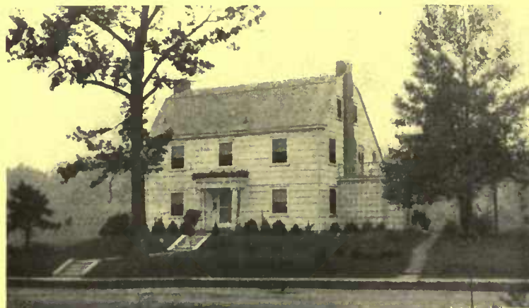
The home of Hutchinson Hinkle in Short Hills, N. J., is an interesting variation of the gambrel roofed house in that it has no front dormers
