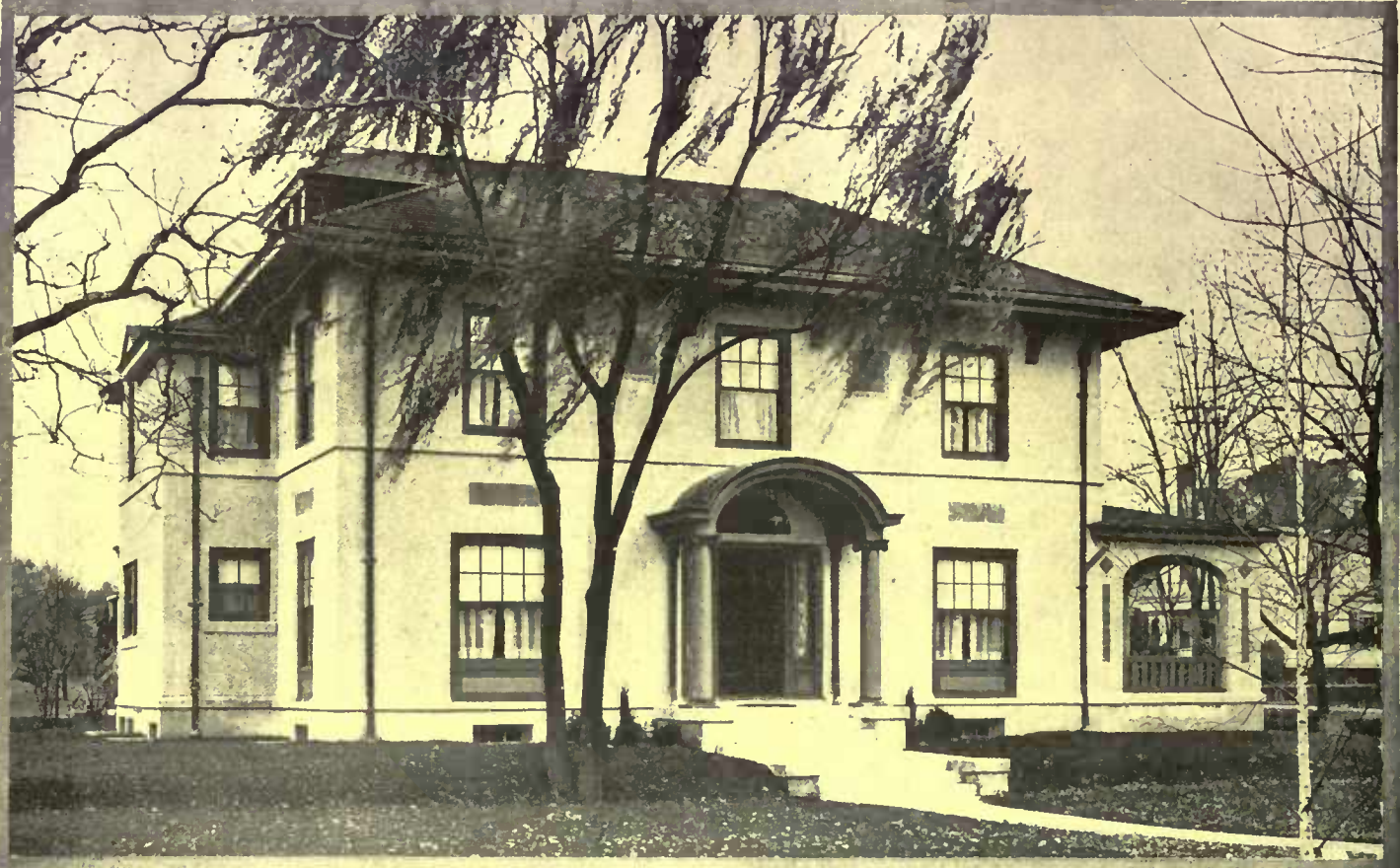
There is a sense of dignity and simplicity about this stucco house that comes from its rectilinear lines and plain, broad windows. Color is obtained by the use of the inlay brick panels
