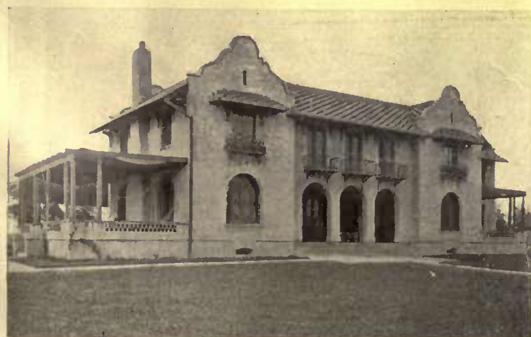
The arched doorways and gable ends here are mission characteristics; the porch is an addition not found in the prototypes
