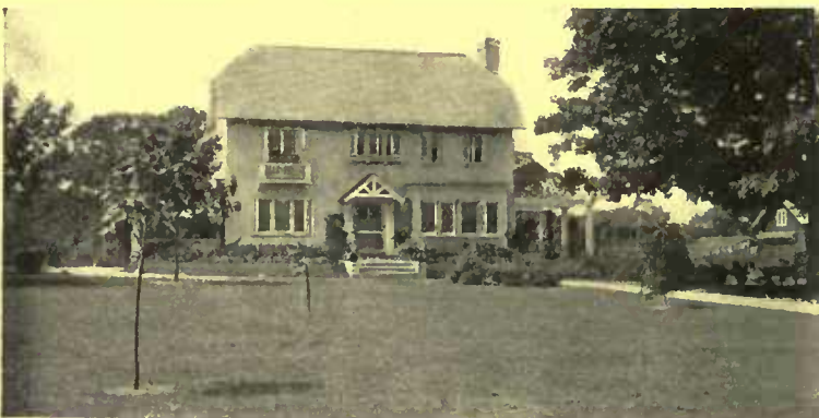
This house of Mr. Minton at Brightwaters, L. I., shows the pleasing effect of the jerken-head roof so much used abroad
