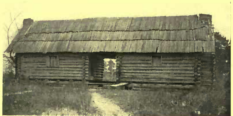
An idea for a camp was taken from the negro cabin roofed with shakes. The ends are living quarters, the open space between, the dining-room
