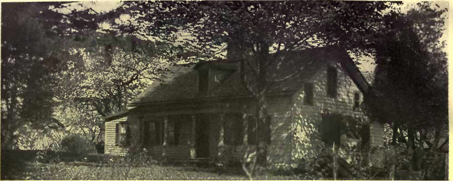
In Connecticut there is many an opportunity to find a home about which the charm of age still clings. An attractive little house near Stamford that was built over a hundred years ago yet is still in good condition and suitable for remodeling
