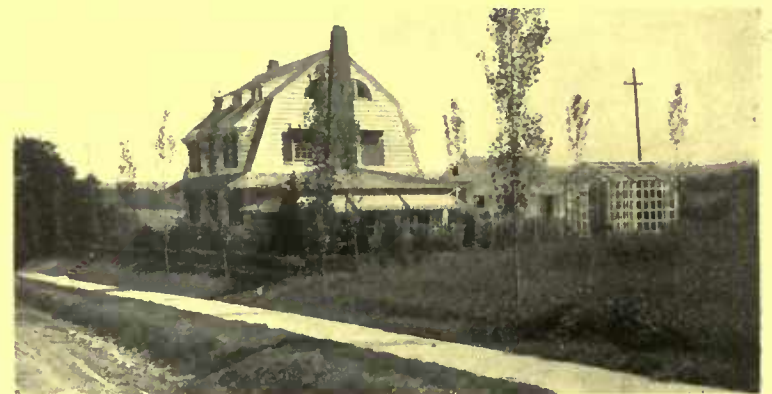
A house at Great Neck Villa, L. I., that obtains a maximum of space by the use of two dormers. Miss Chapman, architect
