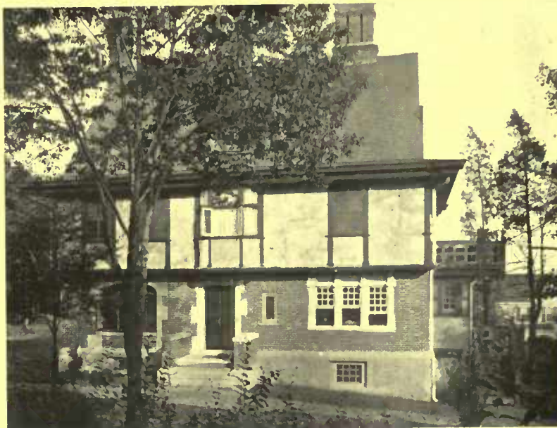
See that the rain leaders carry the roof water to the lower side of a sloping site, unless the foundation wall is amply protected
