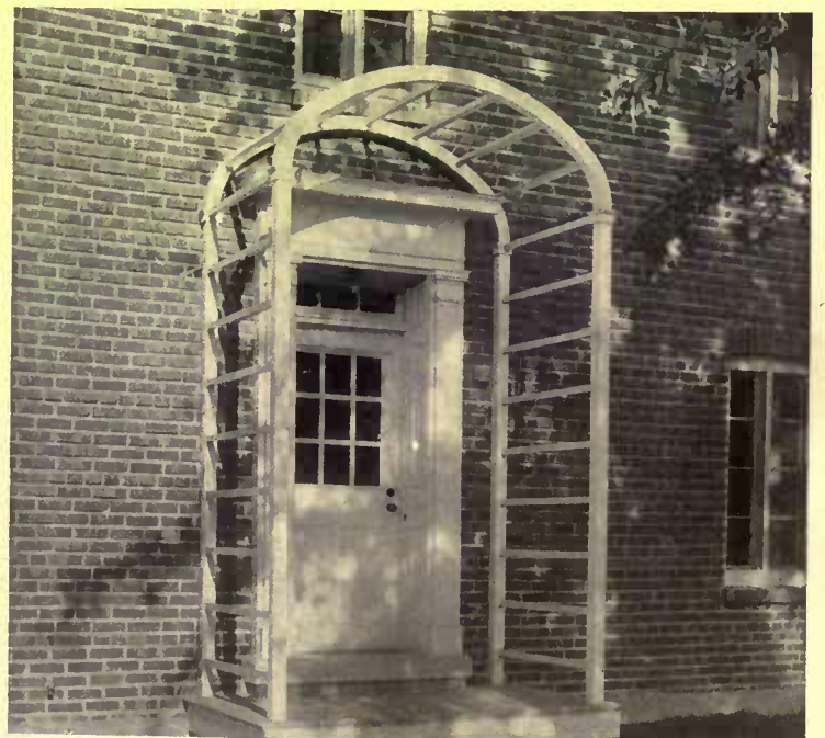
The light pottery colored brick with wide joints makes the wall surface appear large. The arbor will be covered with climbing roses
