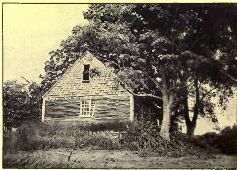
An old home at Gray, Me., that is interesting but really beyond recovery
