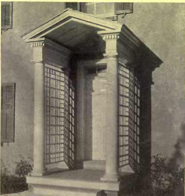
The stucco house has another adaptation of the Salem doorway. Both show different and appropriate uses of lattice
