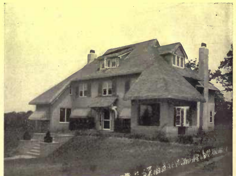
Although pleasing roof lines are obtained by use of shingles laid to imitate thatch, the cost of materials and labor is greatly increased. Albro & Lindeberg, architects
