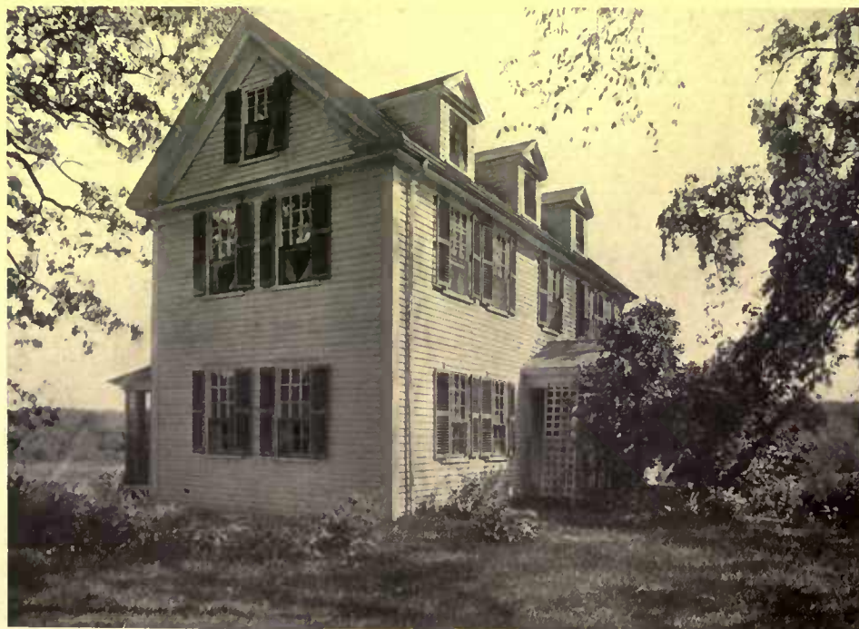
Dormer windows relieved a monotonous roof line and let in light to the apartments built in the unfinished attic space
