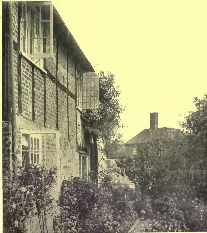
The casement window enables the entire window space to be open to light and air, and the hinged sash may often be used to direct air currents to the room
