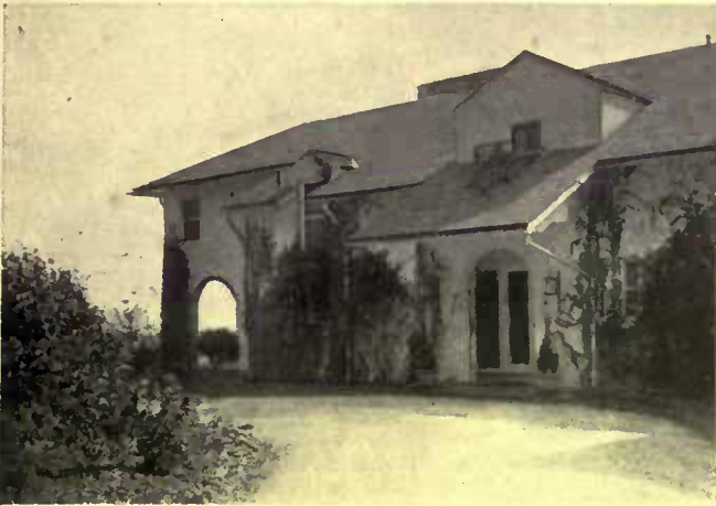
The entrance is away from the living side of the house and does not interfere with it
