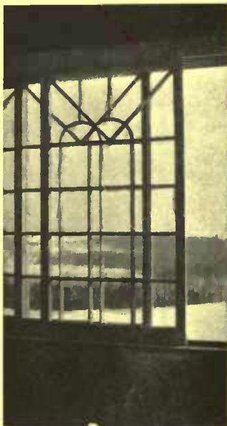
Adjustable sliding sash running in wooden grooves
