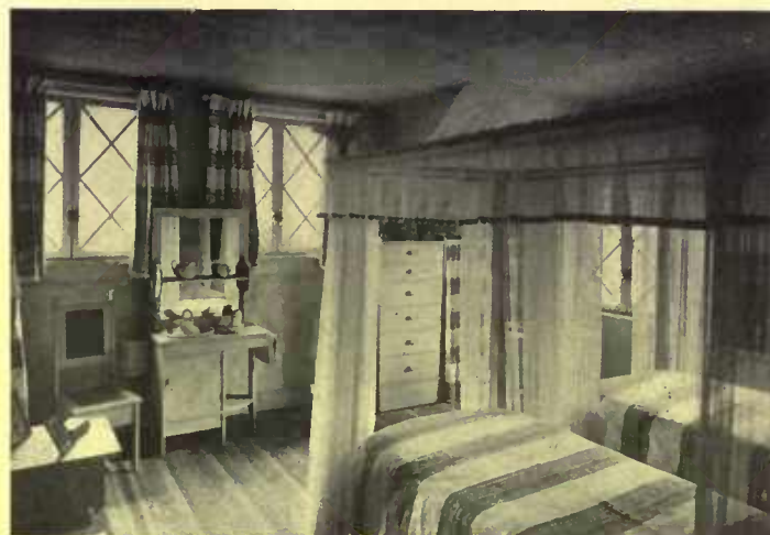
The furniture and fittings at Hukweem were left with the rough tool marks on them and were constructed entirely of native material from the estate
