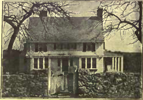
Residence at Newton, Mass., Finished with Old Virginia White. J. Lovell Little, Architect, Boston.
