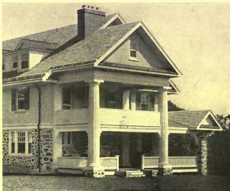
The portico with columns affords a logical place for the sleeping porch, in that it gives the appearance as well as the fact of adequate support
