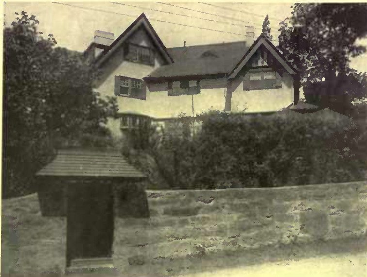
A good example of a wall of faced stones of irregular sizes and shapes, but well laid to harmonize with the style of building
