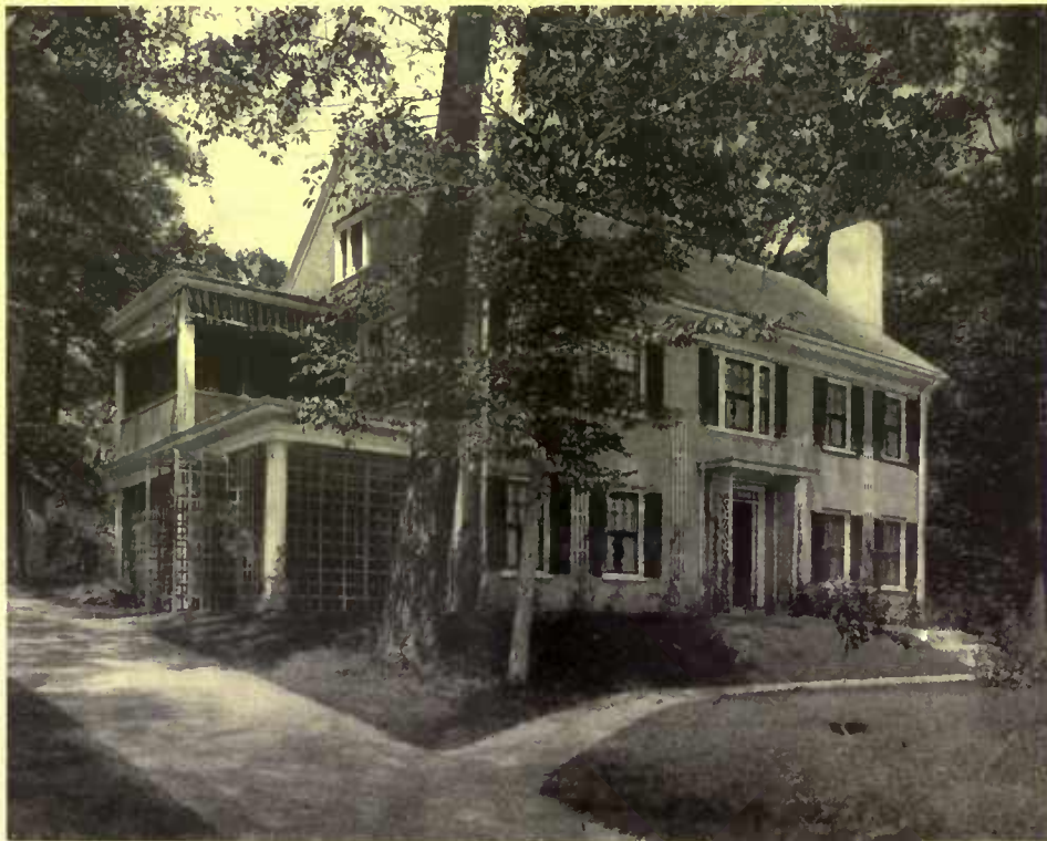
House No. 1 shows a moderate cost plan, with but one variation from the rectangular. It is a good example of an appropriate use of hollow tile and stucco in an unpretentious house, showing its adaptability to fit well into the situation. Putnam & Cox, architects
