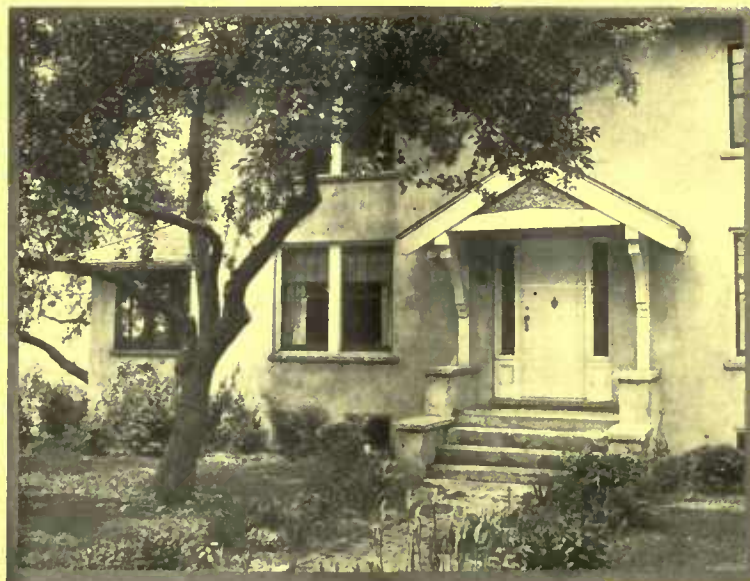
Although the general treatment is essentially simple, the entrance comes in for special attention with its dignified lines
