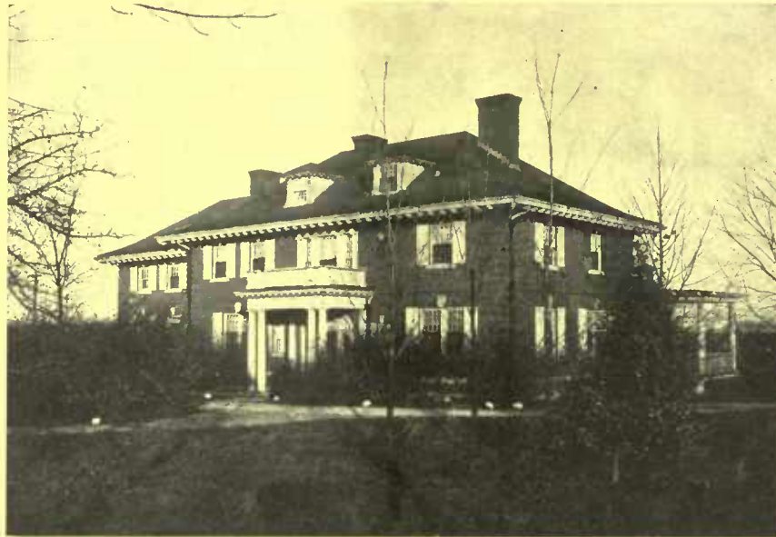
House No. 3 is of brick construction, built so as to produce the best fabric effect. James Purdon, architect
