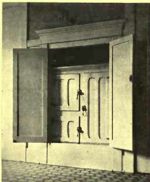
The cooling closet is located in a compartment in the kitchen and opens also on to the porch outside for the convenience of the ice man
