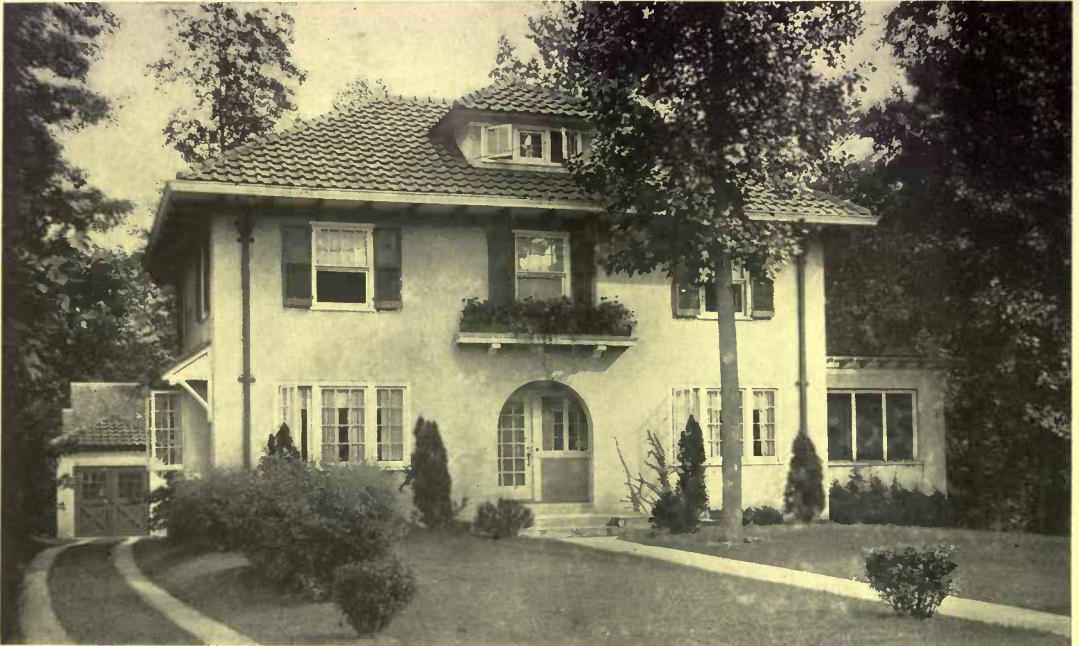
The front elevation of this house is devoid of all ornamentation, but the window box, the structural utilities, the copper leaders and the shutters are extremely decorative, and the impression of the whole is of pleasing interest. The grass-cement-bordered garage drive is worth emulation
