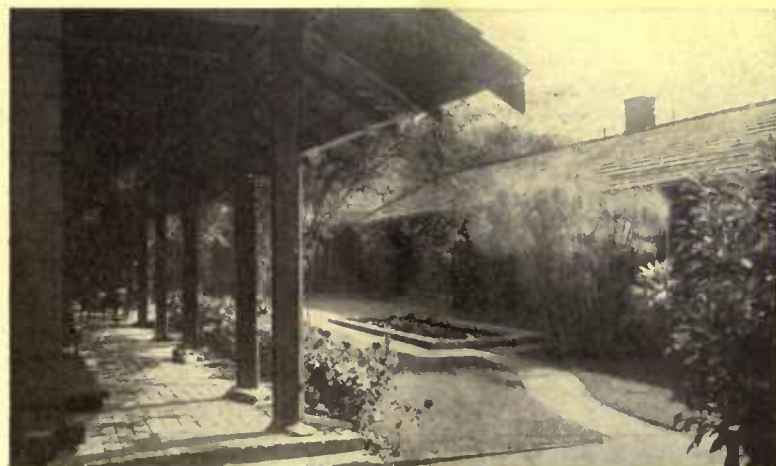
Perhaps one of the most effective plans is that of the inner court. It is a successful way to have cross ventilation in all rooms
