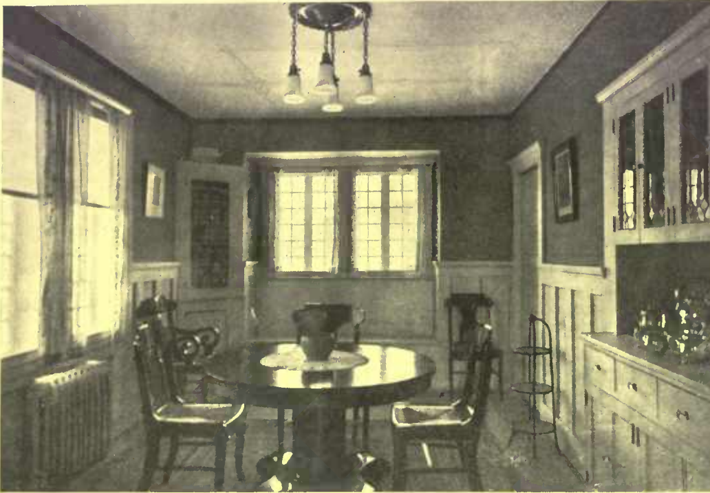
Electricity and steam heat are features of the successful bungalow. Here a saving was made by the use of plaster boards instead of lath and plaster
