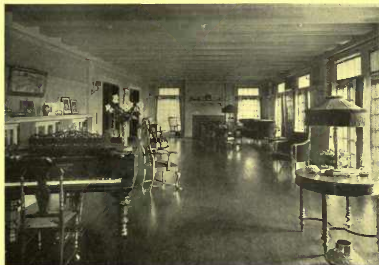
The great living-room is practically all windows on two sides and is planned so that it may be available for all sorts of entertainments
