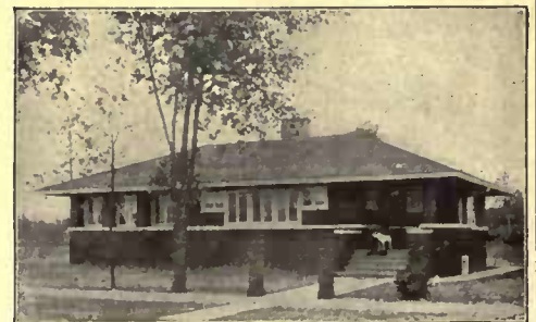
Stained with Cabot's Creosote Stains Sidney Lovell, Architect, Chicago, Ill.
