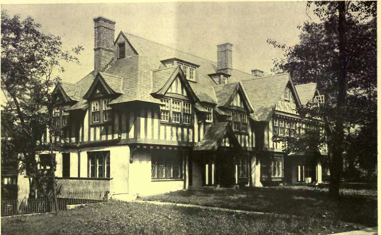
By a double house is meant a building that provides accommodations for two families, but when properly planned the life in each should be absolutely independent of the other. Though in close proximity, the piazzas or verandas should not look out upon each other
