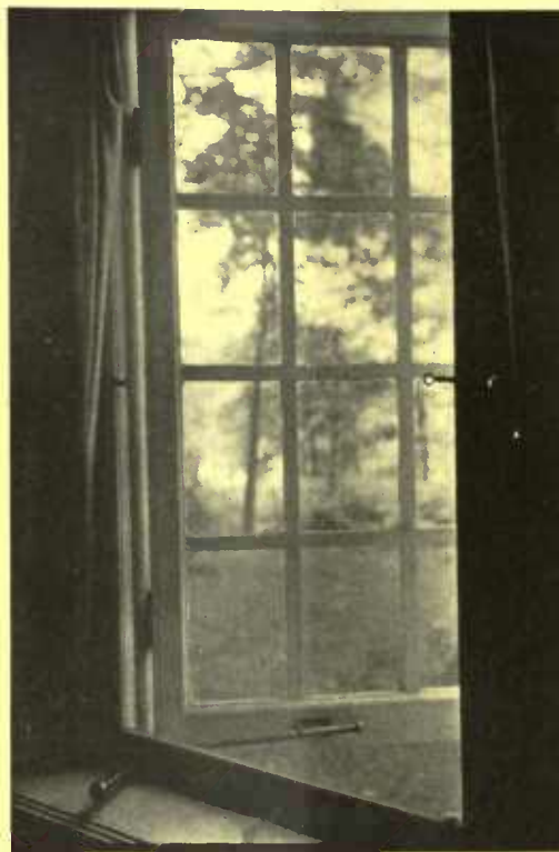
The lever on the inside of the screen, when moved either to the right or the left, opens or closes the window without interfering with the screen
