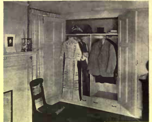
A convenience to almost every house is a built-in wardrobe equipped with a hanging device that keeps the clothes in condition and makes them easy to get at
