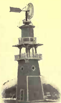
A Church Pneumatic Tank with Pumping Engine
