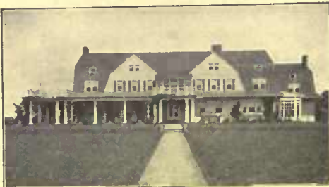
Residence of Ralph Peters, Esq., President Long Island R. R. Aymar Embury, II., Architect, New York Shingles stained with Cabot's Shingle Stains, stucco stained with Cabot's Waterproof Cement Stains, and lined with Cabot's Quilt for warmth
