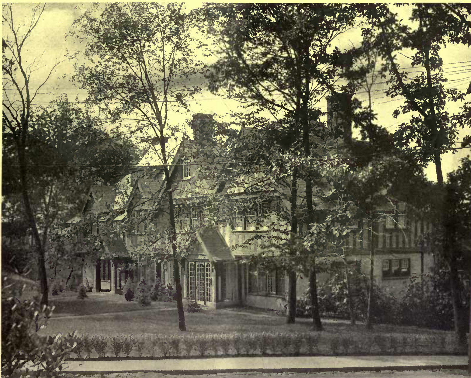
The architects have treated an interesting lot problem very cleverly. The drop of the lawn is not only from the front of the house to the back, but the property has also a longitudinal slope. These differences suggested the double house, and it worked out exceedingly well in providing large rooms and making the life of both places independent, one house from the other
