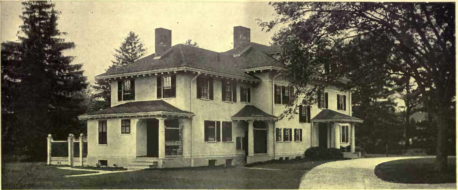
House No. 2 has a wood frame and is over wire lath. The photograph here shows an interesting effect of the architect's planning to create a unified effect in a rectangular house. It will be noticed that the three doorways are treated almost exactly the same and have the effect of the repetition of a unit design. Although the house is large it is compact. George Hunt Ingraham, architect
