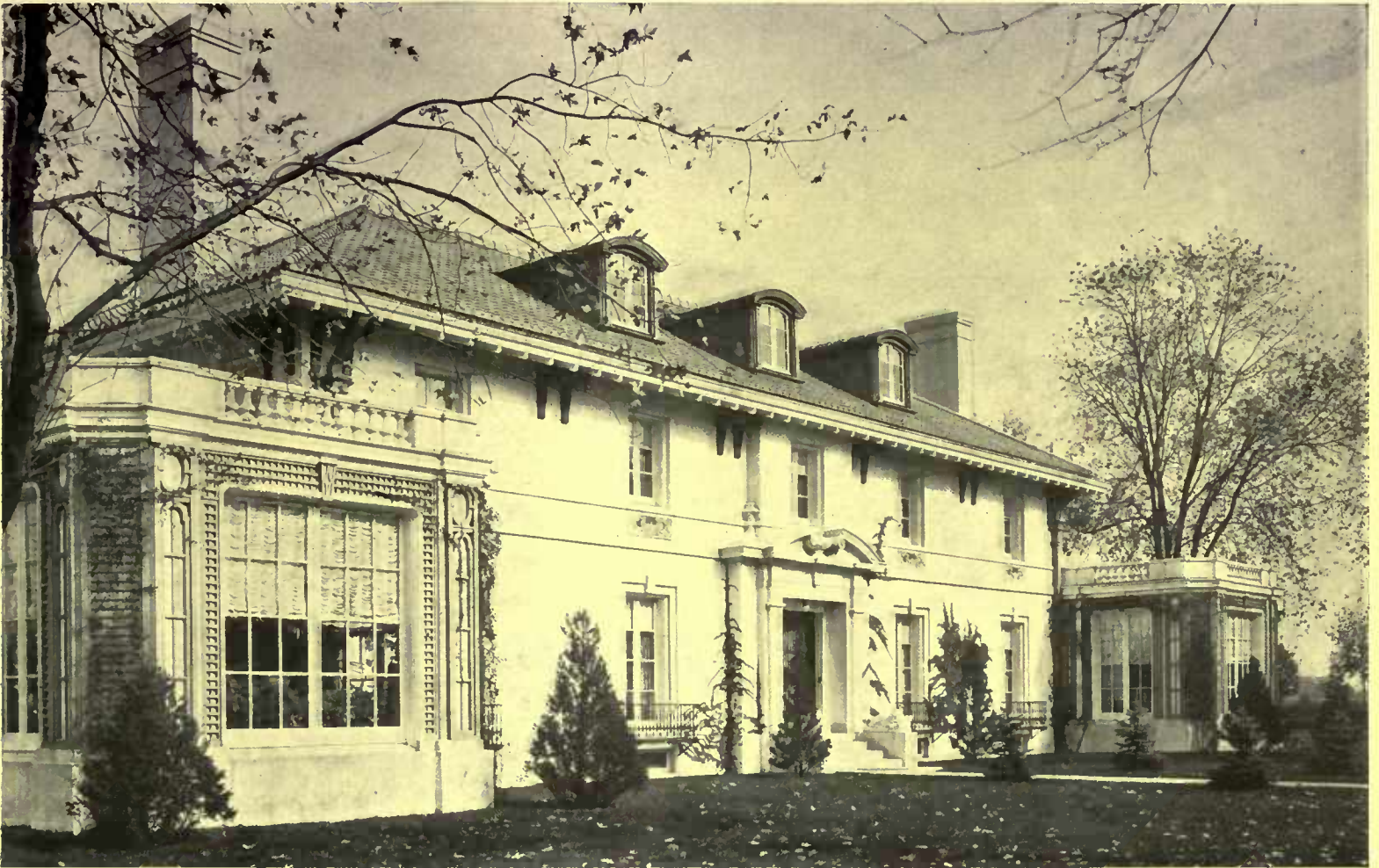
There are a number of sources of decoration in this façade used with an exceedingly fine sense of color and proportion and productive of a rich dignity. The loggia of this sort is supplanting the columned porch, its services are greater
