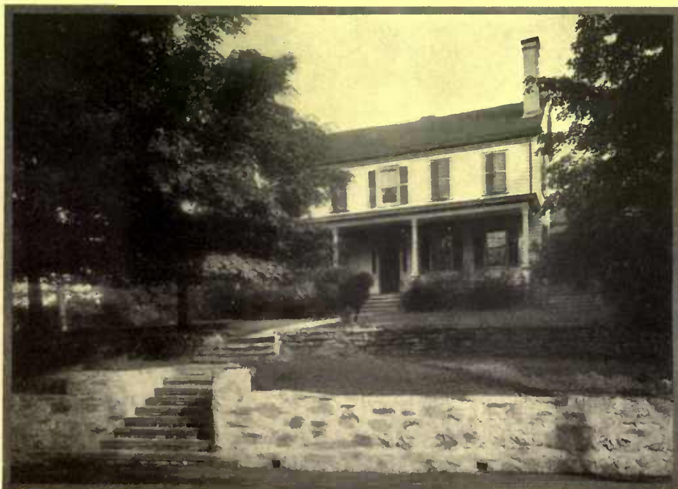
Two terraces, faced with stone, break the slope of the ground between the entrance porch and the road, giving pleasantly harmonious lines to a situation which otherwise might have been monotonous
