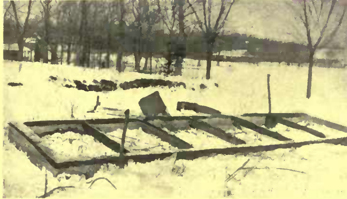
Frames made of cement are impervious to moisture and will last for years
