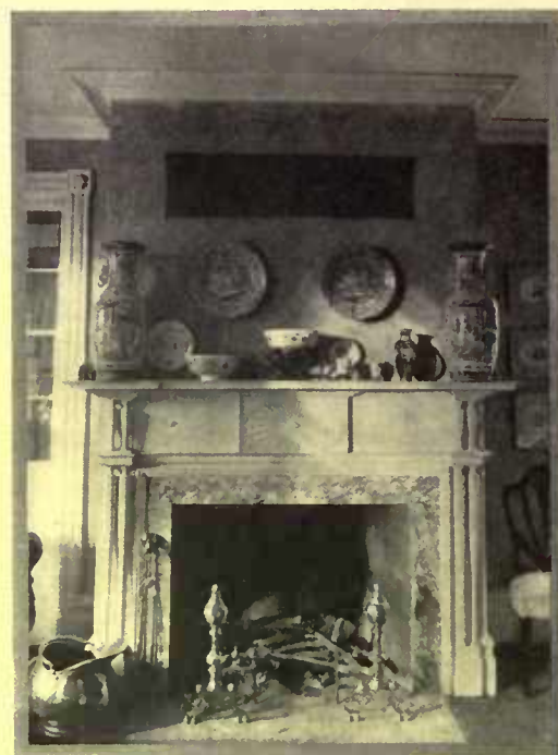
From beneath the kitchen stove were unearthed the marble slabs that once framed the fireplace opening
