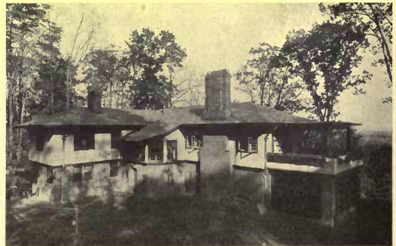
The entire stair space is taken up by the little section at the junction of the two wings; the house proper is devoted entirely to room space
