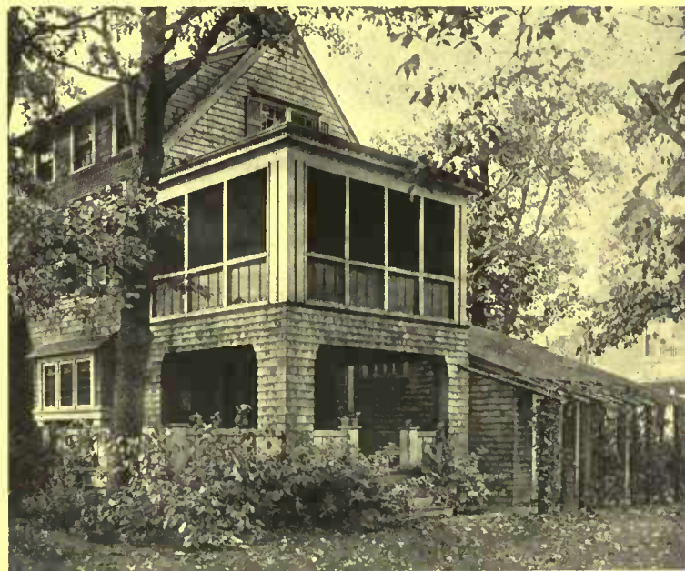
Although rather too prominent in this instance, the sleeping porch over the entrance is usually a satisfactory means of solving the problem
