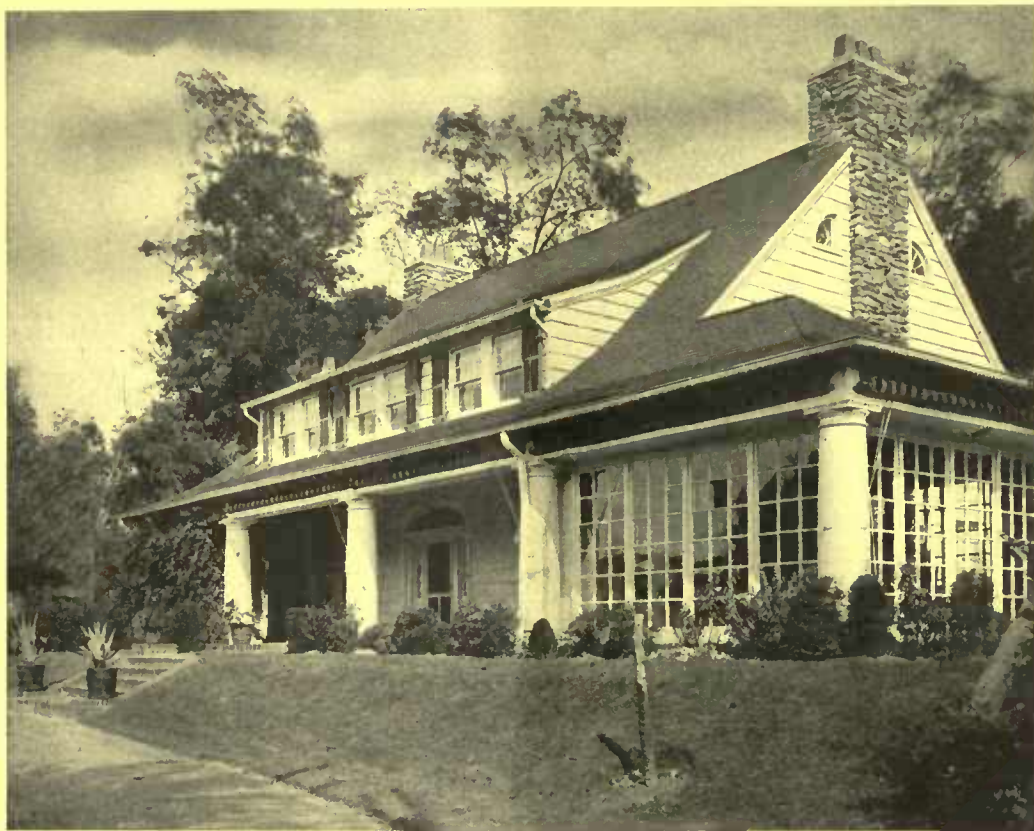
Shingles are most appropriate to a style of house popular in America, and sometimes called the farmhouse type. When laid in wide courses and painted white, with green trimmings, the result is decidedly attractive. Bates & How, architects
