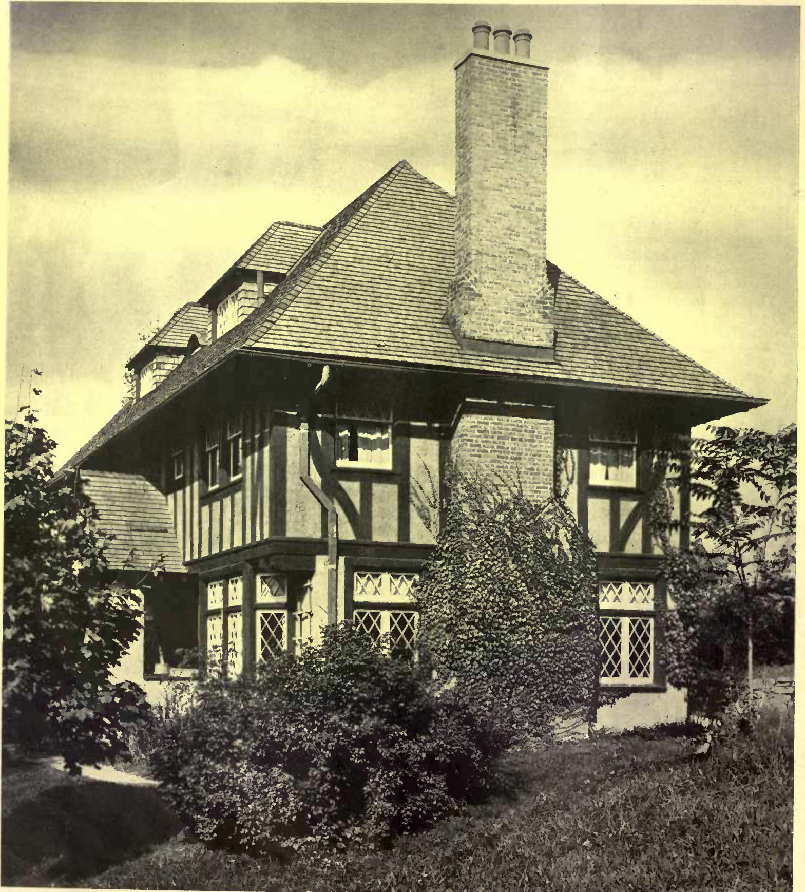
There is a characteristic about this small house that is striven for by many house builders—it really gives the impression of homelikeness. What is more, it is good half-timber work, the woodwork giving the impression of stability and appearing to be structural. Stucco of creamy tint combines well with the browns of the timbers and the roof. The diamond-paned casements add further interest to the whole
