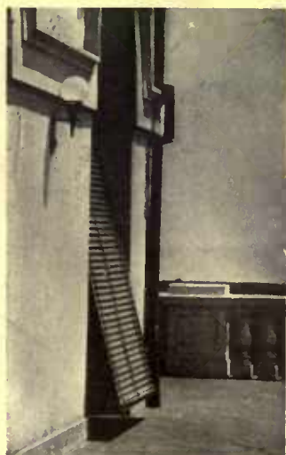
A useful Venetian blind that is both shade and awning gives ventilation without letting in the rain
