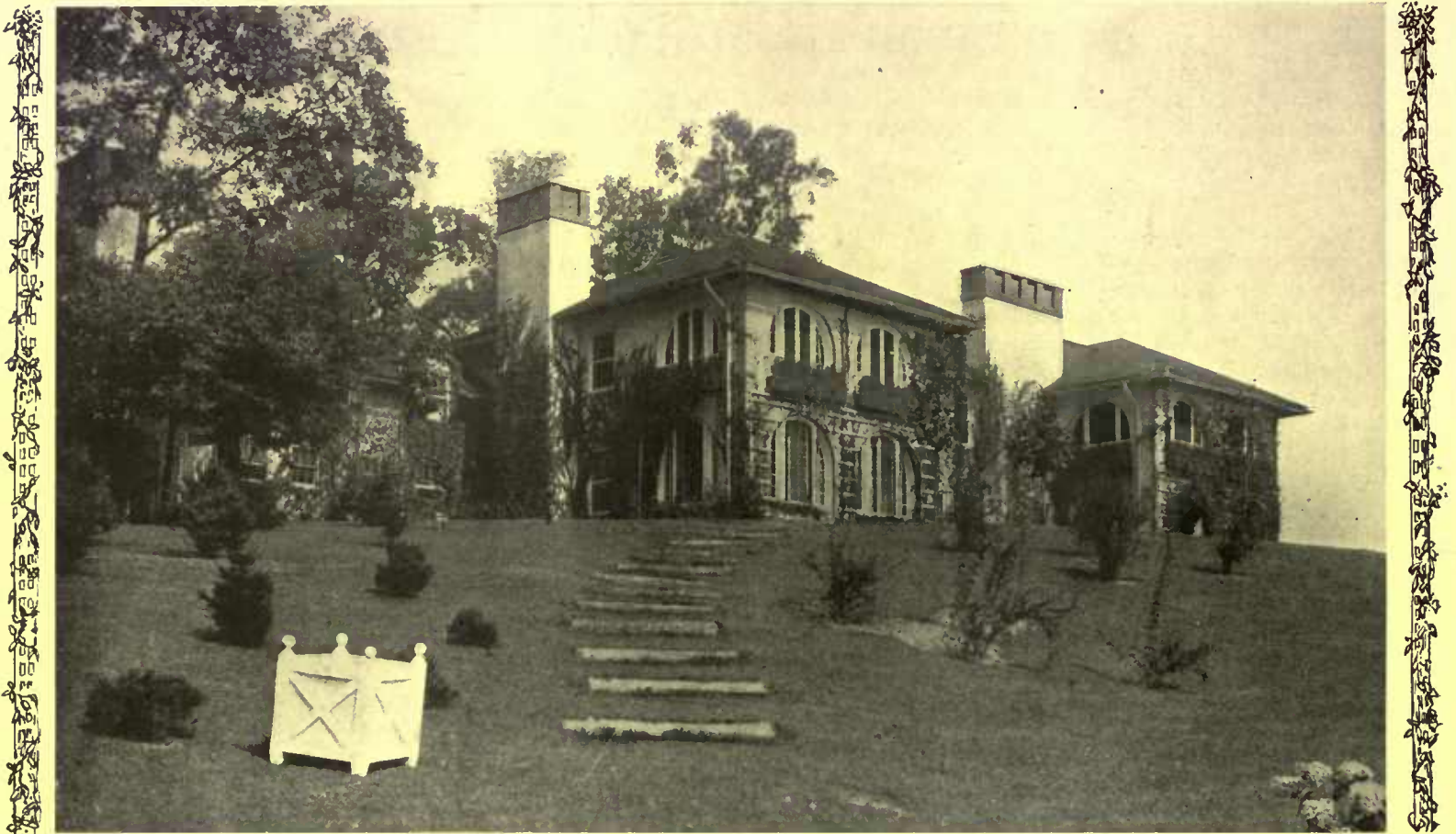
Mr. McGinley's house boasts that desired situation, a hilltop site, but it is distinctive in being so planned that it hugs the ground close instead of rearing monument-like into the sky
