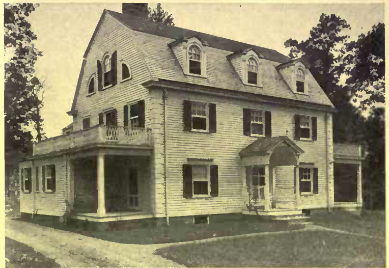
A Colonial house of clapboards that follows the old precedent. Clapboards are especially fitted for designs such as this. Hays & Hoadley, architects
