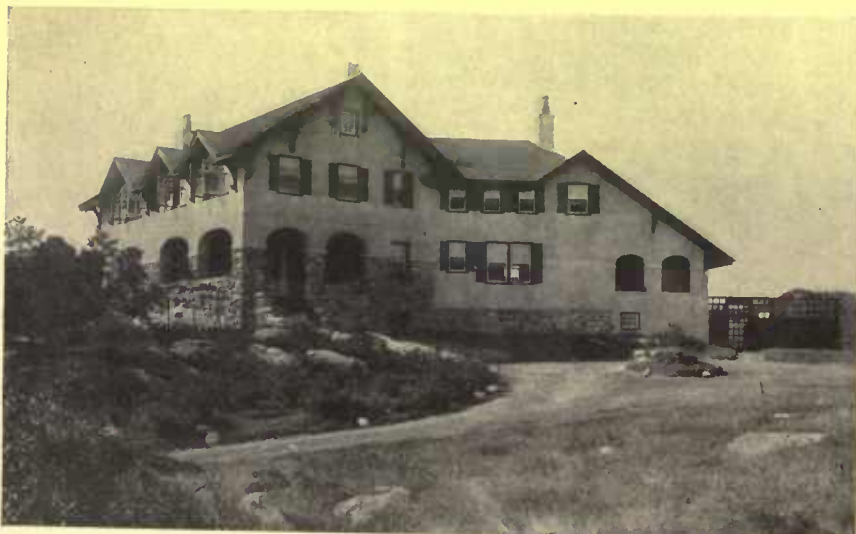
The successful house will partake of the nature of its surroundings. This is made possible, as in this instance, by the use of a foundation of native stone
