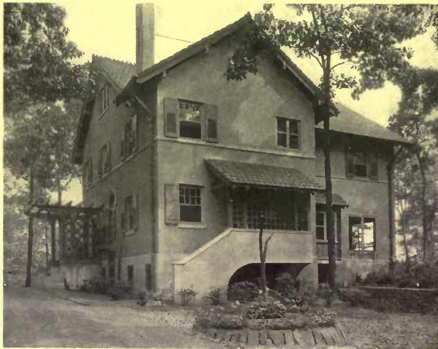
Sloping ground increases the cost of foundations, but gives light to basement rooms, and here provides enough extra space to be used for a garage beneath the dining-room
