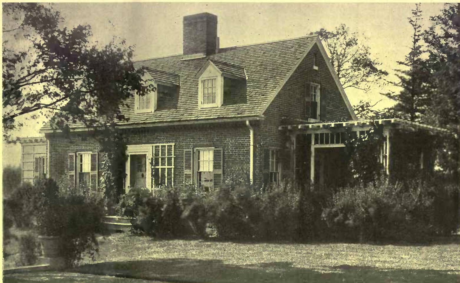
One way to attain coolness is by insulation. There should be air space under the roof and an insulation between the roof and the upper chambers. Brick and hollow tile walls provide cool interiors
