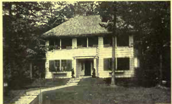
A house practical, livable and attractive for a suburban lot Frank C. Brown, architect
