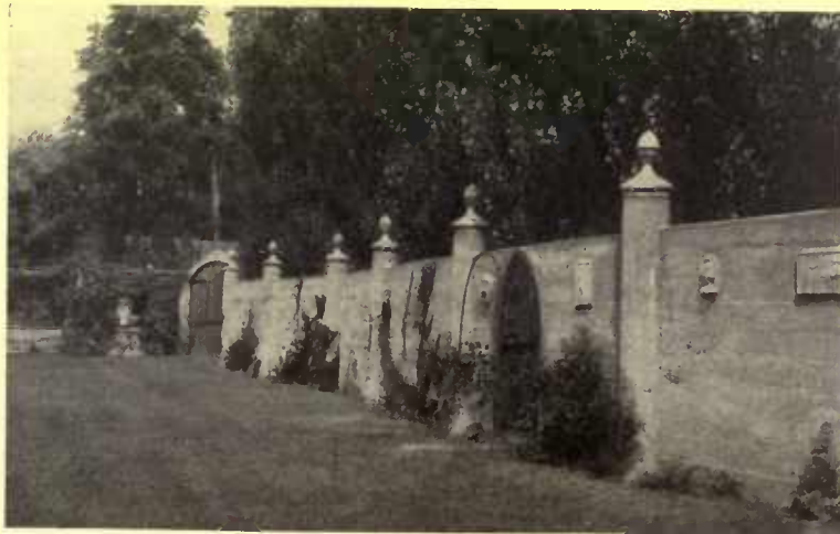
This concrete fence is built in forms and is reinforced with steel uprights. The ornament is also of concrete cast in molds. A slightly roughed surface gives a texture effect
