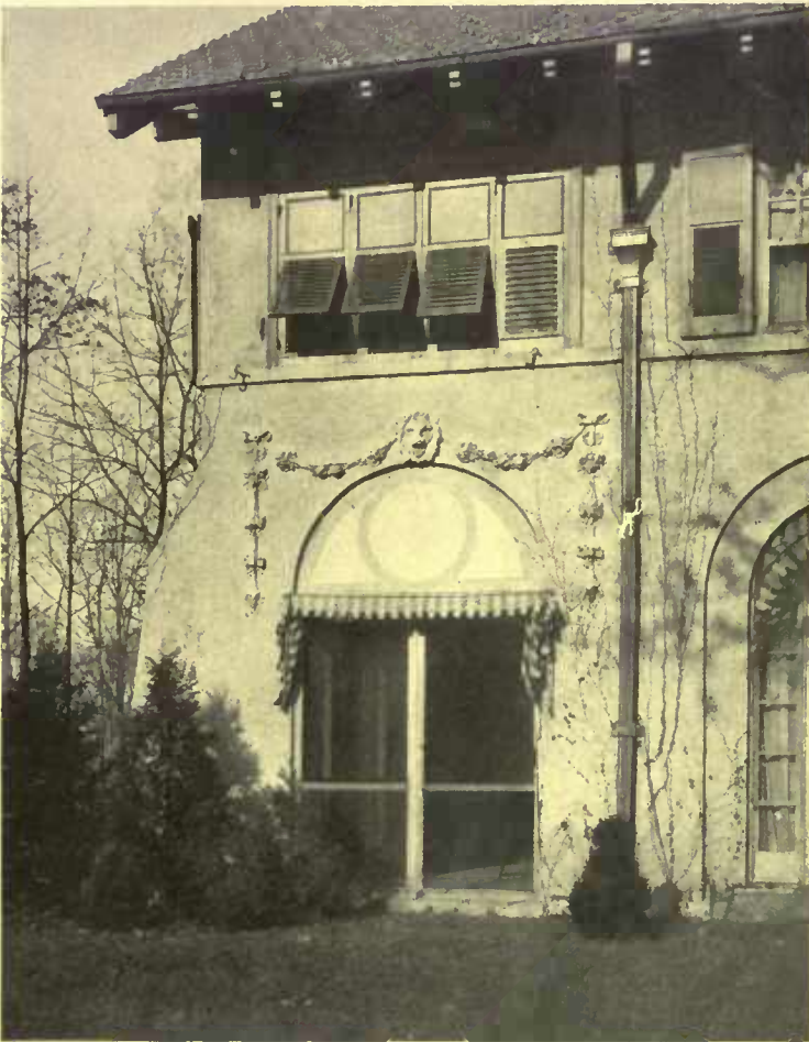
There is a considerable decorative quality in the window disposal, which does not conflict with utility. Such shutters have the added value of awnings
