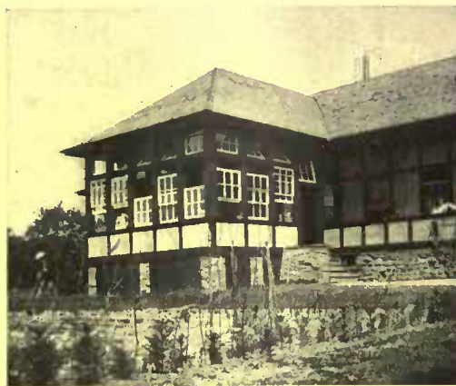
The entire wing of this cottage is devoted to outdoor sleeping. The enclosures are of the ordinary double-sash type, with transoms above
