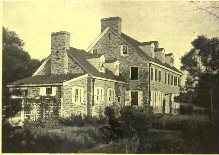
Your choice of material depends largely upon the material found in the neighborhood. An attractive fieldstone house of the Philadelphia type
