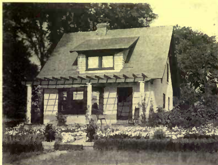
The building material chosen was hollow tile, with a white rough finish and brown trim. The brick-paved pergola was to tie the house to its garden
