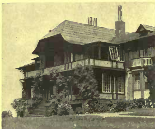
A central porch showing a pleasing treatment. The sash enclosures at the side are of the cellar type illustrated in detail below
