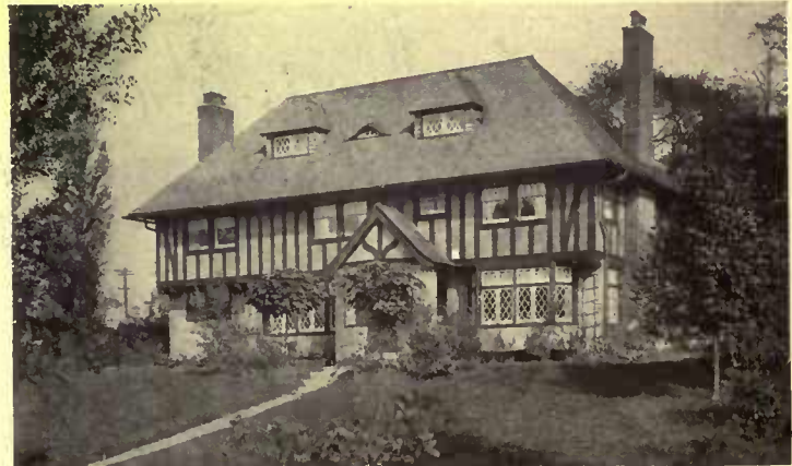
Half-timber modified to our needs, loses no charm. Mann & MacNeille, architects
