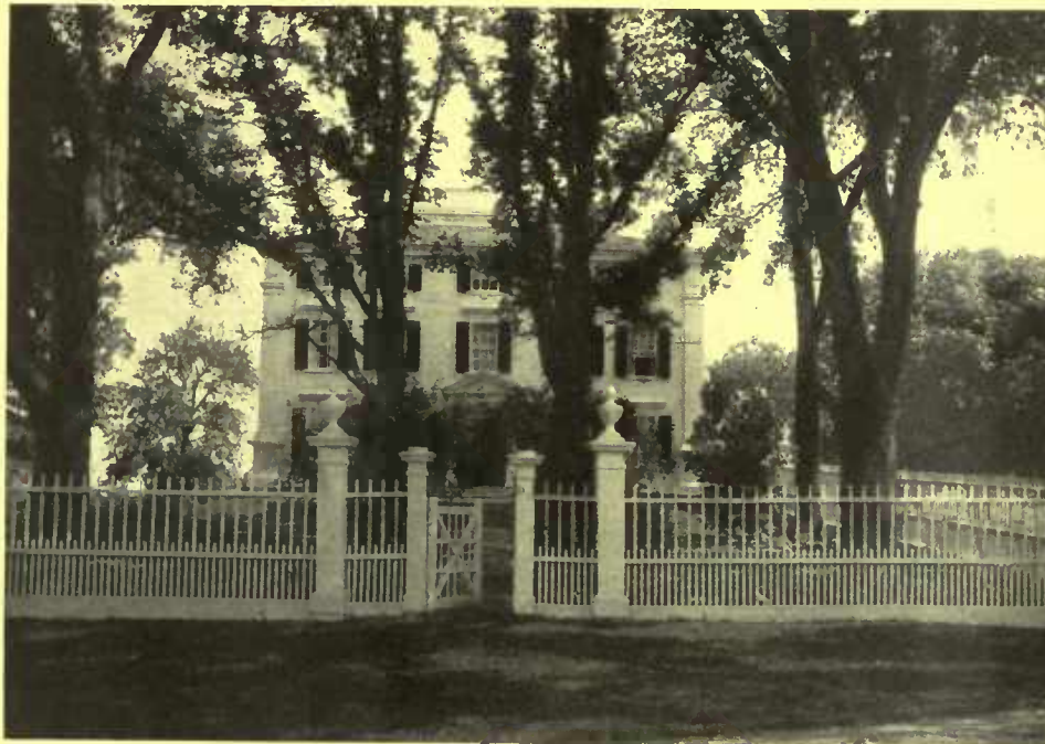
In excellent keeping is this fence of Colonial motif. The square pickets rest on an impregnated wood base and pass through holes in the rails; the double row of short members lends attractiveness to the design
