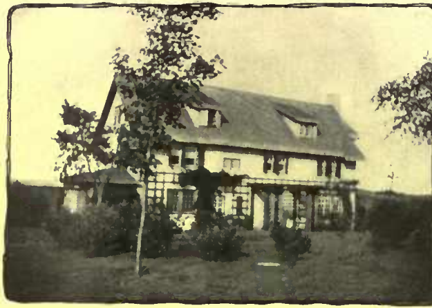
When we look back at the building of the house, we recall the first thrill of completed endeavor
