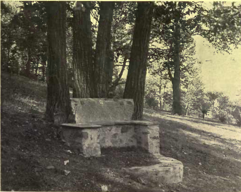
A little cement, some waste slate slabs and the litter of stone work makes "the wishing chair" that commands a magnificent view of the whole garden
