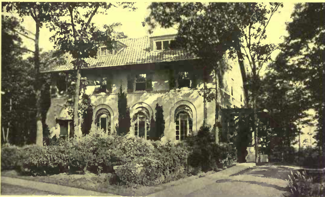
Stucco on hollow tile is really a flexible building material. That one need not resort to the use of exterior wall decoration of other materials to produce a beautiful home, is proved by this house, the home of Mr. Perry MacNeille. Mann & MacNeille, architects
