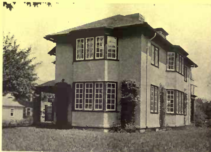
This house was constructed in the manner shown above and demonstrates the prominence of such materials after weathering. A. A. Thayer, architect
