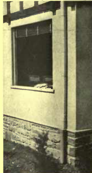
Large windows protected by durable Venetian blinds
