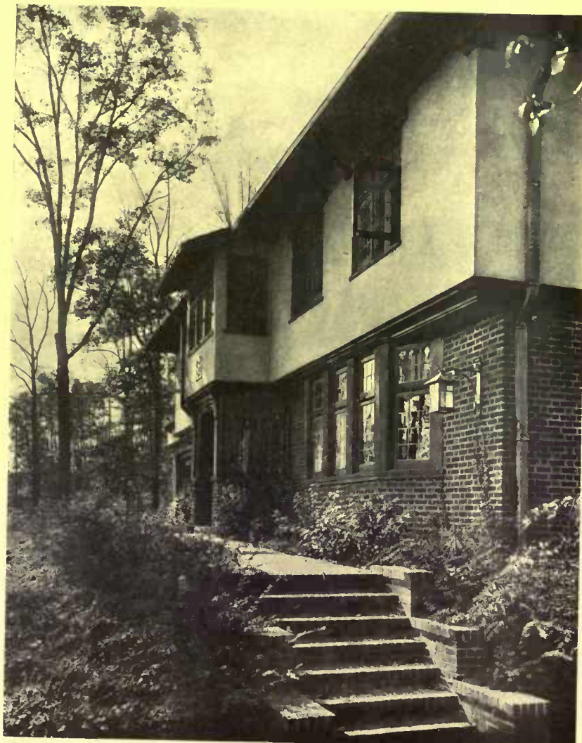
The architects are strong believers in the casement window and they have well mastered its difficulties. Small units are used and grouped with mullions between. If a casement window is not over two and a half feet wide, it may be made weatherproof
