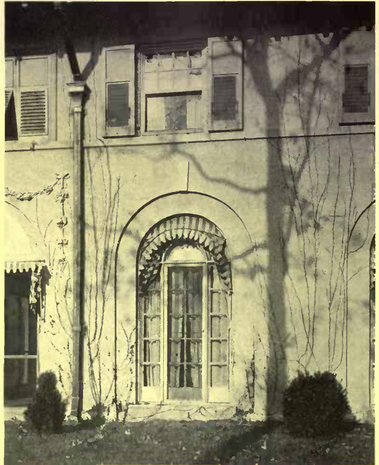
Recessed tympanum arches in the doorways and lower windows give a simple decorative quality in their shadow lines. The architectural ornament is well chosen also
