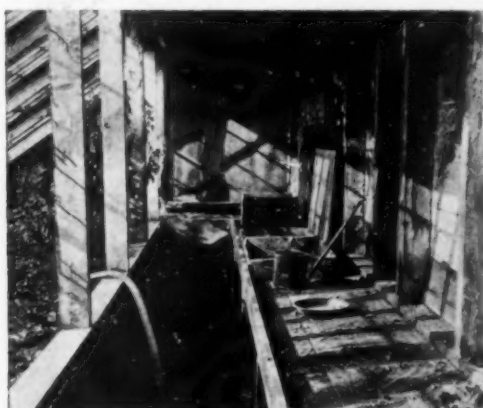
Glass-fronted workroom built against the south wall of out-buildings
