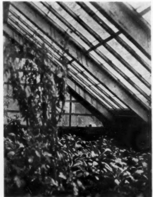
The sashes are set at an acute angle to catch the sun's rays
