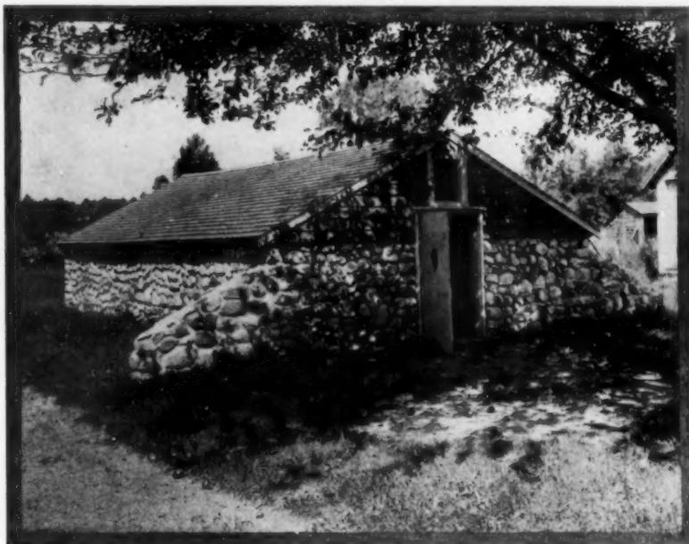
On a large place an incubator cellar will be found more practical, centering the work in one place and avoiding the possibility of a fire in the house
