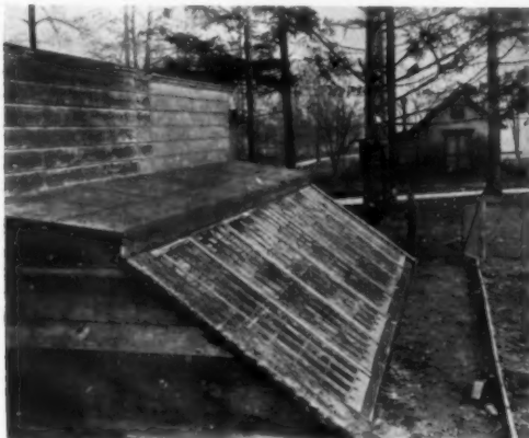
The roof is covered with tar paper and slants enough to shed rain
