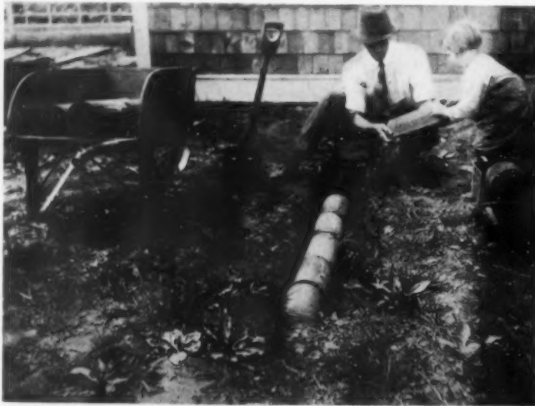
To determine the water table height, the bottom of the drain should start a foot below soil level. Note the sub-surface water level. This seepage should be run off to avoid sogginess.
