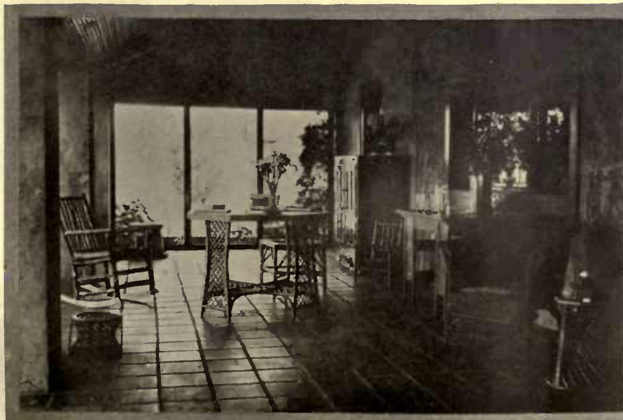
On the floor of the living-porch are square red tiles laid in wide gray bond, with here and there a Grueby for variety
