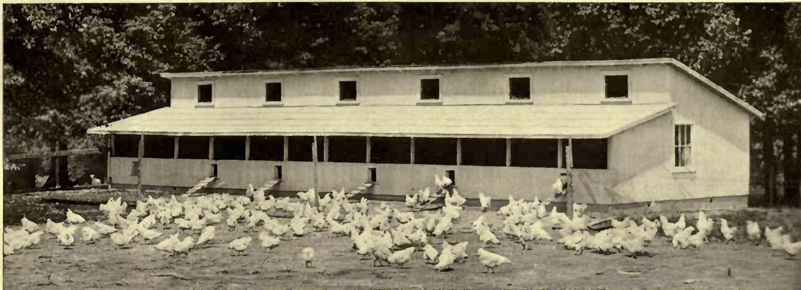
Although somewhat elaborately constructed, the semi-monitor type is excellent for cold climates because it is deep and yet well lighted
