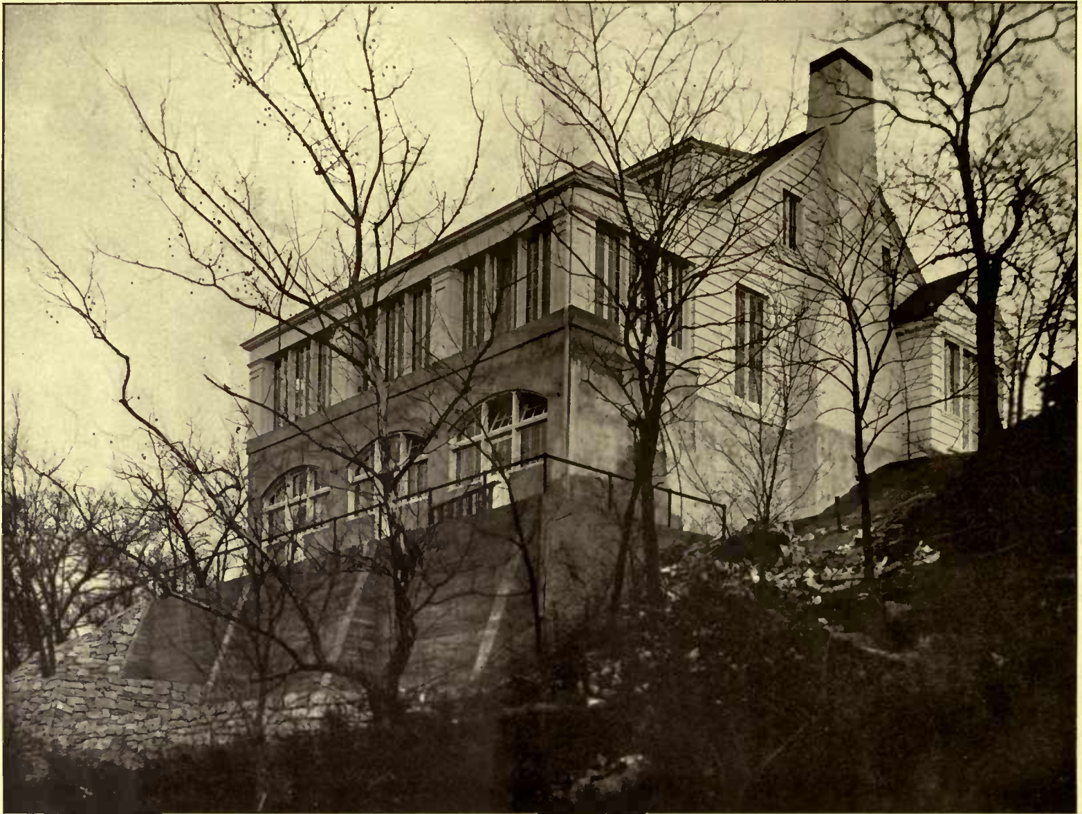
The main factor in construction expense was shoring up the foundations, as the lot was on the edge of a steep hillside. It gave, however, a diversity of levels to the rooms and added interest to the interior
