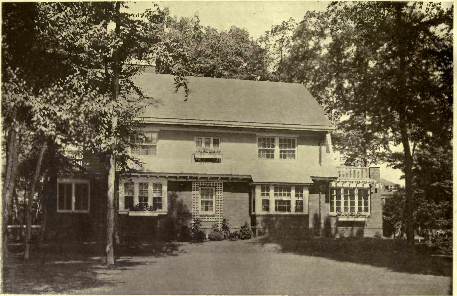
The outside walls are constructed of hollow-tile blocks, faced with brick laid up in Dutch bond in the first story; with stucco in the second and on the gable walls of the attic. The foundation walls are of concrete, water-proofed on the outside, with a tile dry drain all around
