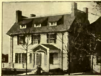
Walter Baschen, Architect, St. Joseph, Mo. Walls finished with Cabot's Old Virginia White. Roof finished with No. 346 Dark Gray Creosote Stain.
