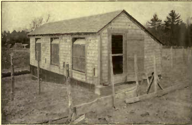
Houses of the semi-monitor type have a double pitch roof, but the rear slope is high enough to allow a row of windows. Such a foundation will exclude rats
