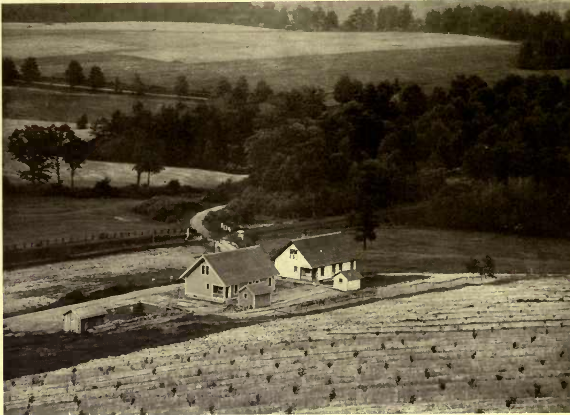
The bungalows for the farm hands were situated near the main road, the first serving as a lodge. Two were built and the foundations laid for a third. Complete cost, $4,775.41
