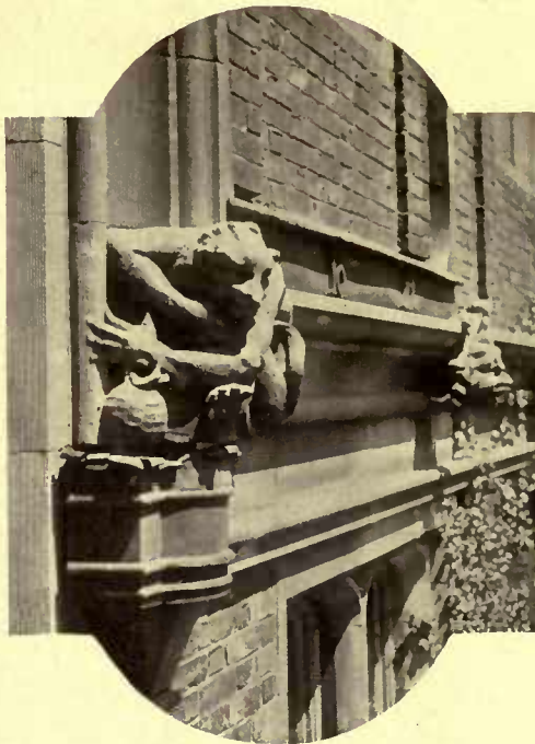
The rain-water head can be successfully used in conjunction with a gargoyle or grotesque
