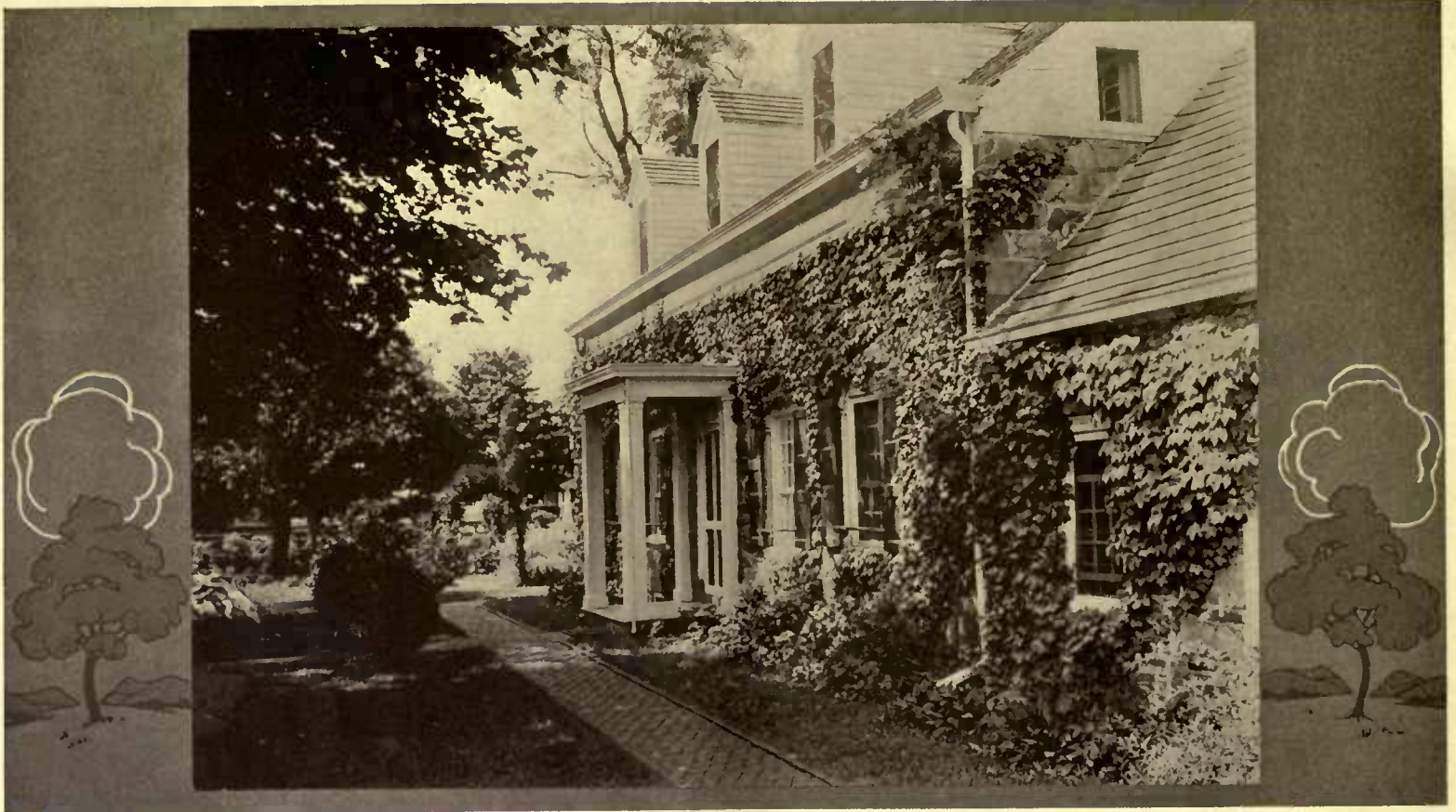
The house stands to-day much as it stood in 1788, save that in restoring dormers were added, a wide, comfortable porch built on the side and back, and a trellised entrance placed at the kitchen end
