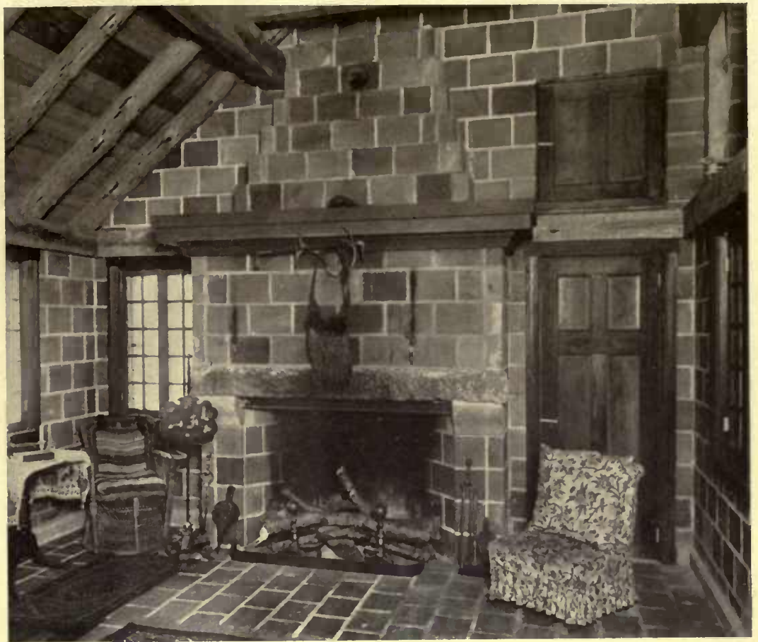
A novel treatment fitting for a room of this type—hollow tile walls and floor laid in wide bonding. It shows also the foundation for plastered or paneled walls in hollow tile houses
