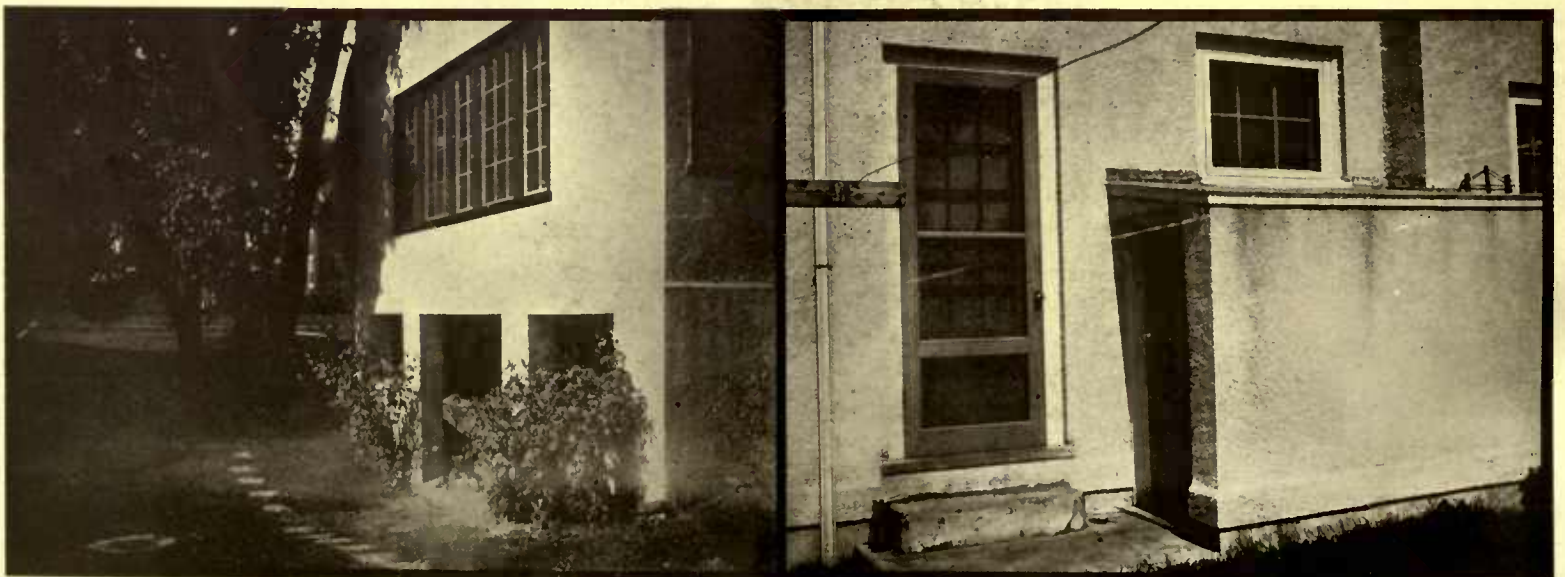
A recessed entrance of this type is decorative, unusual and practical, save that the open space between the pillars is apt to become filled with drifted leaves and paper
