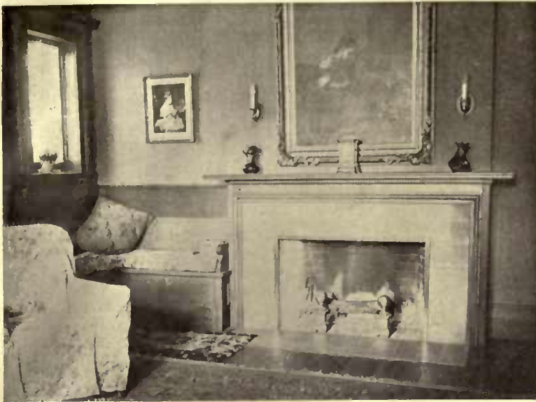
The fireplace of the living-room is faced with dull brown tile, with a brass moulding, the whole blending with the finish of the oak trim
