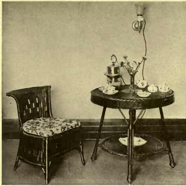
On the fixture is a current-top attachment by means of which any portable electric device may be connected without cutting off the light
