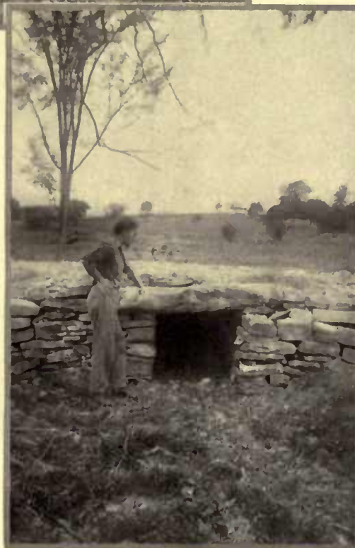
Meadow rivulets are lively creeks in the spring, hence the culverts with heavy stone caps
