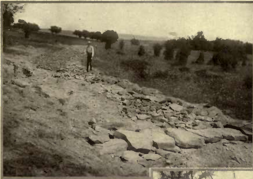
In the hollows the road was built high above the field—a mile of it
