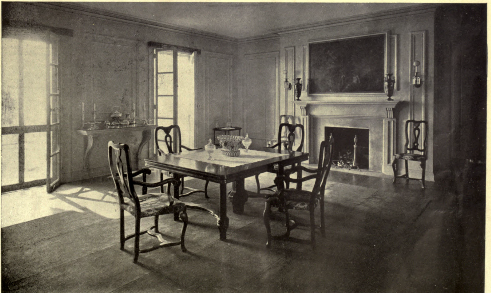
Simplicity in construction and decoration obtains throughout the house. On the first floor walls remarkably decorative panels are made by simply nailing moulding to the plaster; the floors are oak laid in plain strips. The entire interior is painted a neutral grey
