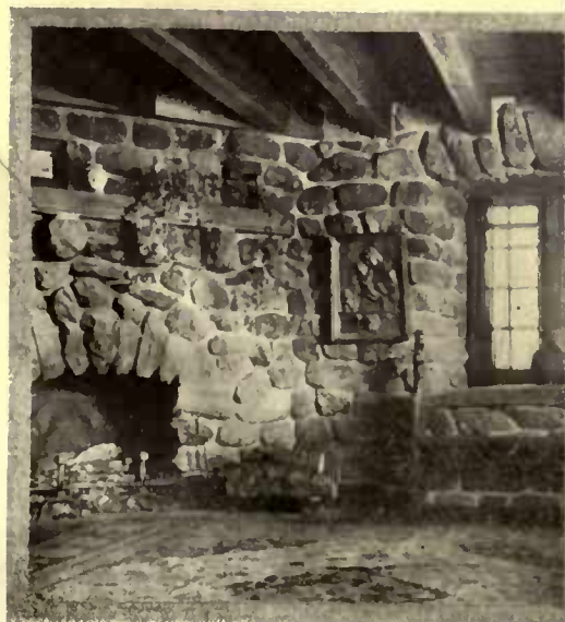
This carries the glimpse of the living-room farther along, showing the massiveness of the masonry and the airy spaciousness of the beamed ceiling
