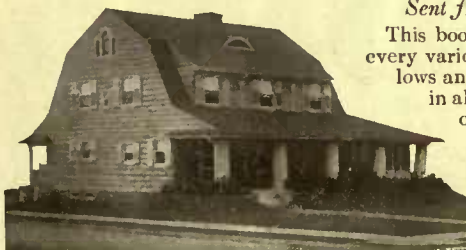
Stained with Cabot's Creosote Stains Charles M. Sutton, Architect, New York
