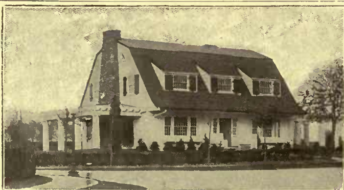
Stained with Cabot's Shingle Stains Forman & Light, Architects, 40 Cedar Street, New York
