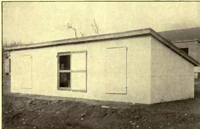
Stucco board cuts the cost of construction at least 10 per cent. This material, which comes in squares and is nailed to the frame, is rapidly growing in popularity
