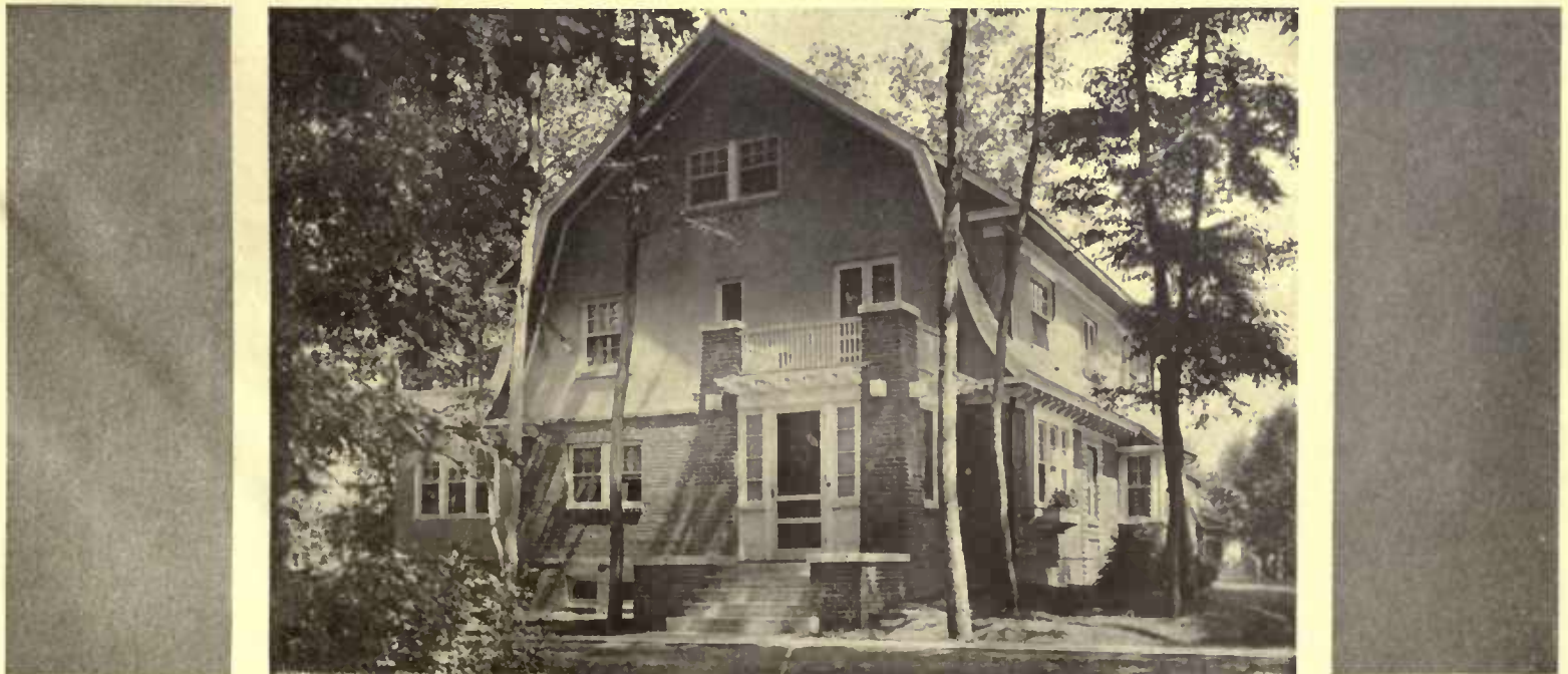
The end elevation shows the generous service quarters, which include a servant's alcove at the rear. In the cellar beside the heating apparatus is the laundry, a vacuum cleaning pump and, under the sun room, a "Trinkstule," trimmed in cypress, with wainscoting, amber colored leaded glass windows and plaster finish
