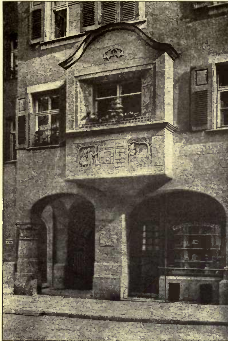
A combination of various materials has been used to excellent advantage on the buildings facing the Geiss-Strasse, ground floors mainly of stone, the upper of stucco. On this façade is a stone oriel, illustrating the tale of Hansel and Gretel
