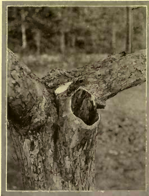
Cut off the small branches surrounding the stump and see that the decayed edges are cut away
