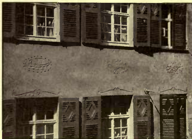
Sgraffito ornament in browns, greys and yellows, are used on all the buildings. The shutters are carved with decorative designs and painted a dark green
