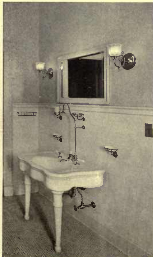
Arrange to have lights on each side of the mirror in the bathroom
