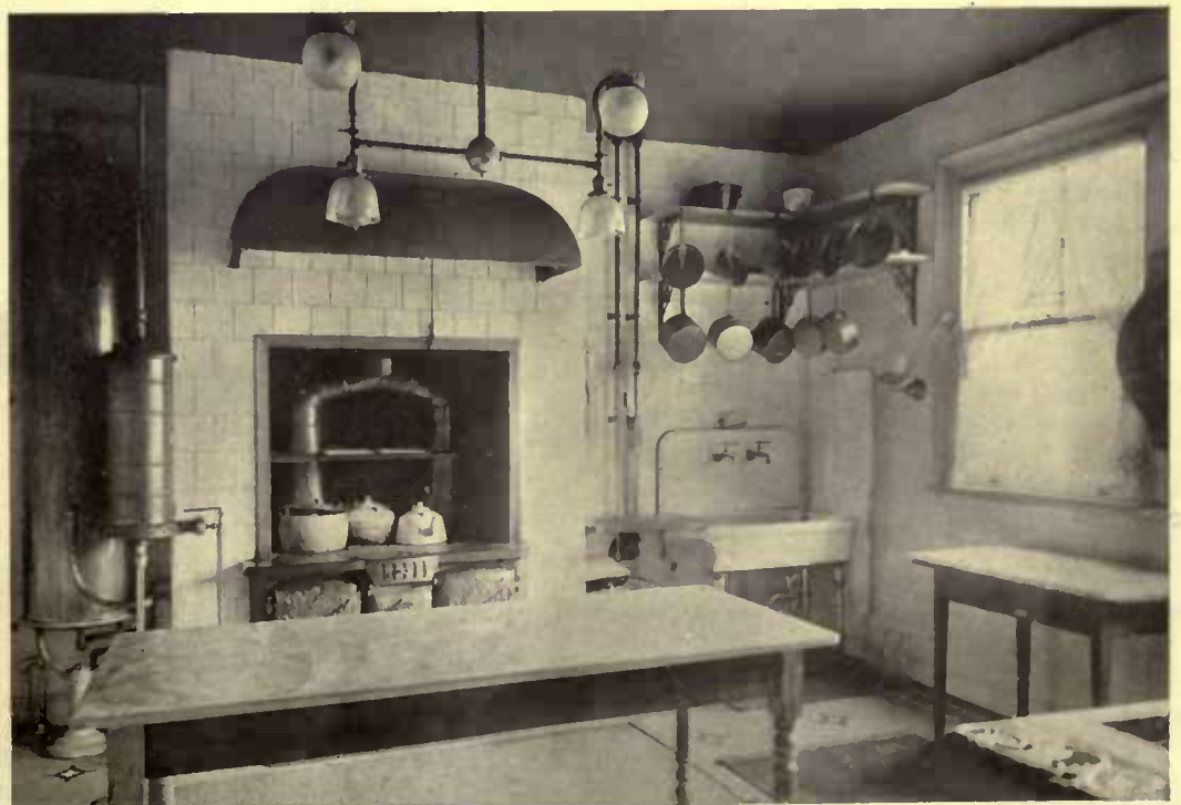
For kitchens, laundries and bathrooms glazed tile is the best treatment. Have the tiles set close together to avoid any roughness from cement joints. The cost is not necessarily prohibitive
