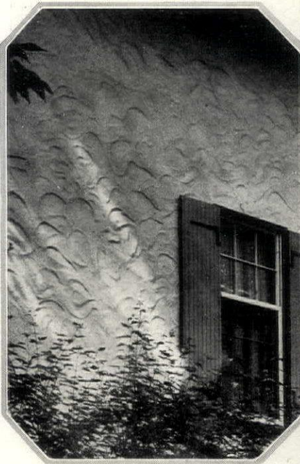
Because stucco is a plastic material, applied with a trowel, there is considerable latitude in the degree of texture which it may assume
