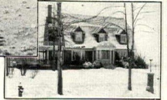
Residence at Westfield, New Jersey. Exterior of Redwood shingles and siding.
