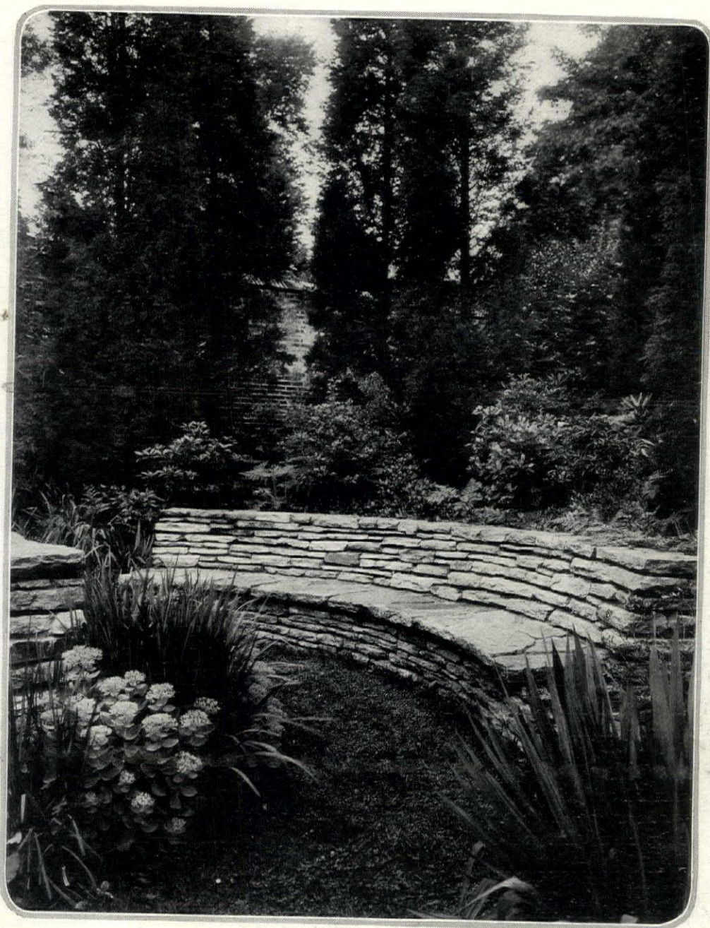
An unusually fine masonry seat and retaining wall combined designed for a Greenwich, Ct., garden. Ellen Shipman, landscape architect
