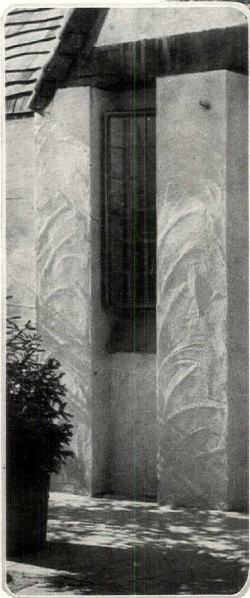
Texture in rough stone work in which the mortar is nearly as prominent as the stone
