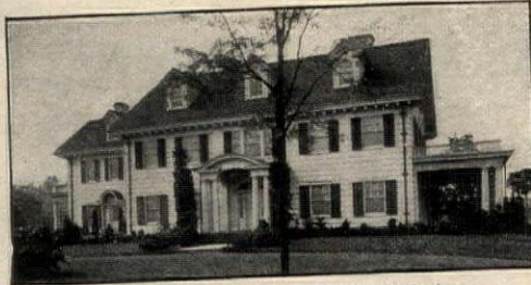
Stained with Cabot's Creosote Shingle Stains. C. M. Hart, Architect, Bay Shore, N. Y.
