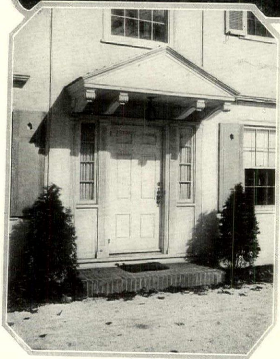
The treatment of the entrance front, with its tall pilasters and omission of the usual eaves, is unusual and effective, adding classic dignity without destroying the simplicity of the house. The hooded door is consistently designed
