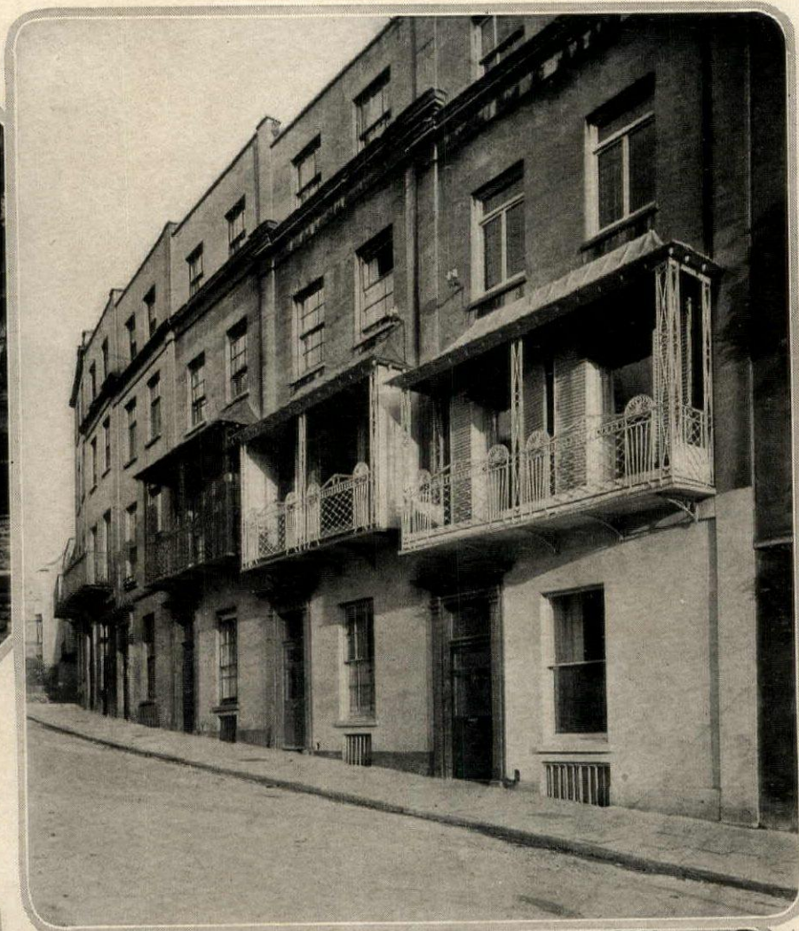
Roofed balconies with wrought iron in a great diversity of patterns were one of the most fascinating characteristics of the Regency period. Apart from their usefulness they proved to be an economical method of giving decoration
