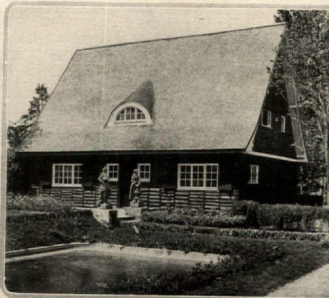
A model wooden country house of the north German style, with high-pitched roof and with log-faced walls
