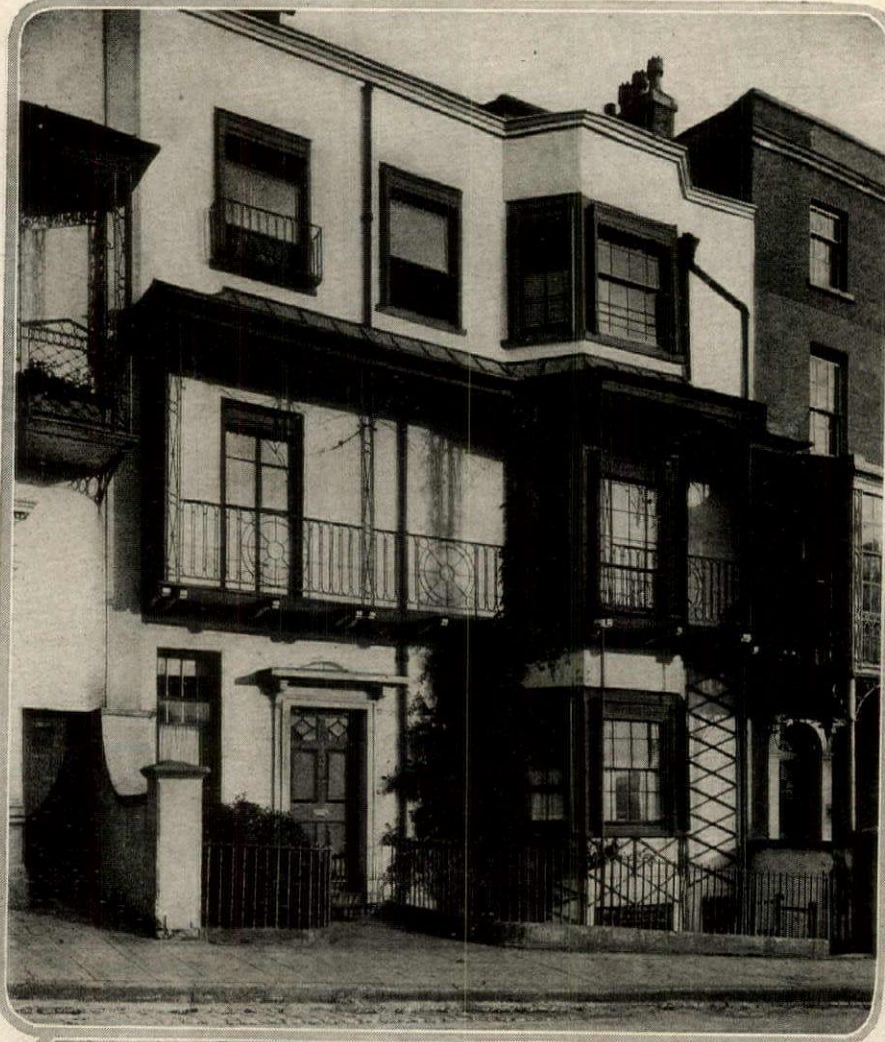
These balconies of Regency houses at Clifton, England, are so contrived that neither their floor projections nor roofs darken any of the windows. The attenuated pattern of the wrought iron accords with the spirit of design of the period
