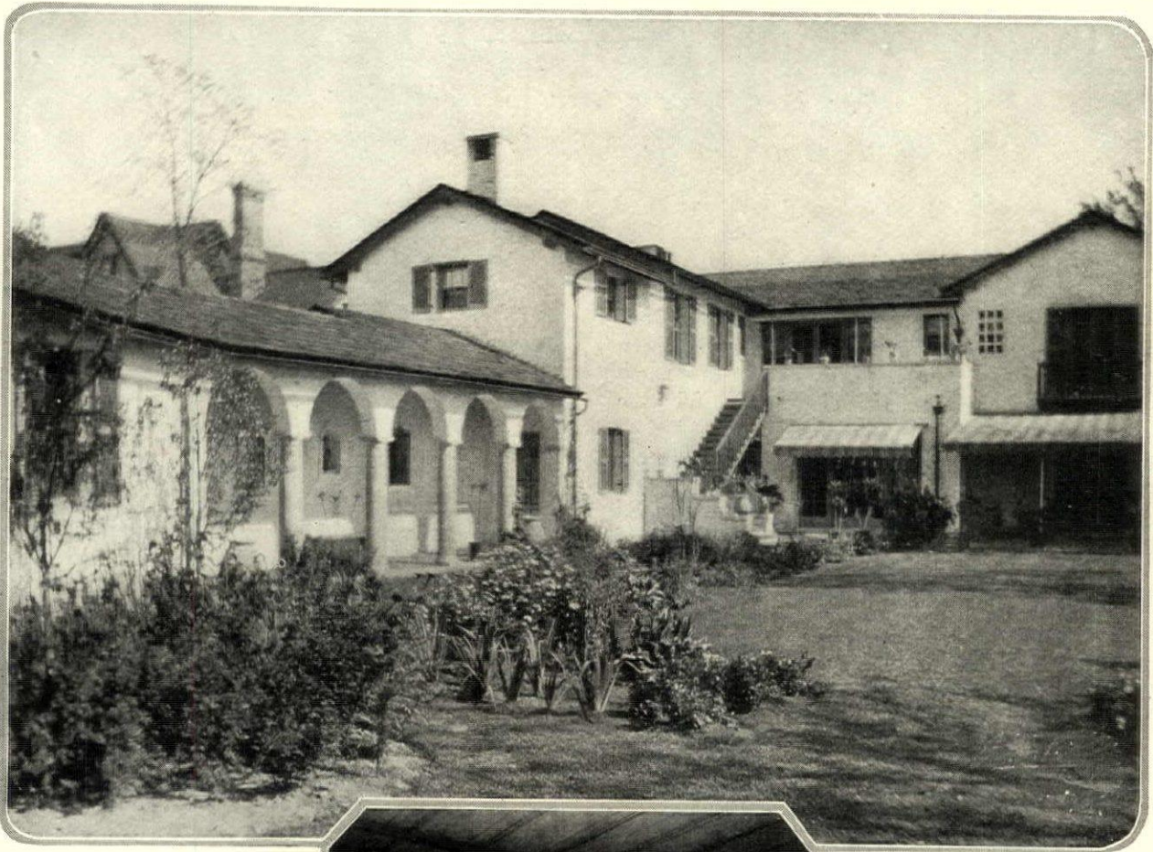
From the far end of the garden the interior angle of the house shows to best advantage, with its cloister-like passageway, its balcony up the outside stairs, and its shaded terrace
