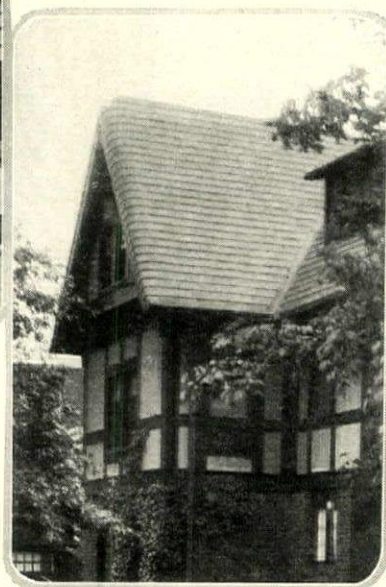
Here asbestos shingles, laid to form apparently hexagonal units, are being placed directly over an old wood shingle roof
