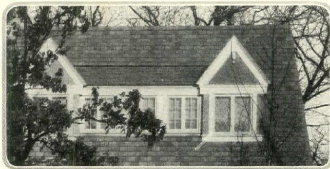
Asbestos shingles have developed in the direction of a beautiful range of colors. A roof of the type illustrated here naturally created the name "Colorblende"
