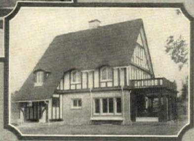
Residence of F. A. Pistorious, Rochester, N. Y. Architect—W. W. Ward, Liverpool, N. Y. Bishopric Stucco over Bishopric Base.
