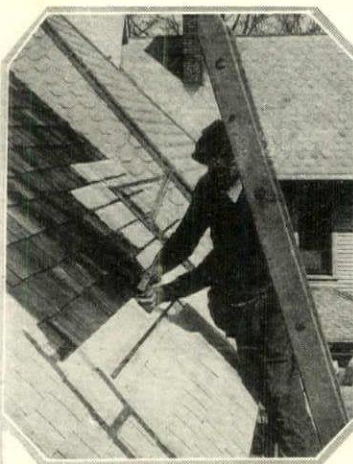
Laying "Flextone" asbestos shingles over an old roof, the roofer uses beveled strips of pine to make an even surface
