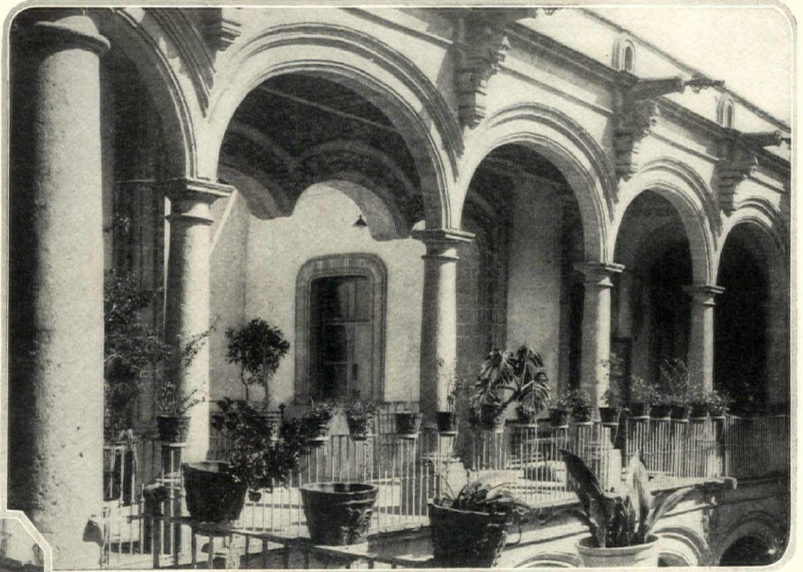
The upper cloister in the Conde de Santiago's house is remarkable for its splendid arches and its cannon gargoyles that are the insignia of those holding the rank of Capitan General
