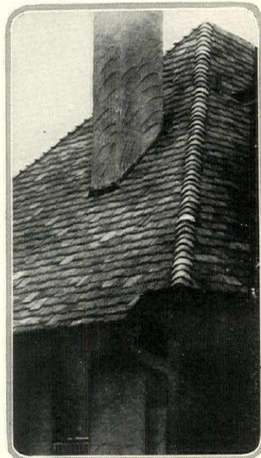
A roof of vigorously rugged character and texture is effected here by good use of “Mohawk Tapered Asbestos Shingles”
