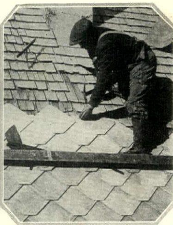
Here asbestos shingles, laid to form apparently hexagonal units, are being placed directly over an old wood shingle roof
