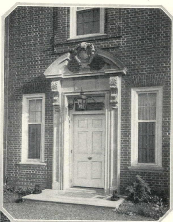
The main, or north entrance is pronounced by a carved cartouche in the broken pediment, a lantern, and a moulded brick panel above. The roofs and the flashings of this house are of lead
