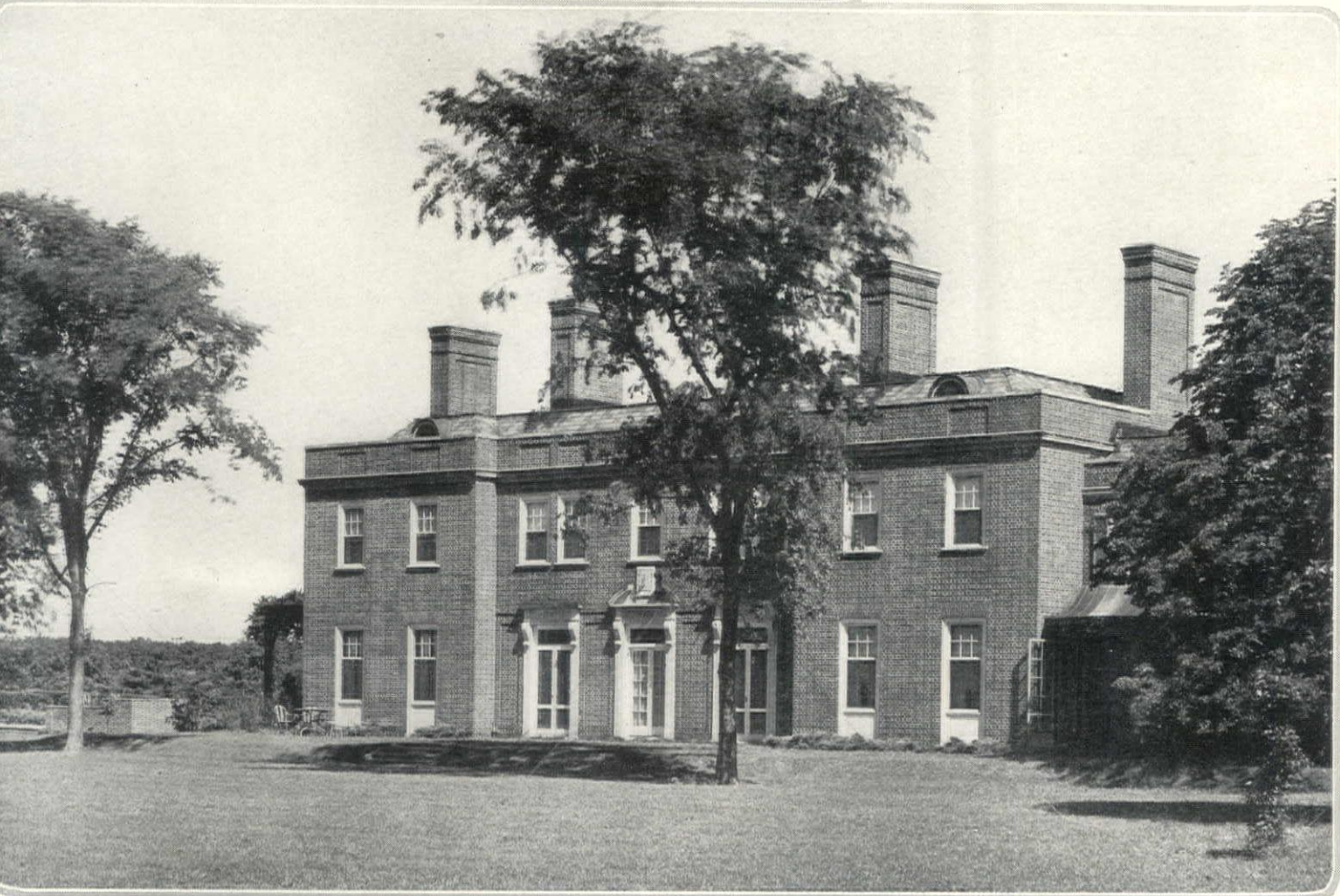
The south side faces one of the stretches of lawn that surround the house. Huge Elms have been moved in to give immediate shade and beauty to the grounds. The landscaping was designed by Olmstead Brothers
