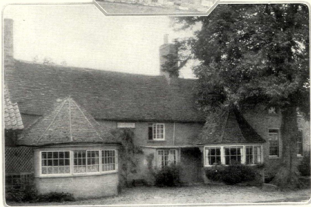
A pair of one-story bay windows on a little tavern in Northamptonshire. These bay windows are exceedingly simple in conception and are capable of turning the entire end of a room into a sun parlor
