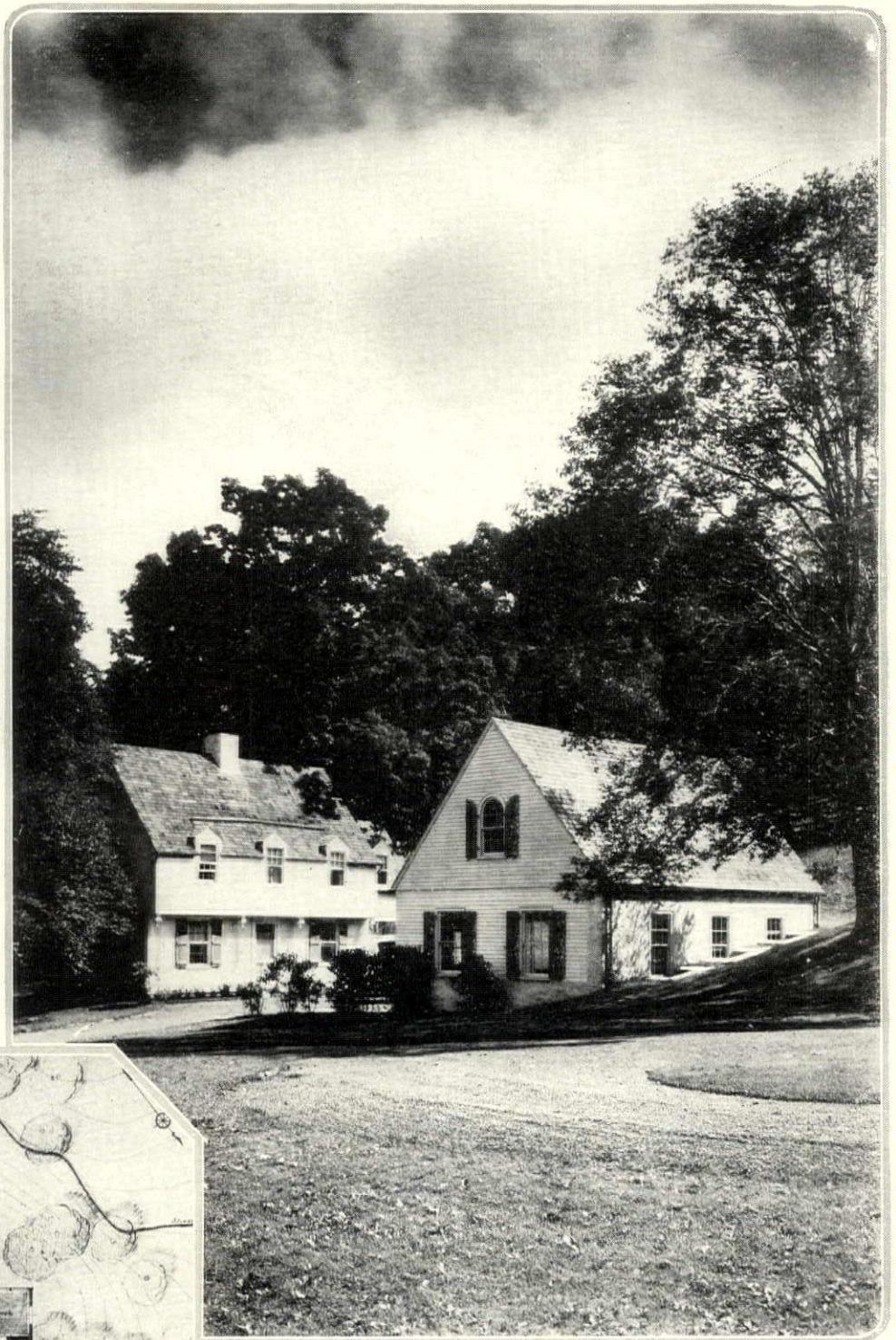
A three-car garage is in the foreground and the chauffeur's cottage is just across the road. The latter with its overhanging second story is a reproduction of some of the early New England Colonial types. Tilden, Register & Pepper were the architects
