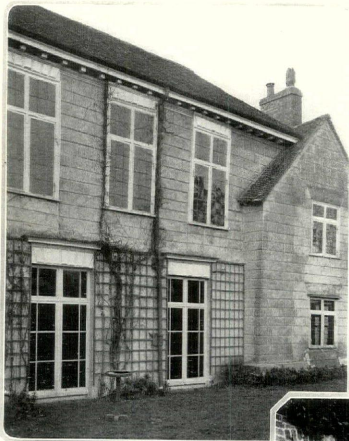
The late 17th Century windows on Harlington Manor, Bedfordshire, mark the gradual transition from the Tudor to the Classic style of architecture in England
