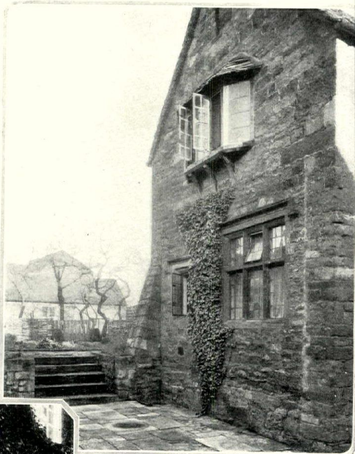
Windows at the back of the Spencer cottage, Broadway, Worcestershire. The upper one is a form of shallow bay and has leaded casements and wood mullions
