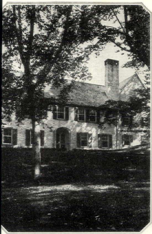
A part of the south side of the home of Charles E. Brinley at Chestnut Hill, Penn., is shown above. The exterior of the house is finished in rough stone painted with a thin mixture of white cement and lime
