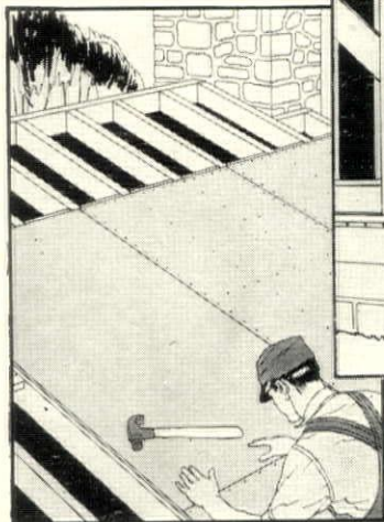
Most heat beats through roofs in summer, causing hot attics. Most heat leaks out through roofs in winter, causing high fuel bills. Celotex applied over or under roof rafters gives the needed protection. Both uses are recommended.
