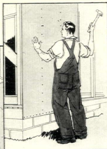
As sheathing, Celotex supplies the insulation needed back of brick, wood or stucco exteriors. Here, it replaces the rough boards formerly used, gives greater strength to the house walls and makes building paper unnecessary.
