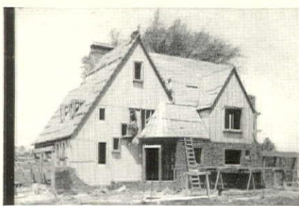
Celotex Sheathing insulates the house, adds to structural strength and is easy and inexpensive to apply.
