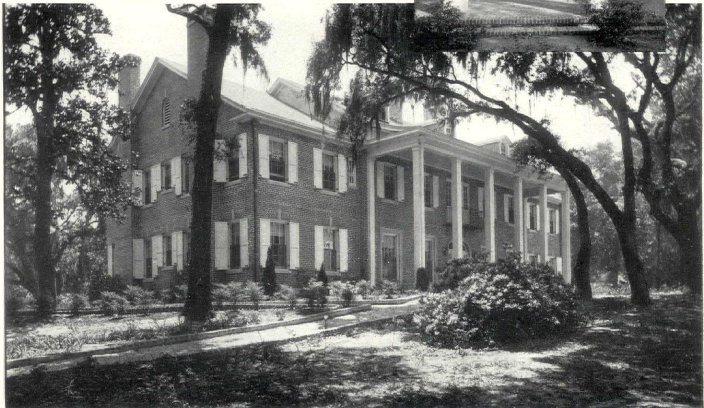
FRONT FAÇADE WITH TWO-STORY PORCH
