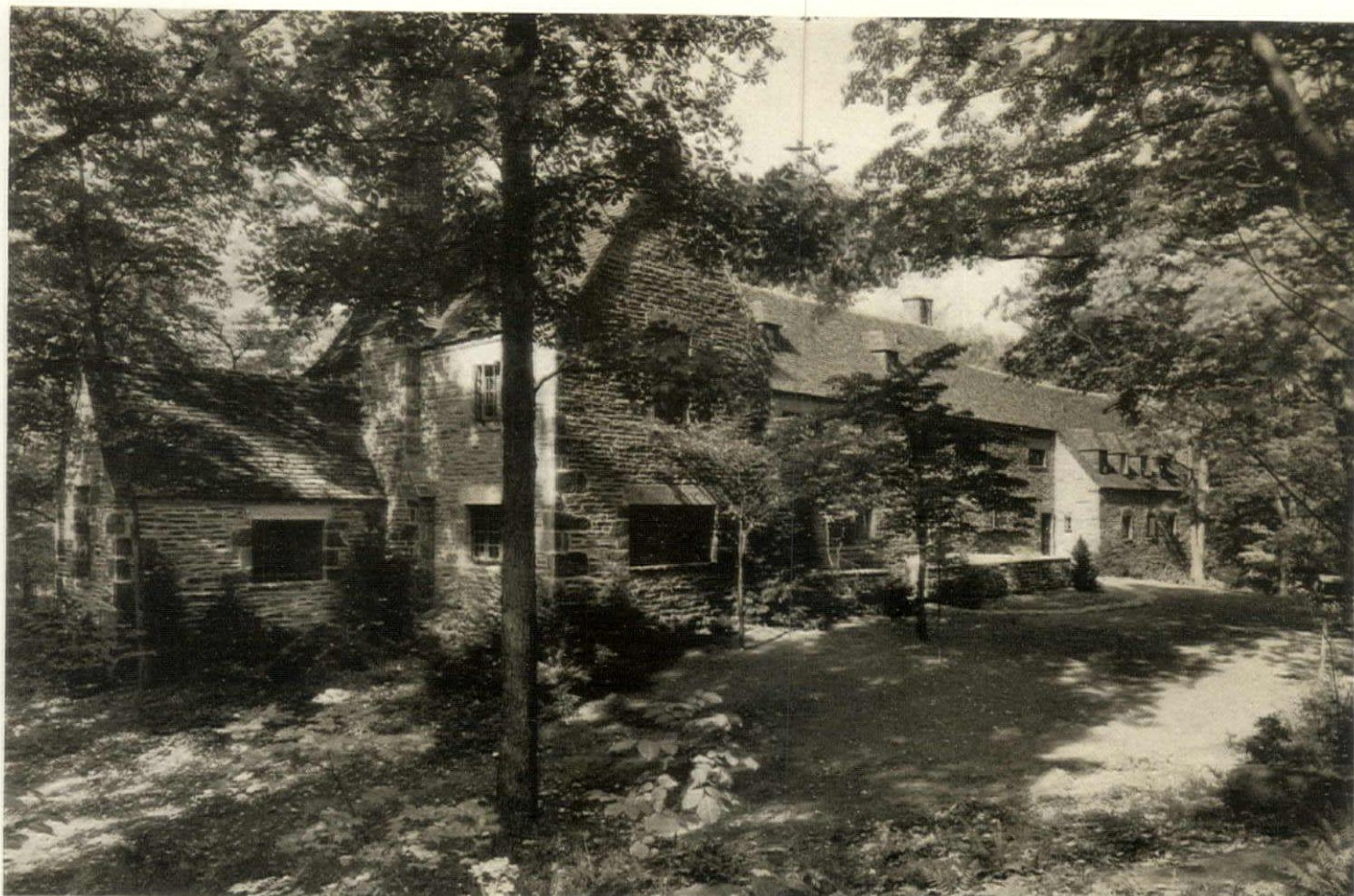
GENERAL VIEW OF REAR FAÇADE
