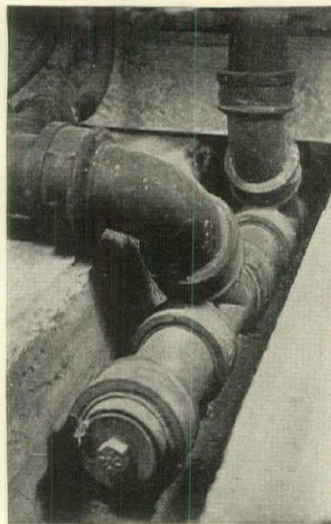
Should this waste pipe become clogged, the conveniently located clean-out will facilitate a speedy remedy. Every important bend should have a clean-out
