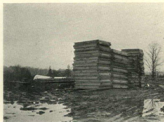
Exposed to the weather, these window frames will become saturated, then warp and shrink after installation. Millwork should be protected at all times
