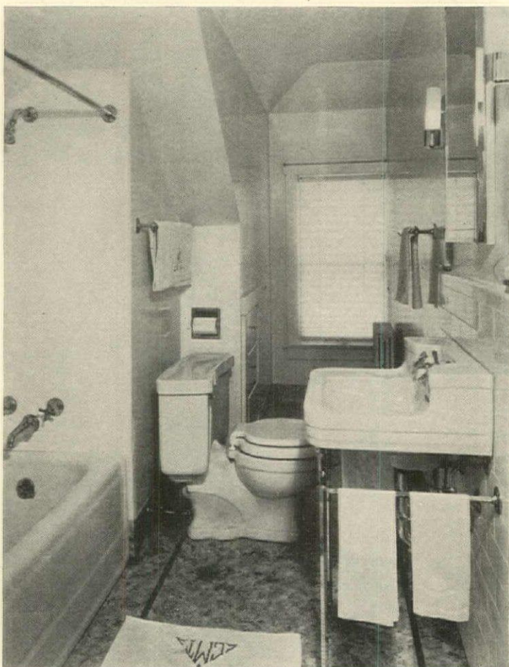
A good example of a complete bath, added during remodeling, in an attic space which had size and head-room problems. Crane Co.
