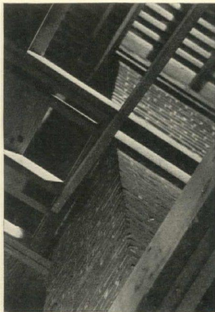
The chimney stands free of the structure. Wood and masonry never settle or shrink equally and if tied together can cause serious distortion
