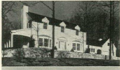
DOUBLE-WHITE house in New Canaan, Conn. Gloss Collopake trim. Robert C. Kilborn, Architect.
