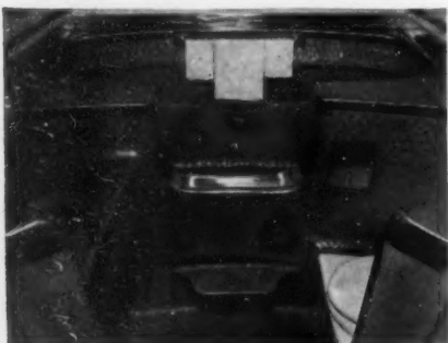
An experimental bathroom designed as a single unit, by Buckminster Fuller, foreshadows postwar developments.
