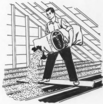
Attics with no floors can be very effectively insulated by laying moisture-proof paper between the joists, pouring in insulation to the thickness of the joist.
