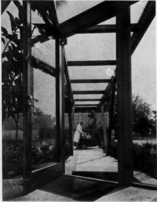
Daringly cantilevered on cypress posts, a wired glass canopy protects the entrance path. At the far end Mrs. Wallace loads the auto-scooter.
