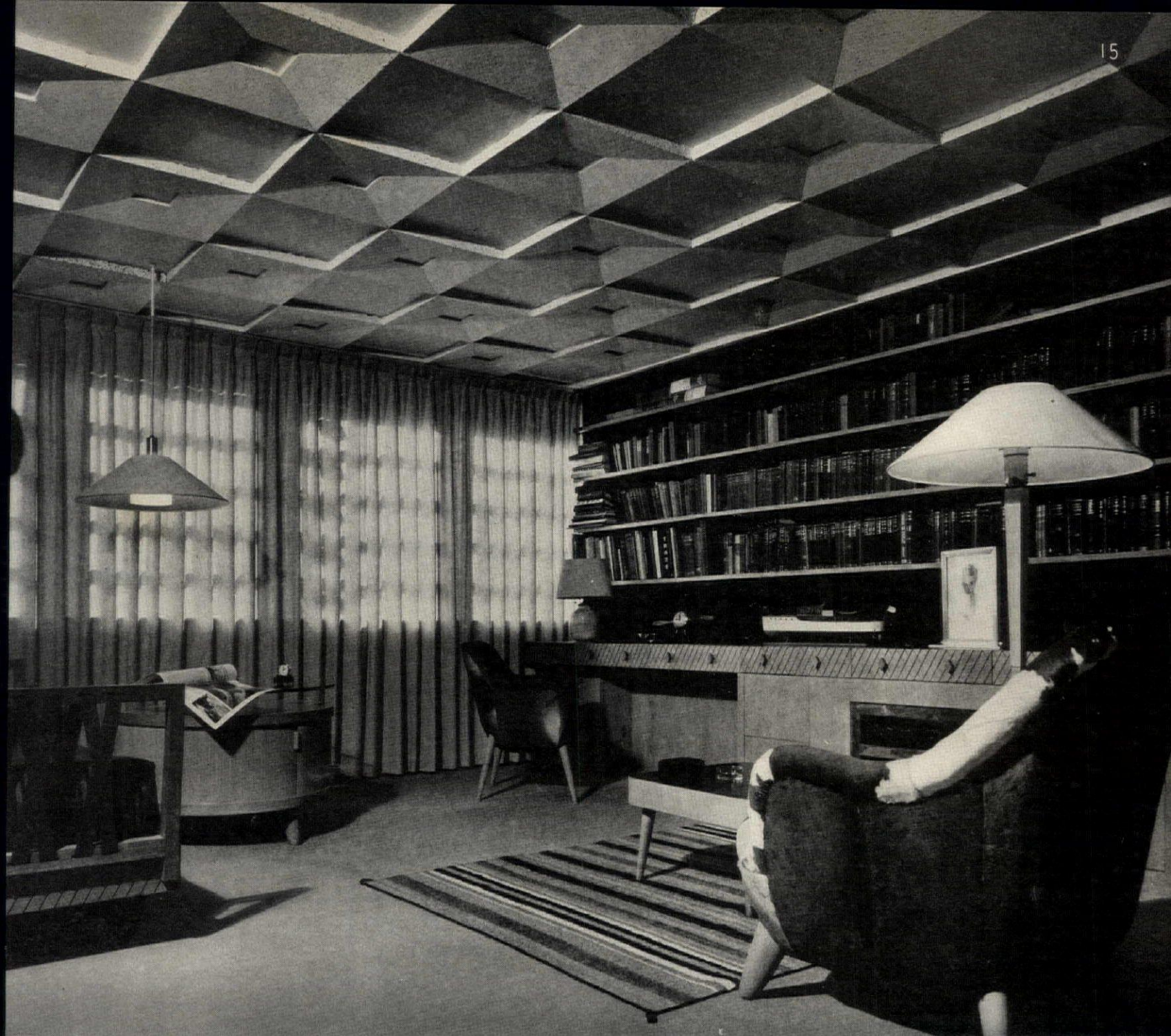
MR. FAIRCHILD'S BEDROOM IS HUSHED BY A COFFERED CEILING OF CORK
