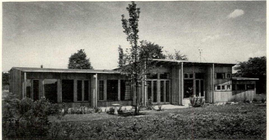
The south façade. Uprights bar the entry of the western sun.
