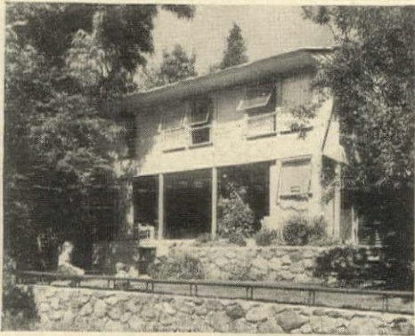
LIVING-DINING AREA HAS GLASS WALL
