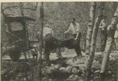
CLEARING THE ROADWAY
