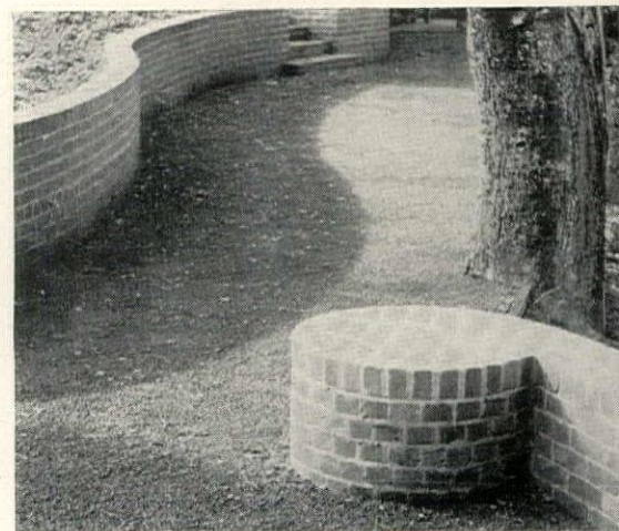
SERPENTINE BRICK WALLS recall Jefferson. They harmonize with the natural landscaping.
