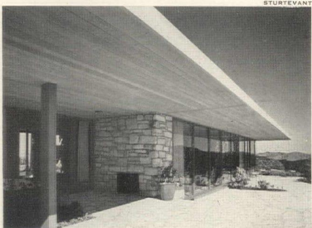
TERRACE borders the hill to the south and west, a step away from the living room through sliding glass doors. Terrace is reached from the patio by the entrance hall, left. The woodbox adjacent to the living room fireplace may be filled from outside through the small opening at the base of the chimney wall.
