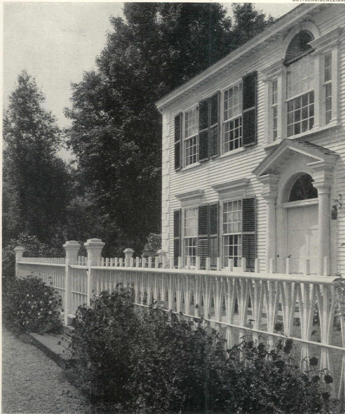
WHITE-PAINTED FENCES of the post-revolutionary Colonial period were in the spirit of the architecture of the houses. The native white pine, whose strips could be easily bent into a pattern, gave early designers a versatile medium.
