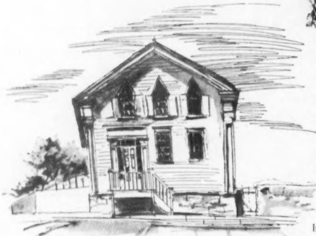
HIGH STOOP AND POINTED WINDOWS ON PINE STREET
