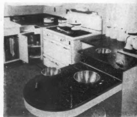
4. CARROUSEL CUPBOARDS for pots and pans flank the range. They solve the age-old problem of waste space at the back of storage units. Note low work counter.
