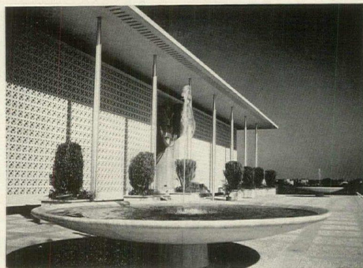
Huge saucers on low pedestals catch the flow from fountains on the terrace of the U. S. Chancellery in New Delhi, designed by Edward Durrell Stone. Outer shell of grillwork conceals the fact that the building is two stories high.
