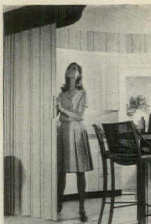
Sliding tambour doors pull easily on their serpentine track to separate the kitchen's two parts.
