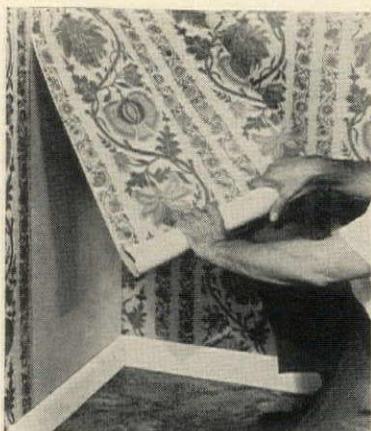
Moving day: paper is gently peeled from wall, rolled up from baseboard.
