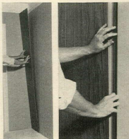
Step 4. You line up panel at starting line and press into place. Next to it, snap in the joint molding, which has a groove to fit panel-tongue. Repeat the process ad finis .
