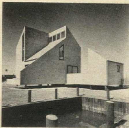
Nine piles support the house, keep it high and dry in hurricane weather.
