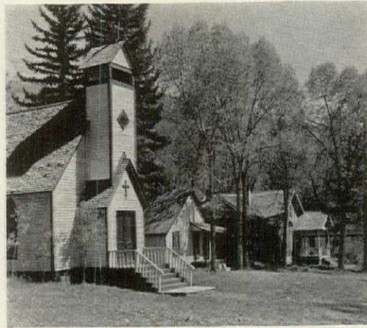
A frame church and an orderly row of cottages once sheltered quarry workers' families at Marble, southwest of Aspen. Mines in area produced silver, lead, and zinc; marble from quarries was used in Lincoln Memorial, Tomb of Unknown Soldier.
