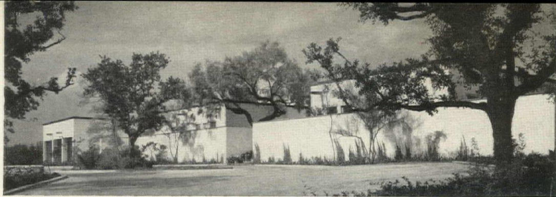
Like an oasis, circling walls ring the masonry house for maximal privacy.
