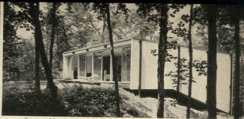
Supported by steel posts, the house is angled to fit the contour of the site
