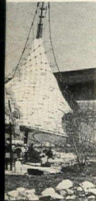
Small extension of Germany's big top is same superb windswept shape held taut by steel mesh.
