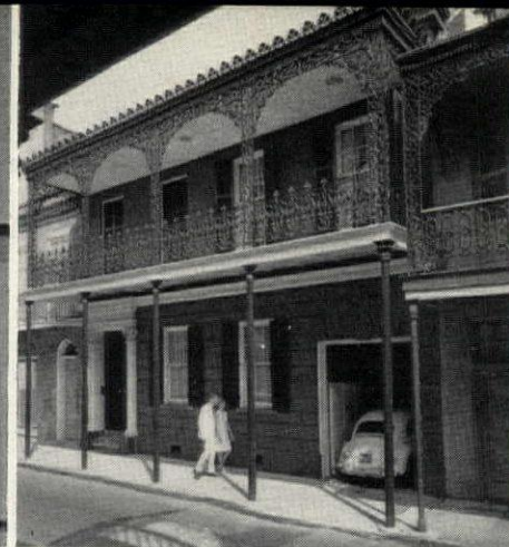
Front door is at left of façade, old carriage way at right.
