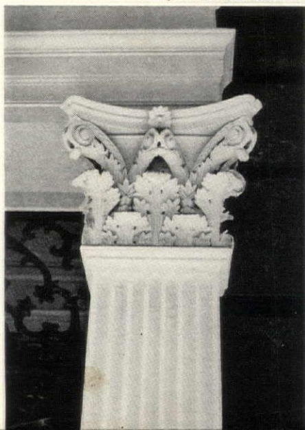
Columns and cornice of front door are characteristic of Gallier's work.
