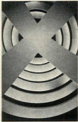
Domed ceiling of graduated white wood bands could be adapted to crown foyer.
