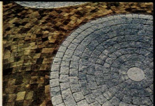
Wood and stone blocks alternately pave a terrace—wood on flat parts, stone for saucer-shaped fountains.
