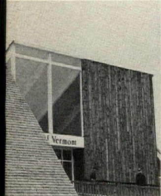
Wood in two forms—shingles and sheathing—are effectively juxtaposed on staggered halves of an A-frame.
