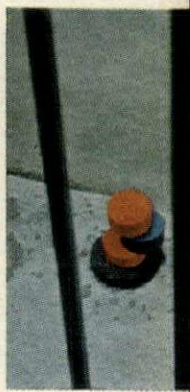
Wood disks piled into a bollard conceal a shore light.
