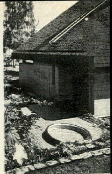
This page The house seen from the garden and paved courtyard. Section and floor plans are shown at left, with ground-floor plan at the foot of the column
