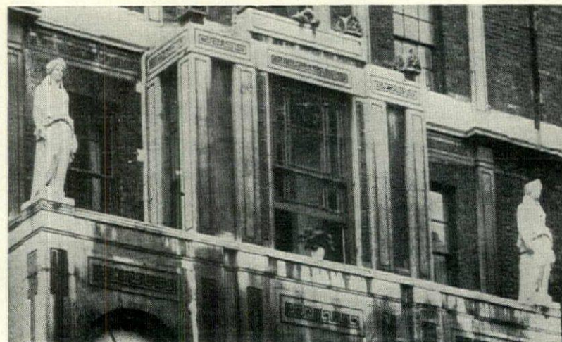
Coade figures on the façade of the Soane Museum, Lincoln's Inn Fields, formerly the home of Sir John Soane
