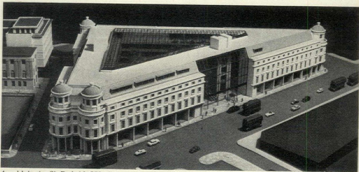
A model showing Sir Frederick Gibberd's proposals for Coutts Bank with 'a top-lit open-plan banking hall' as a centre-piece
